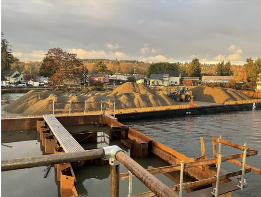
Barge of clean sand used to cover the dredged areas in SMA 14A, 14C, and 14D. (Geosyntec, November 24, 2025)
