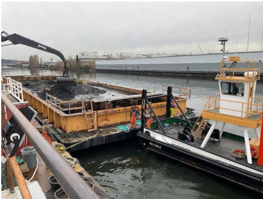
Barge of contaminated sediment from SMA 15A as the construction team nears the completion of required dredging. (Geosyntec, November 25, 2025)
