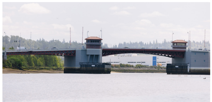
PHOTO CREDIT: KING COUNTY WASTEWATER TREATMENT DIVISION
