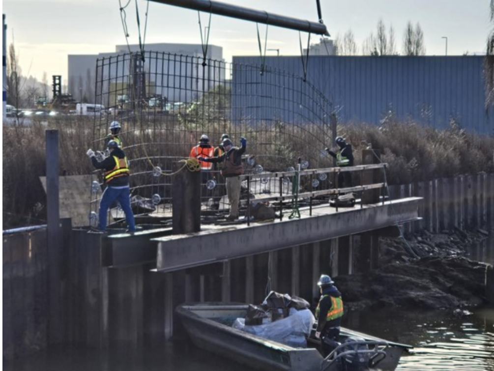
Preparing for the finishing work of SMA 9 bulkhead wall system (sheet pile wall) with the installation of concrete reinforcing rebar (Geosyntec Consultants, week of February 24, 2025).
