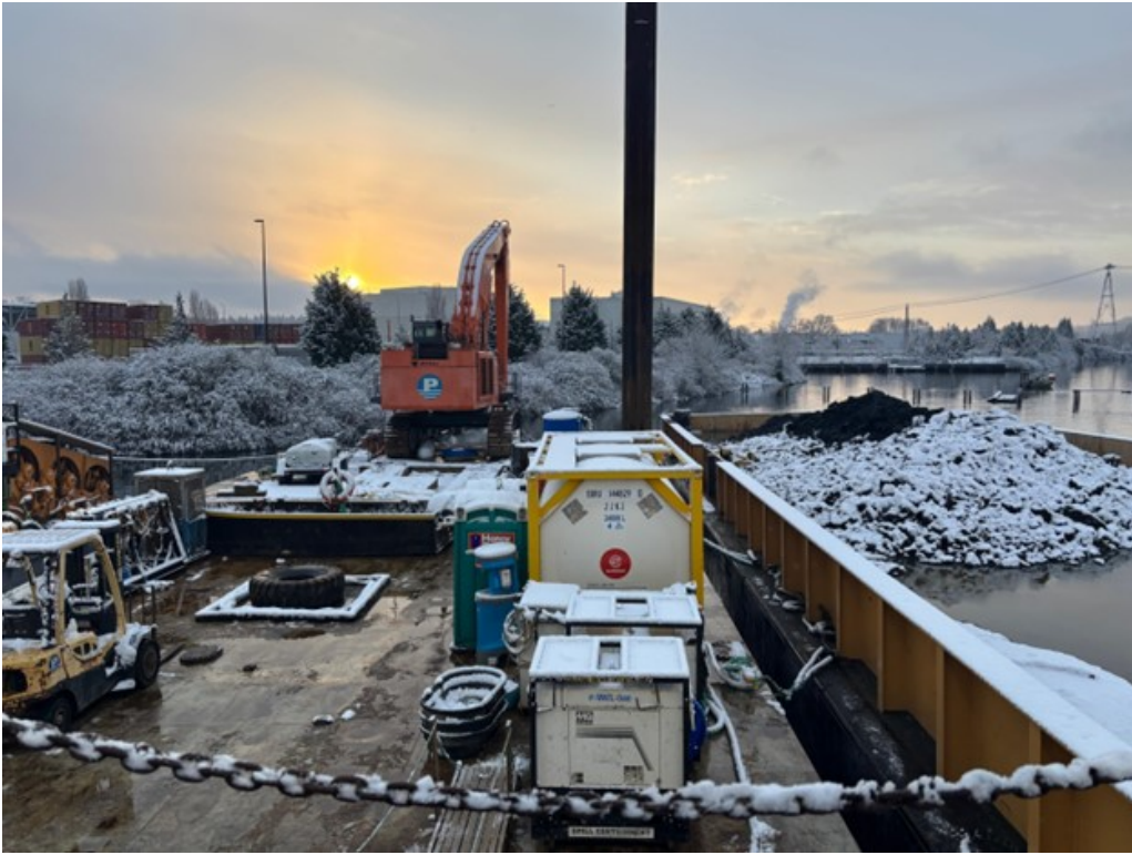
Backfilling must be done during high tides which may require working before sunrise or in snowy conditions (Photo credit: Geosyntec, week of February 3, 2025).
