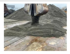
Example of the sandy material used for Enhanced Natural Recovery to be placed at SMA 8, 11, and c1.
