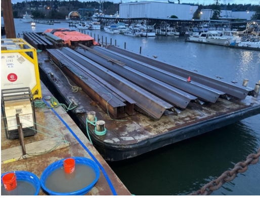
Sheetpiling materials ready to be installed at SMA 9. (Photo credit: Geosyntec)
