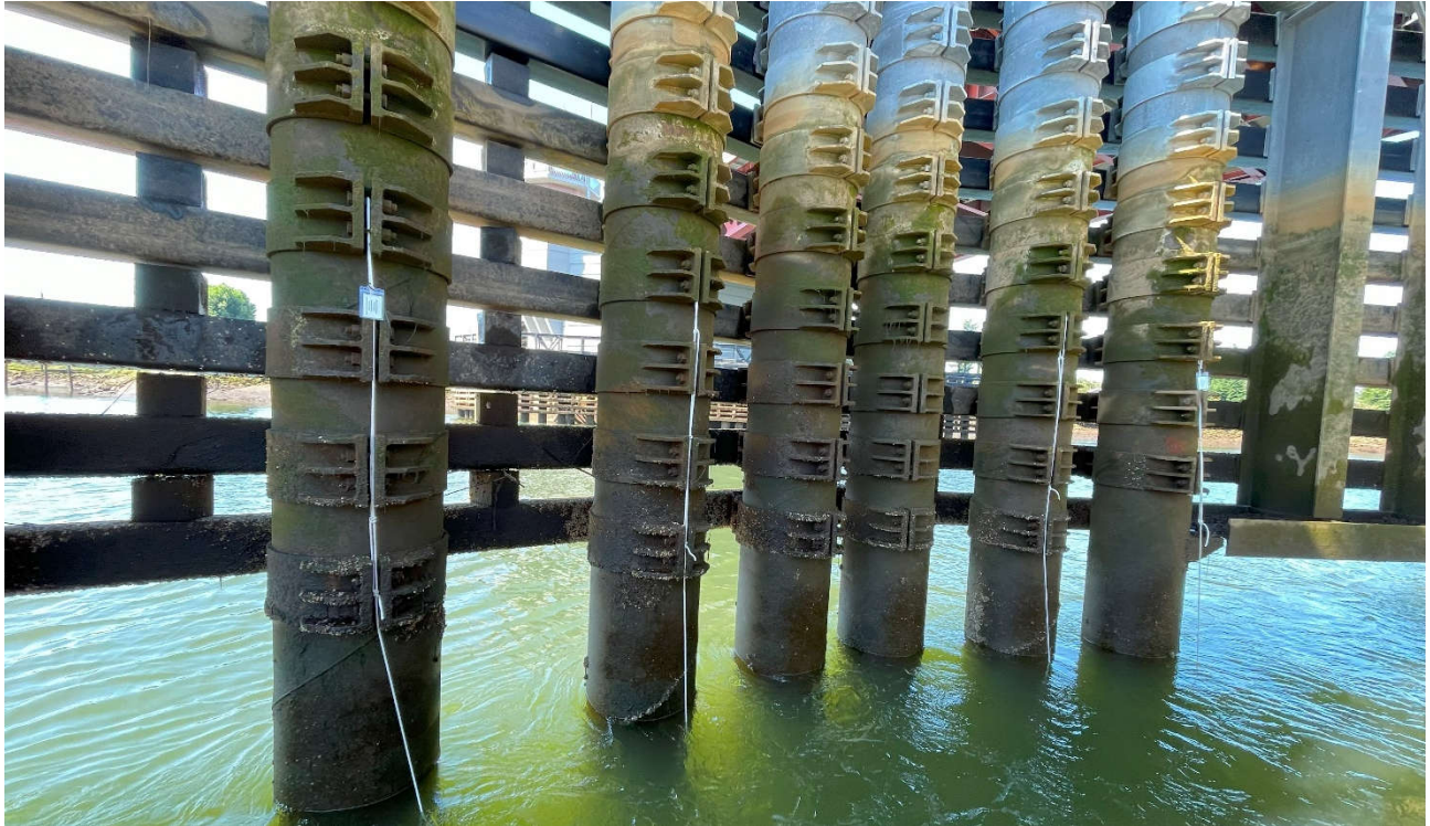
Figure 13. Passive sampler deployment location PS1 at RM 3.3E (South Park Bridge)
