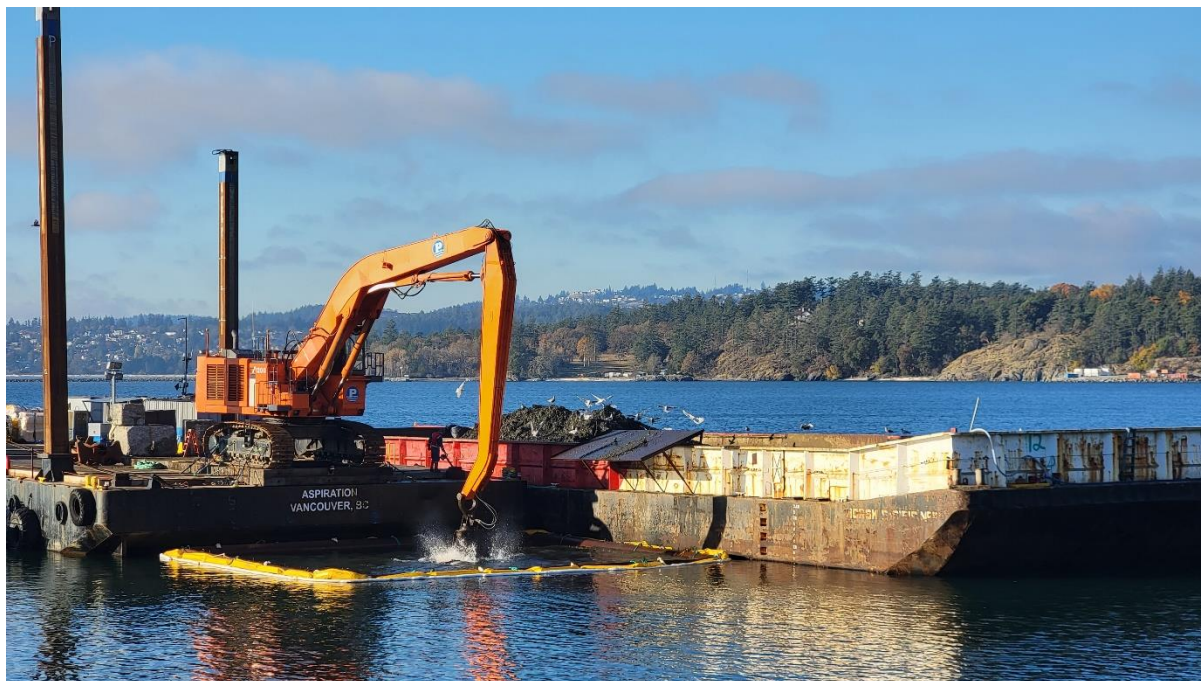
Figure 1: Typical Moonpool Configuration
