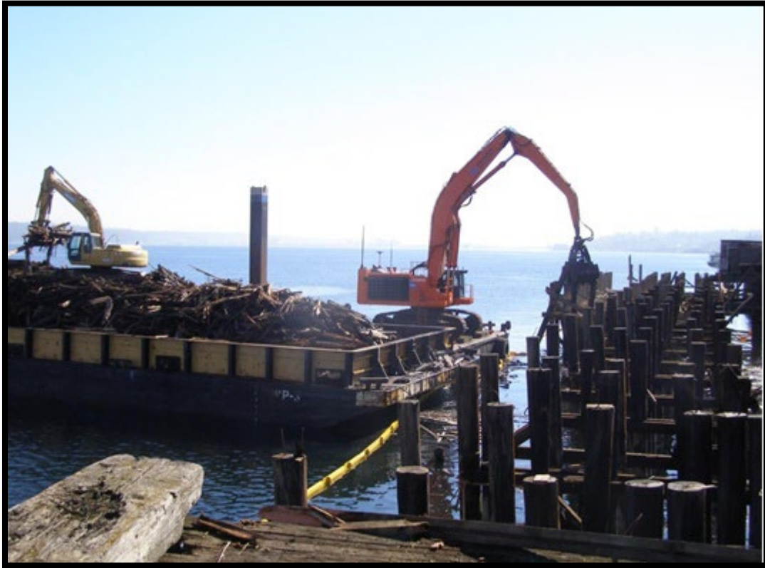
Figure 1- Pile Extraction w/ Clamshell Bucket
