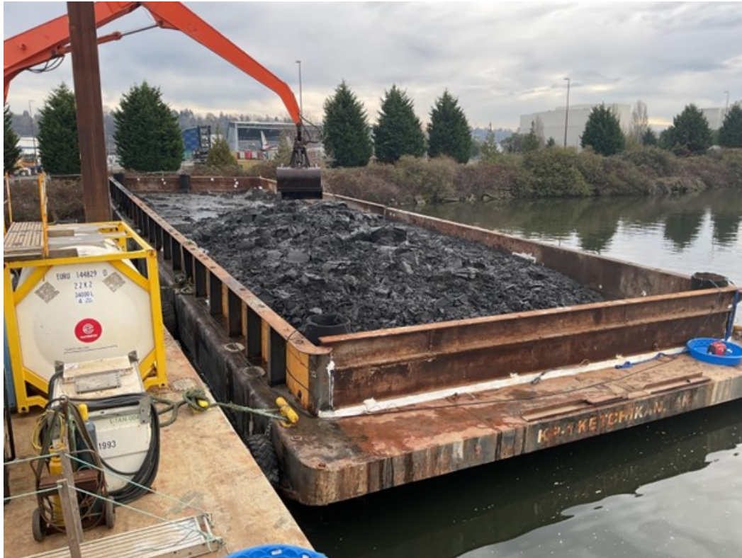
A barge holds excavated sediment from SMA 6. (Photo credit: Geosyntec)
