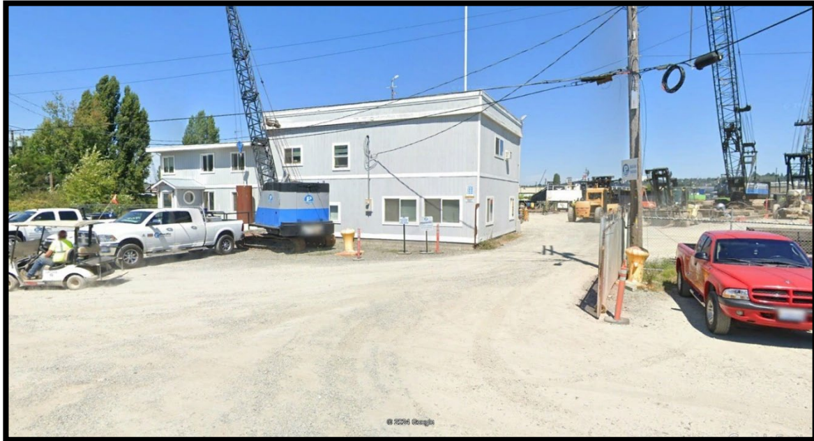
Figure 4. PPM's Permanent Offices front gate.
