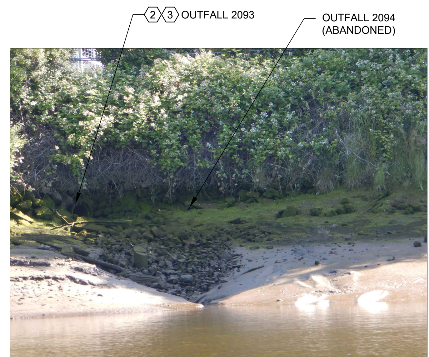
OUTFALLS PHOTO 1 SCALE: NONE
