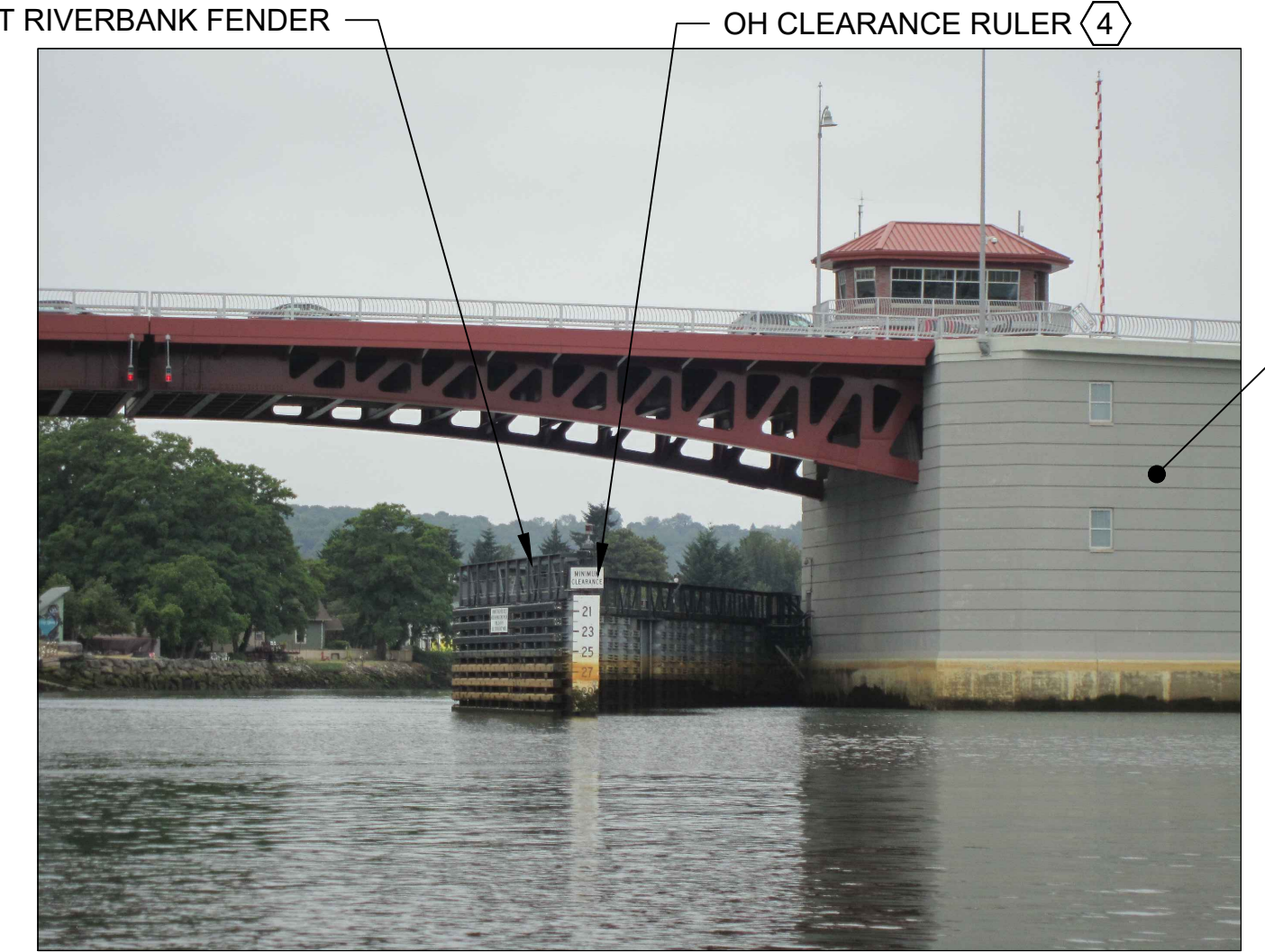
FENDER (LOOKING DOWNSTREAM)
