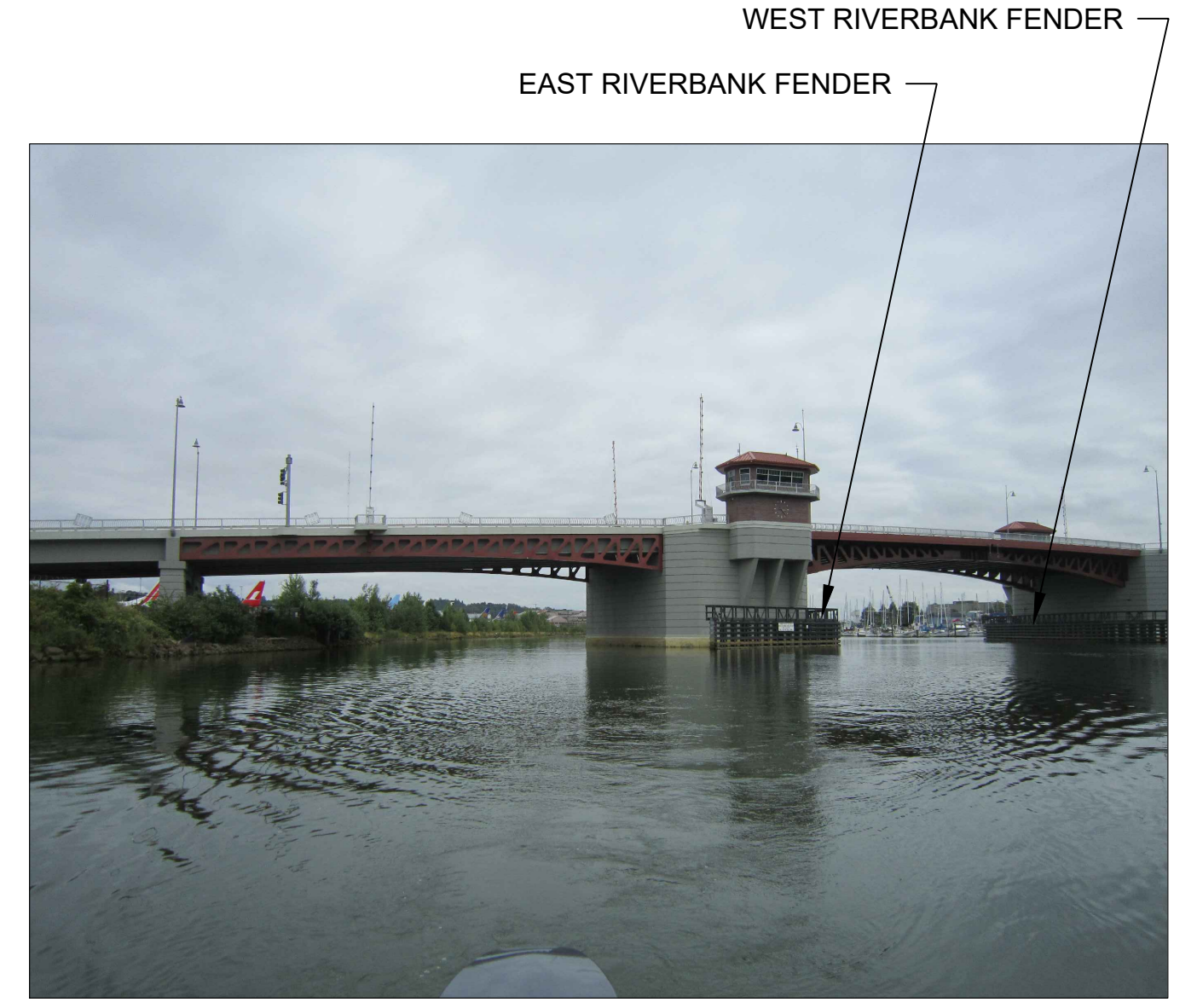
FENDERS (LOOKING UPSTREAM)
