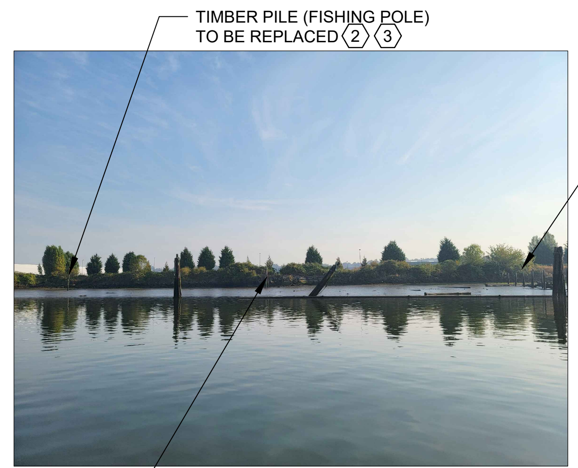
TIMBER PILE PHOTO SCALE: NONE
