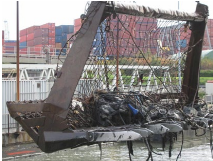
Exhibit 11-1 Debris Removal Prior to Dredging
