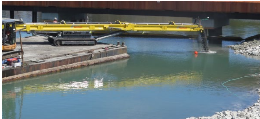
Variable-speed telebelt placement
