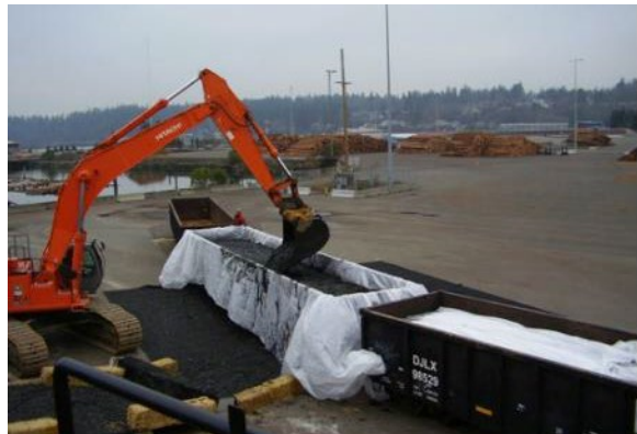
Loading of sediment into lined containers
