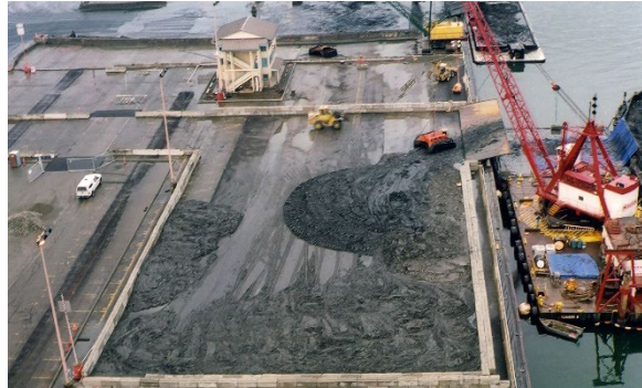
Contained landside facility
