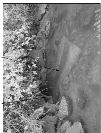
OUTFALL 2093 PHOTO SCALE: NONE
