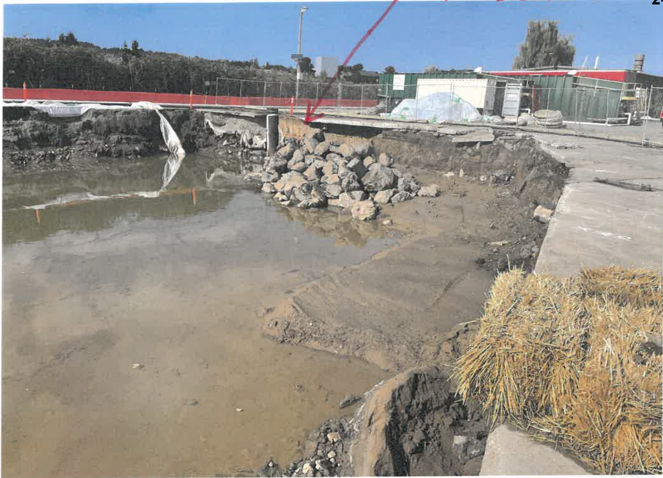
Wall 1 Sheet Pile
