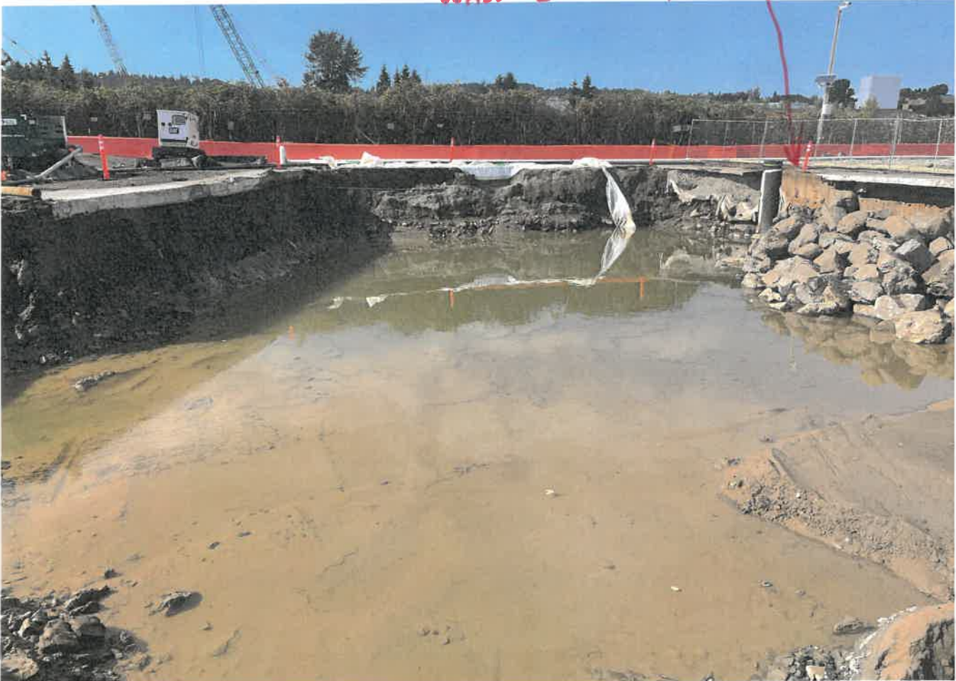
Wall 1 - Looking West
