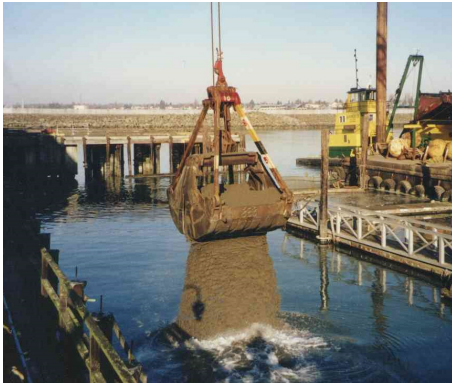
Controlled bucket placement
