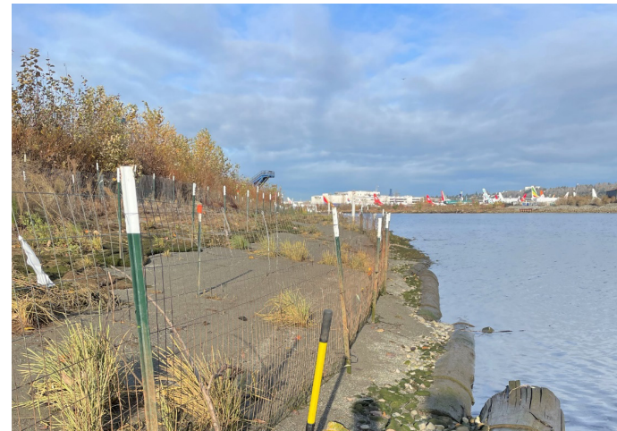
Photograph D: Phase III, West Bank
