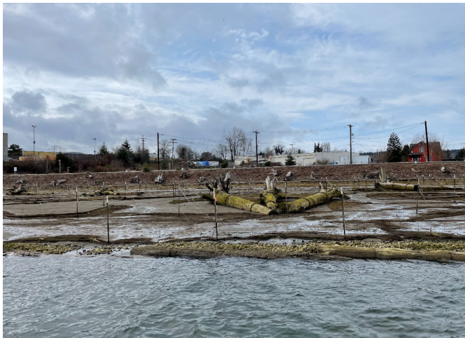
Photograph C: Phase III, East Bank
