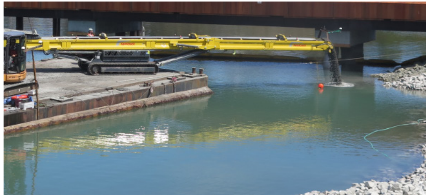
Variable-speed telebelt placement
