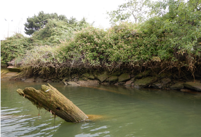
Photograph A: Phase II, East Bank
