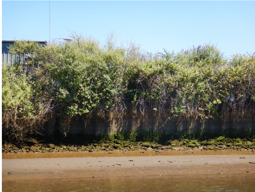
Photograph A: Phase I, East Bank
