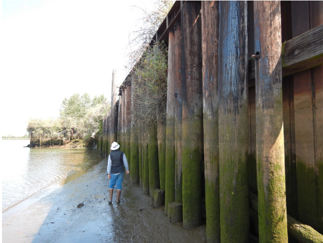
Photograph A: Phase II, East Bank
