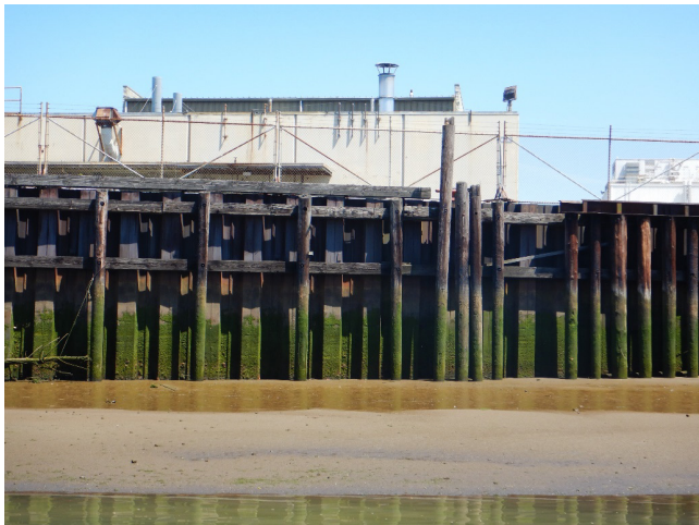
Photograph C: Phase I, East Bank
