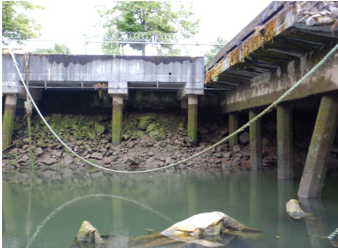
Photograph A: Phase I, East Bank
