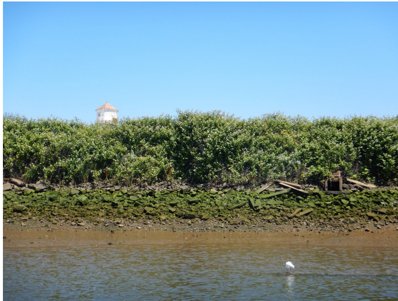
Photograph A: Phase I, East Bank
