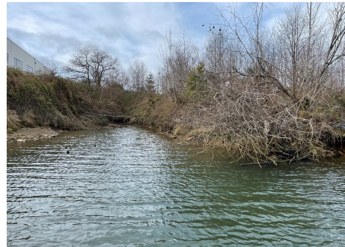
Photograph D: Phase III, West Bank
