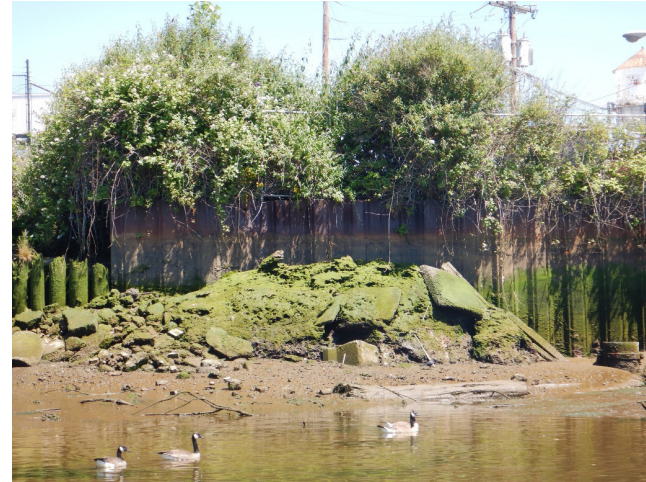
Photograph B: Phase I, East Bank
