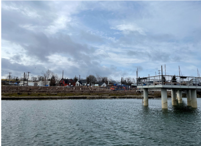
Photograph A: Phase III, East Bank
