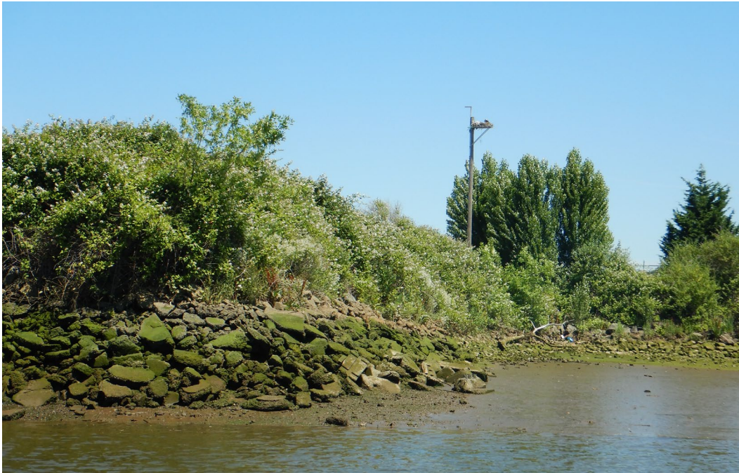
Photograph C.1.4-1 Bank Conditions at the Northern End of SMA 5, Looking East
