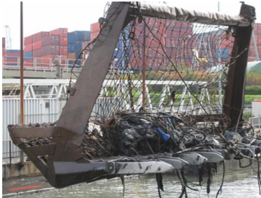
Exhibit 11-1 Debris Removal Prior to Dredging
