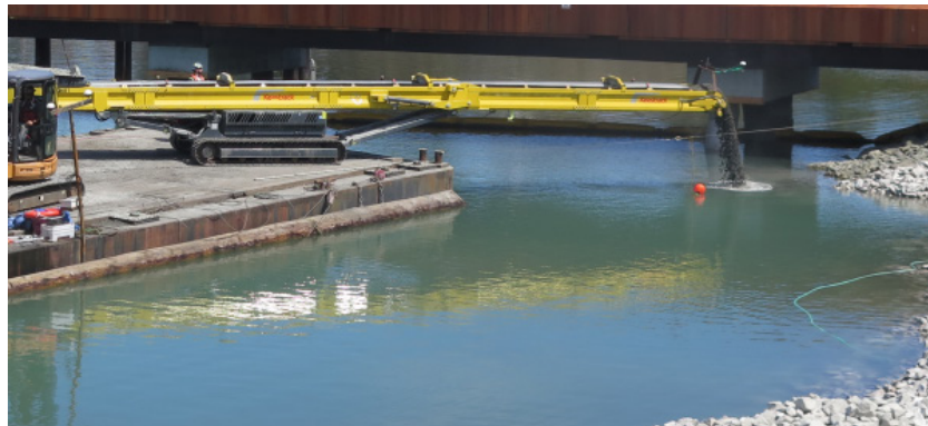
Variable-speed telebelt placement
