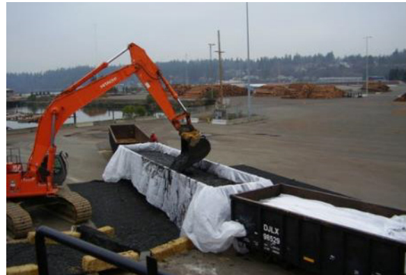
Loading of sediment into lined containers
