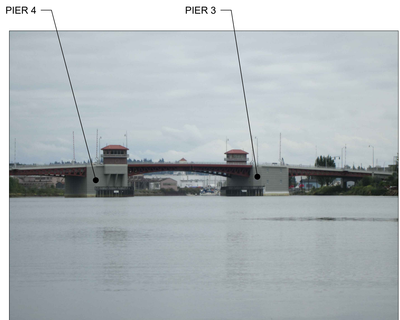
BASCULE BRIDGE (LOOKING UPSTREAM)
