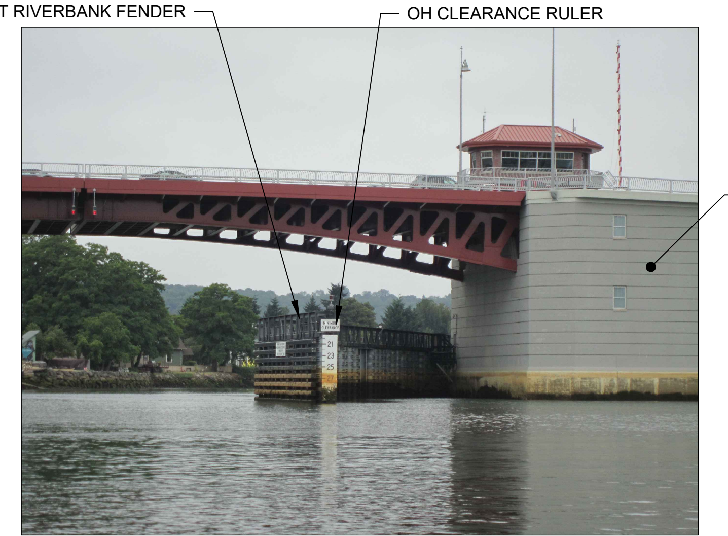
FENDER (LOOKING DOWNSTREAM)
