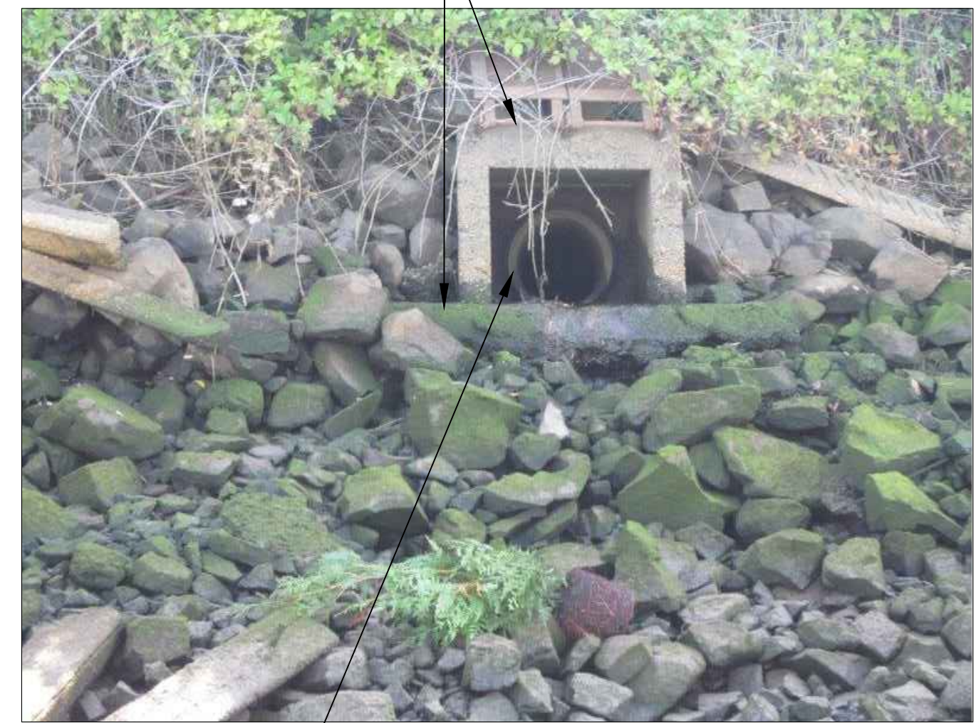
OUTFALL 2073 SCALE: NONE 5 OUTFALL 2073 18" DIA CONCRETE PIPE. IF OUTFALL IS WITHIN DREDGE PRISM, REMOVE EXISTING RIPRAP AS REQUIRED
