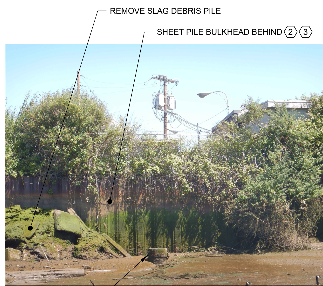
OUTFALL 2075 SCALE: NONE 4 OUTFALL 2075 32" DIA STEEL RISER 5 REMOVE SLAG DEBRIS PILE SHEET PILE BULKHEAD BEHIND 2, 3
