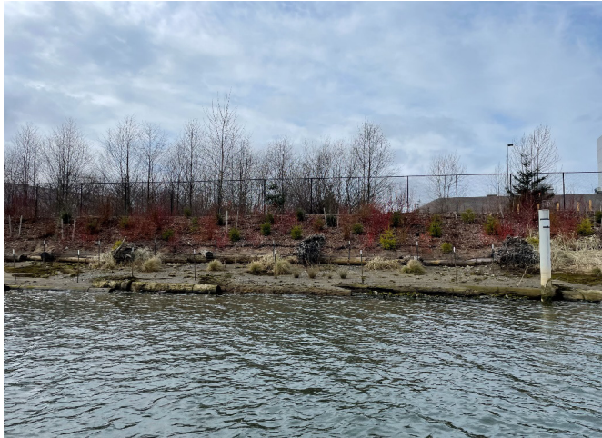
Photograph A: Phase III, West Bank
