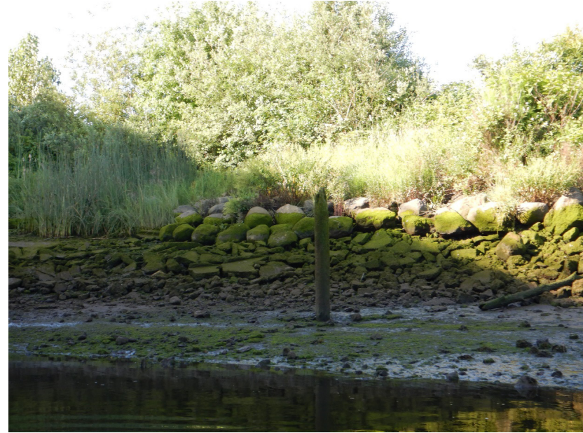
Photograph B: Phase I, West Bank
