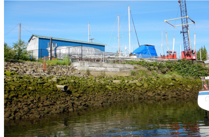
Photograph B: Phase I, West Bank
