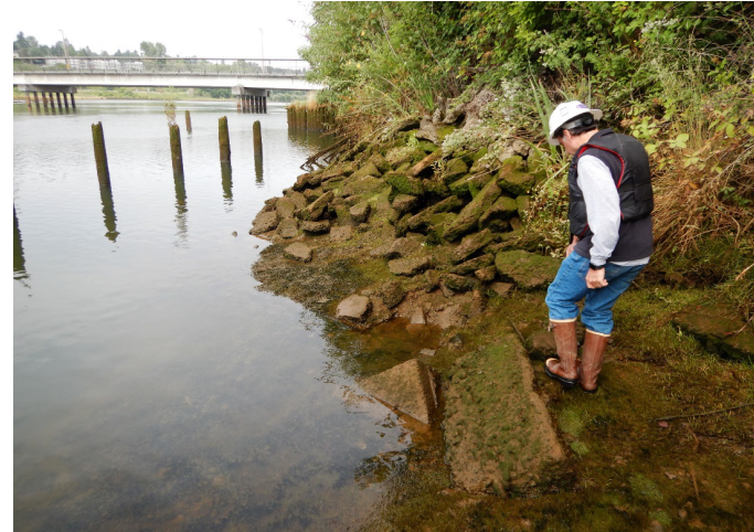
Photograph B: Phase II, East Bank
