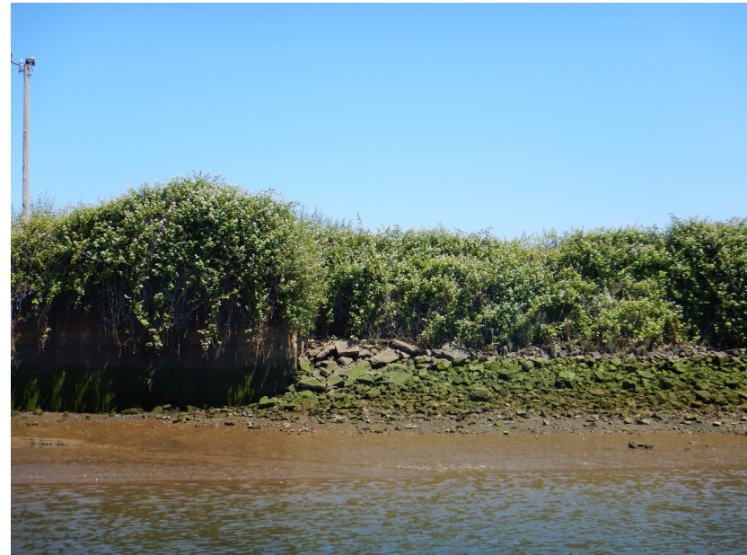
Photograph B: Phase I, East Bank
