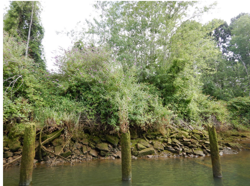
Photograph B: Phase II, East Bank
