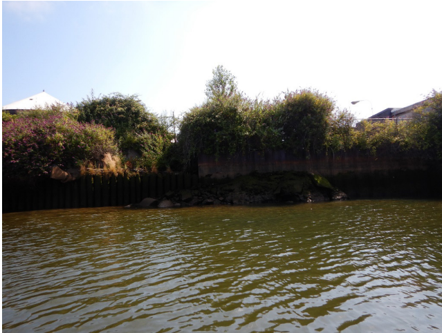
Photograph A: Phase II, East Bank
