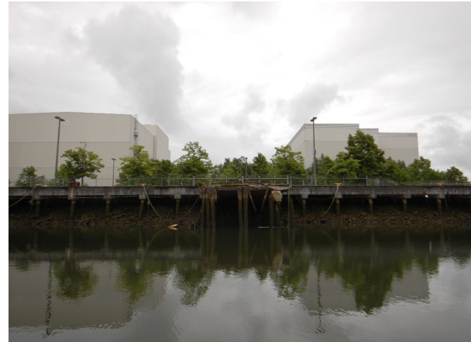
Photograph B: Phase I, East Bank
