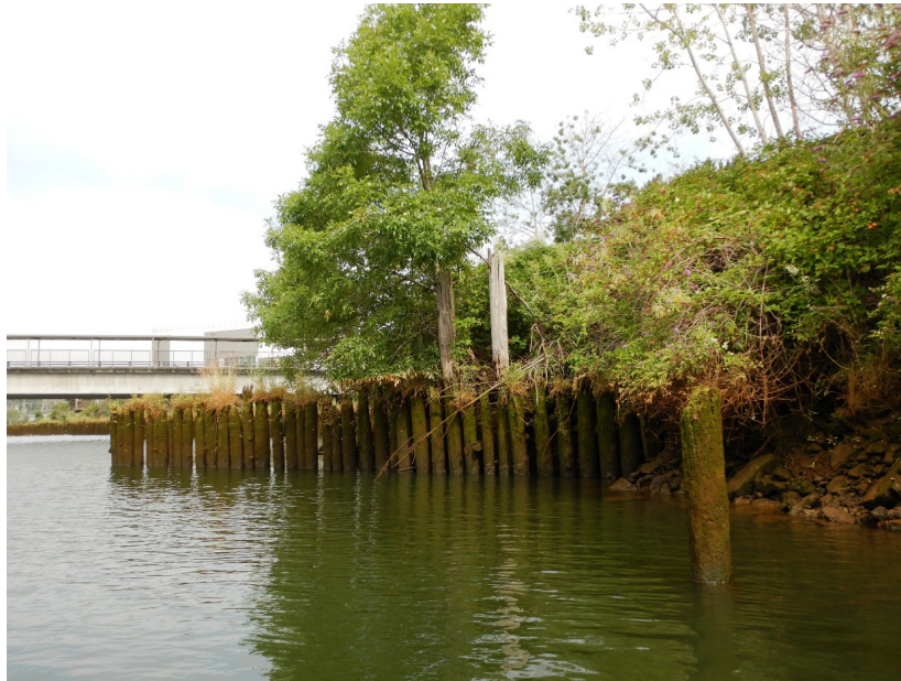
Photograph A: Phase II, East Bank
