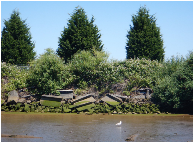
Photograph C: Phase I, East Bank
