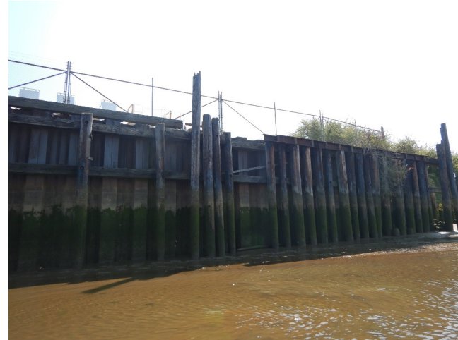
Photograph B: Phase II, East Bank
