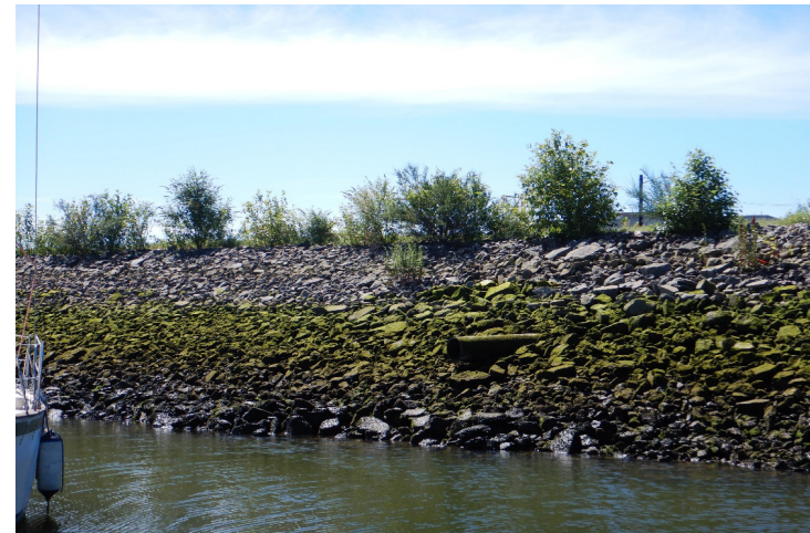
Photograph D: Phase I, West Bank
