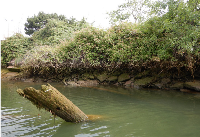
Photograph A: Phase II, East Bank
