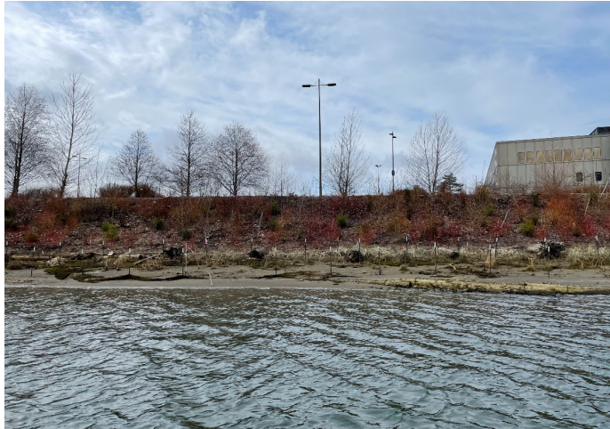
Photograph A: Phase III, West Bank
