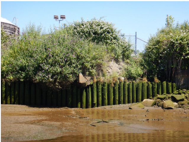
Photograph C: Phase I, East Bank
