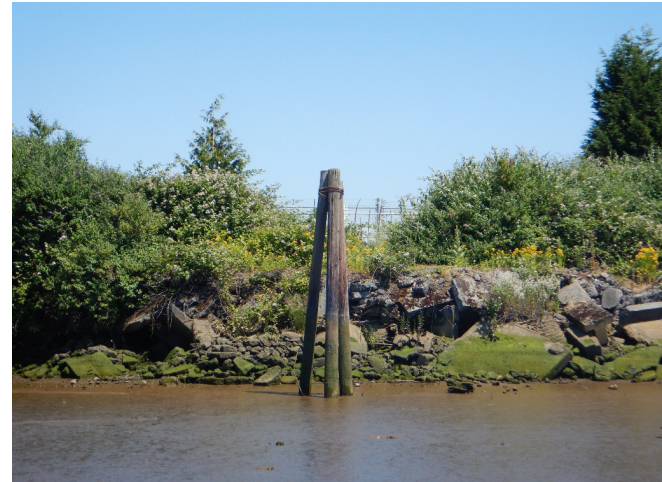
Photograph B: Phase I, East Bank
