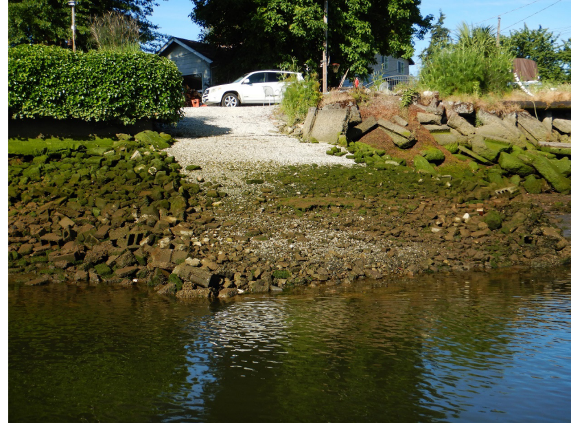
Photograph B: Phase I, West Bank
