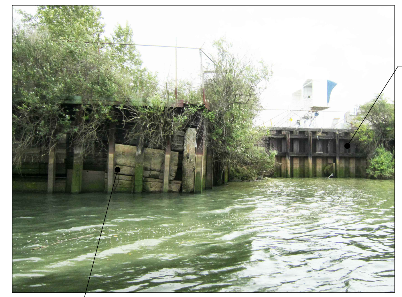
STEEL H-PILES WITH STEEL AND CONCRETE PANEL RUBBLE LAGGING
