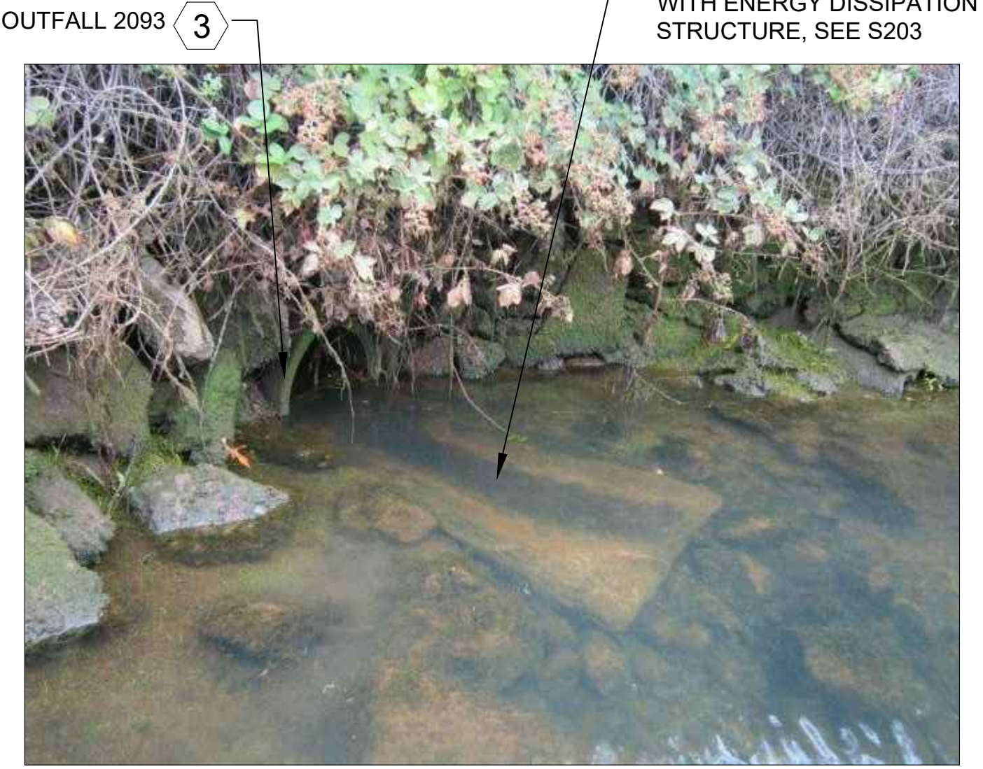
OUTFALL 2093 PHOTO SCALE: NONE
