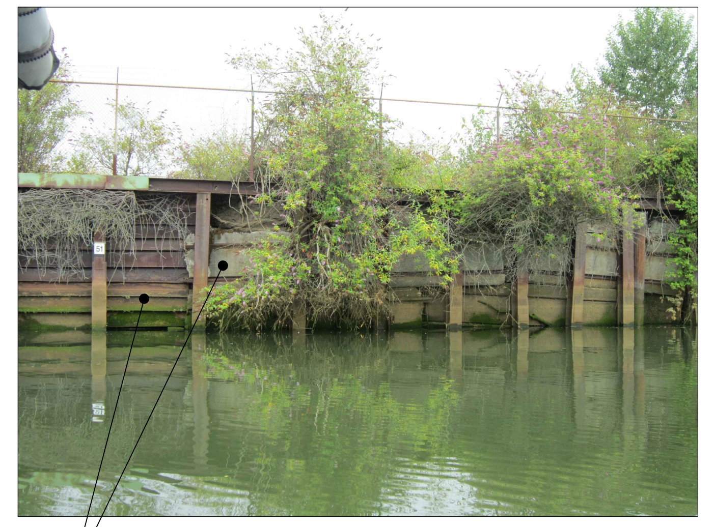
STEEL H-PILES WITH STEEL AND CONCRETE PANEL RUBBLE LAGGING
