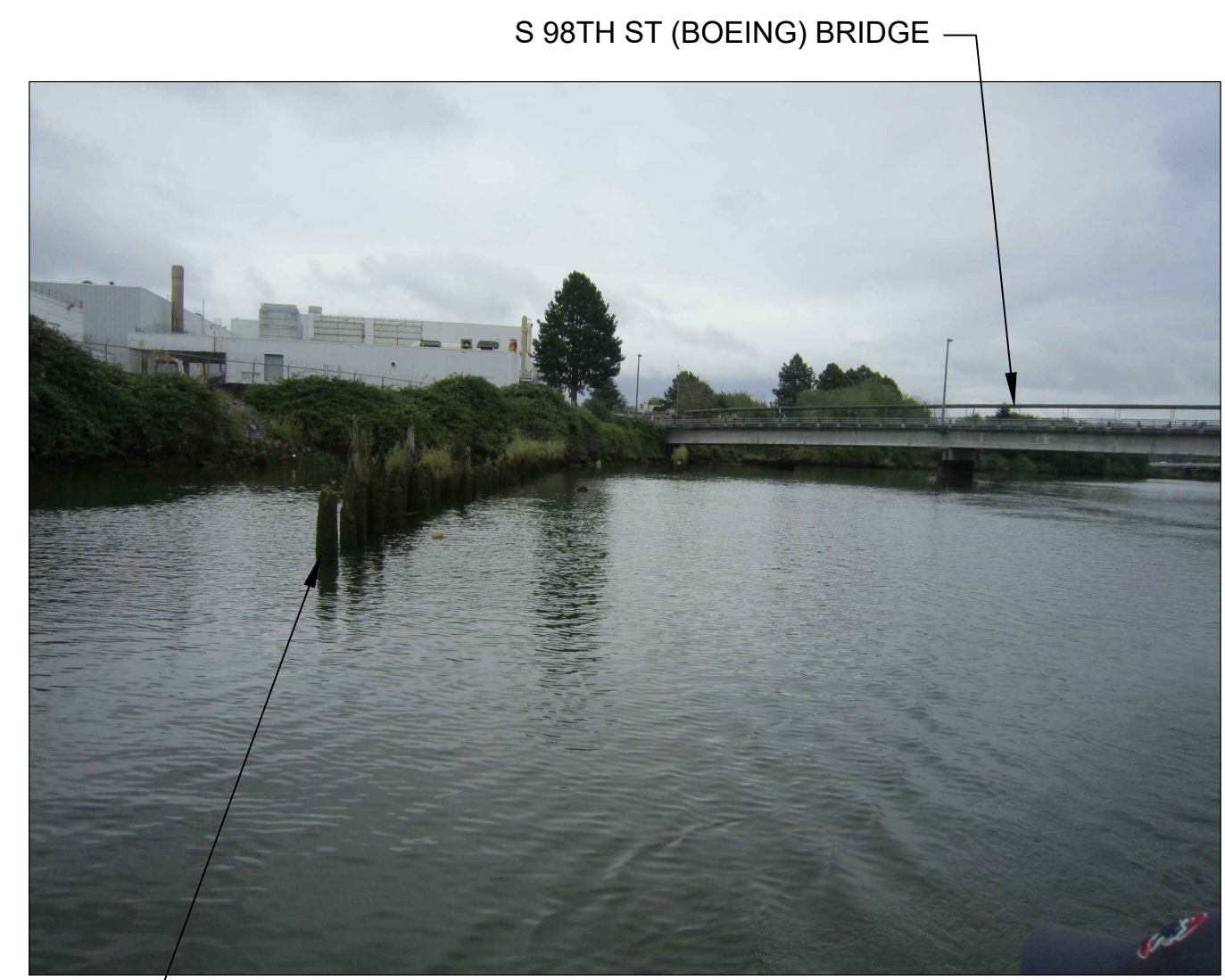
GROIN PILES TO REMAIN GROIN PILES PHOTO SCALE: NONE
