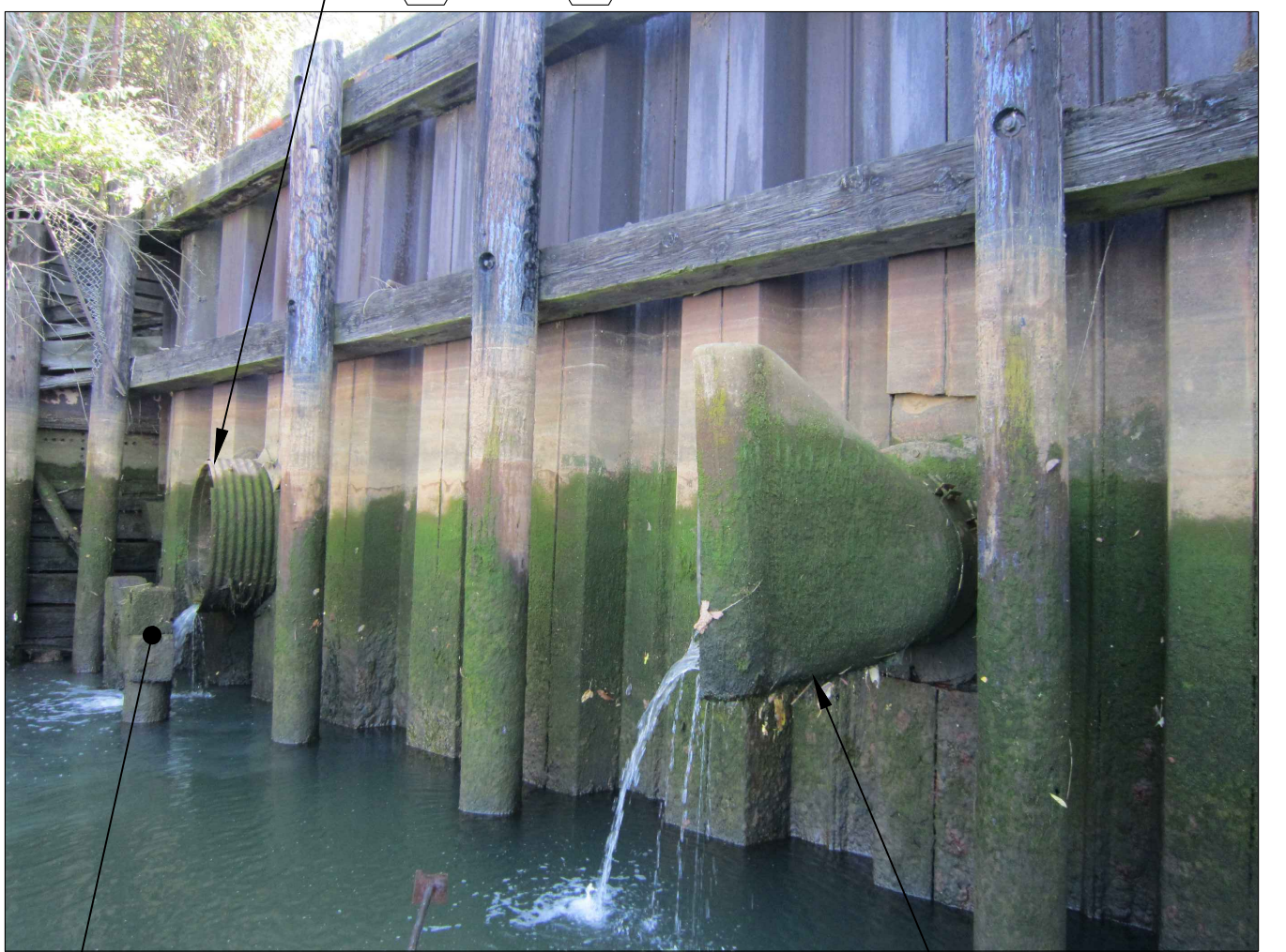
OUTFALL 2061 (6) PIPE SADDLE TO BE REMOVED PHOTO SCALE: NONE (3)
