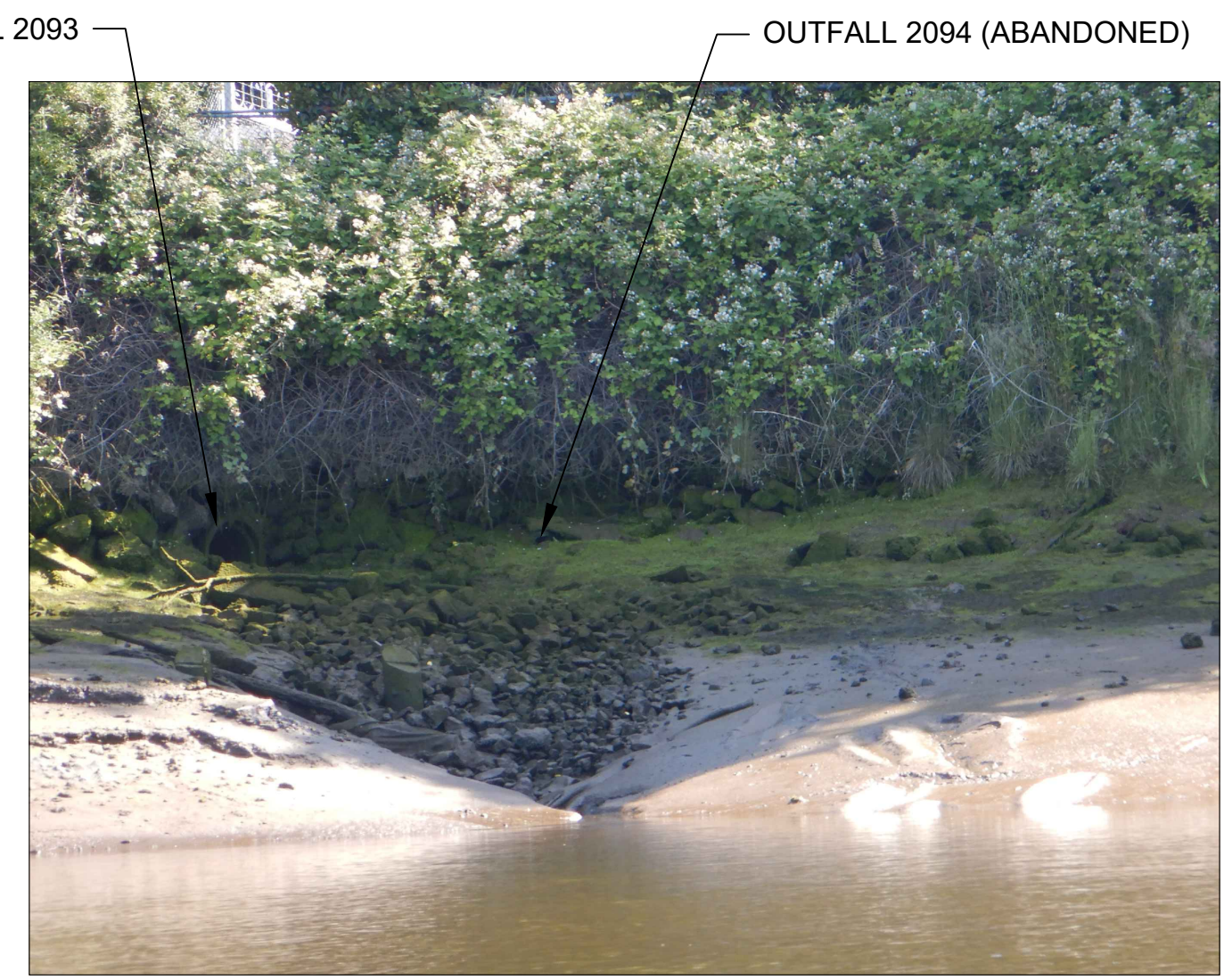
OUTFALLS PHOTO SCALE: NONE
