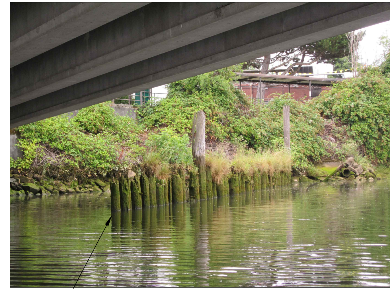
GROIN PILES TO REMAIN GROIN PILES PHOTO SCALE: NONE
