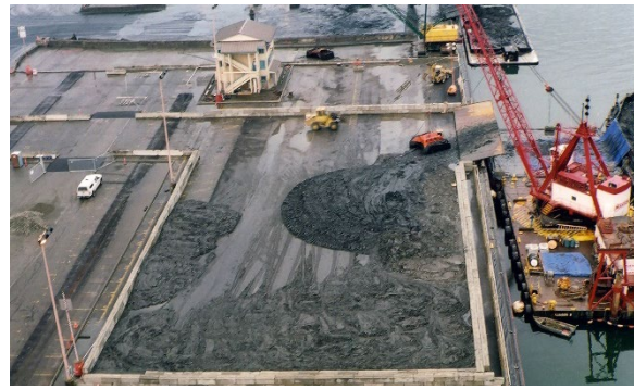
Contained landside facility
