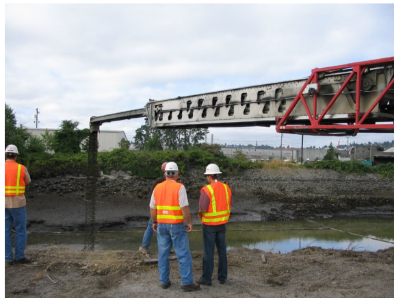
Variable speed telebelt placement
