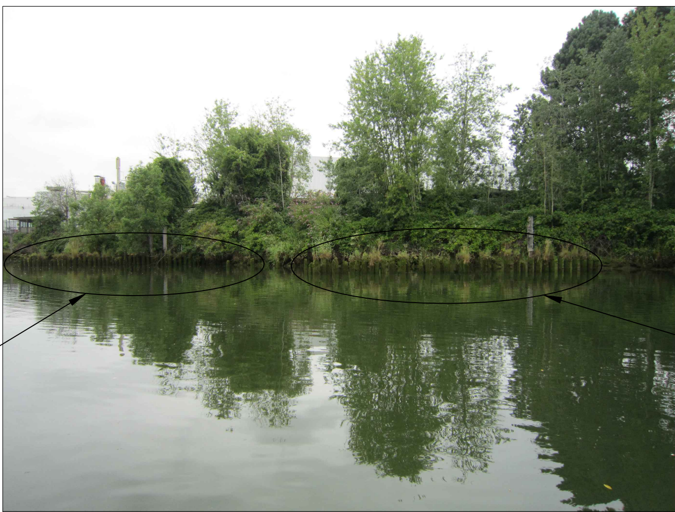
GROIN PILES (LOOKING EAST)
