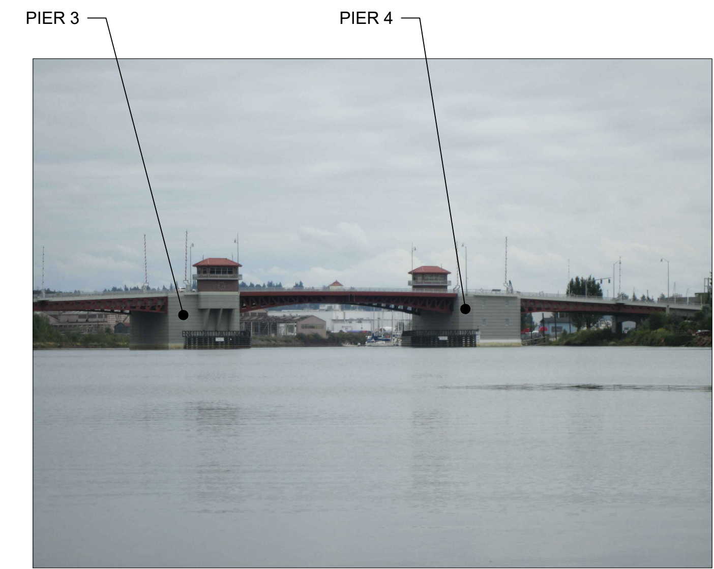
BASCULE BRIDGE (LOOKING DOWNSTREAM)
