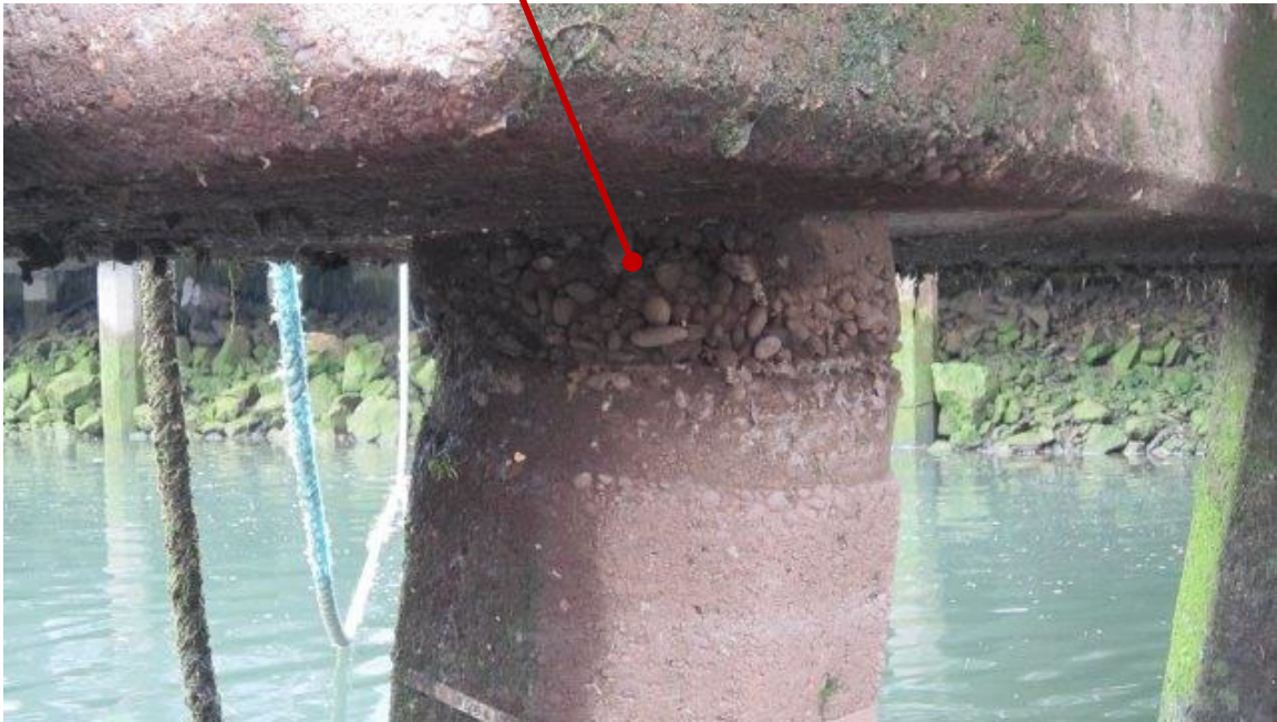
Photo ST05-23: Pier 5, Bent 1 East Cap Beam
