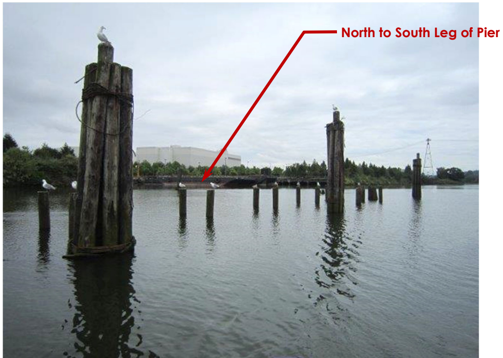
Photo ST04-02: L-Shaped Pier and Dolphins (Looking South)
