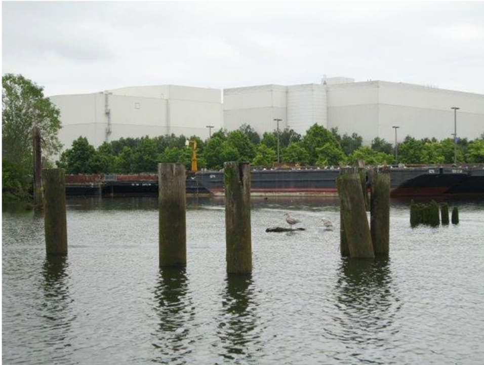
Photo ST04-03: South End of Pier
