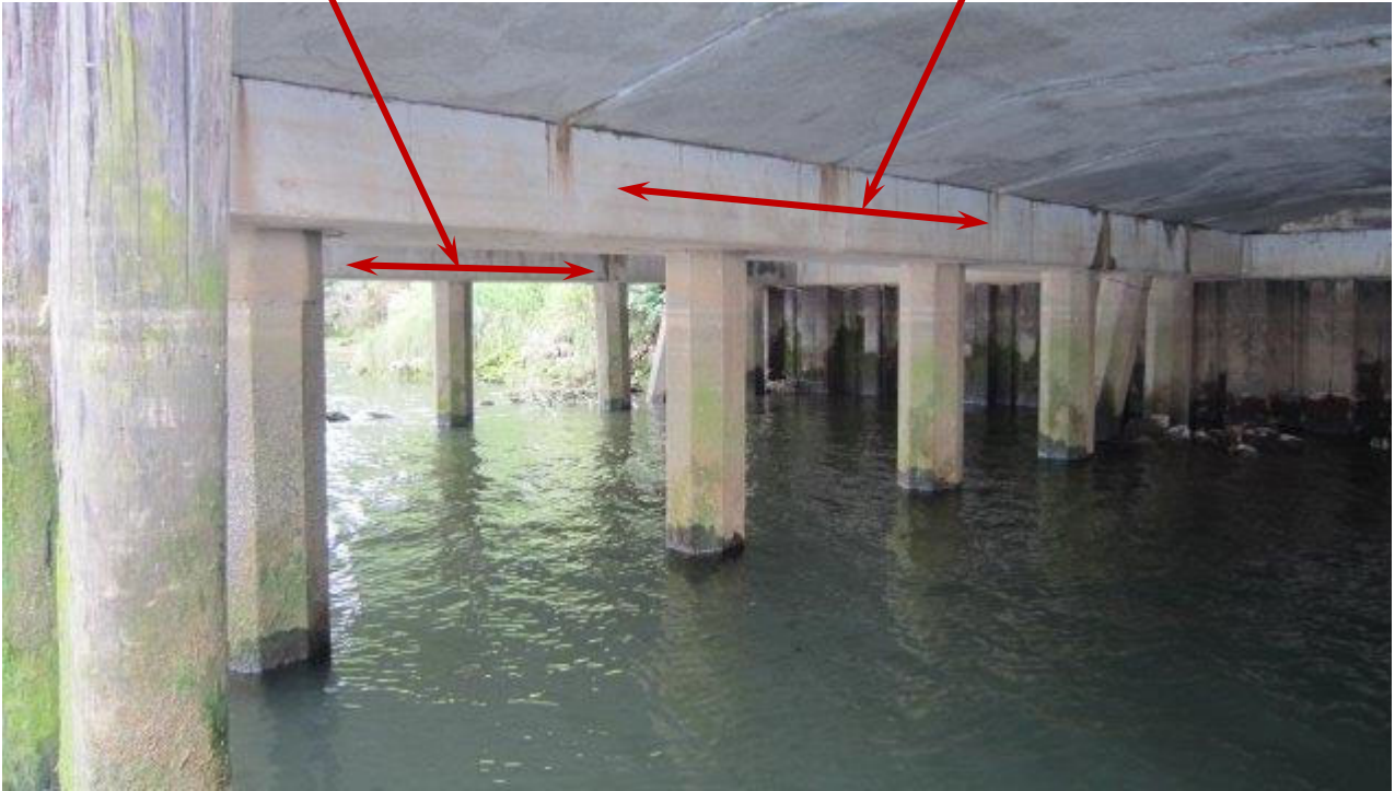
Photo ST16-11: Piles and Pile Caps (Looking Southwest)
