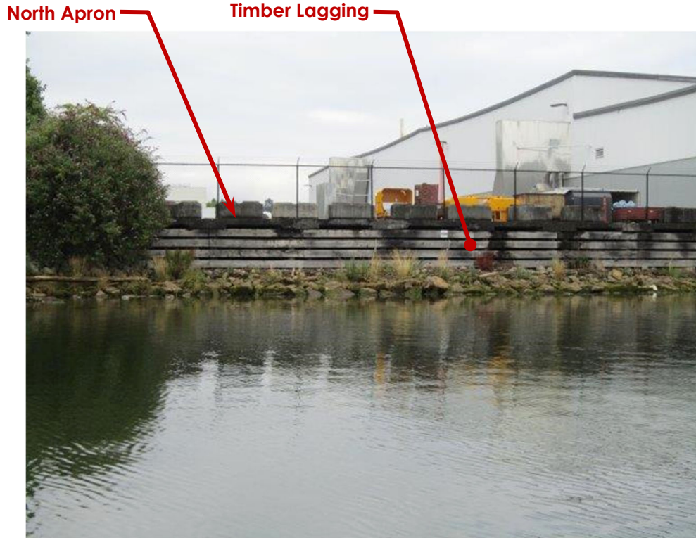
Photo ST38-01: North End (Looking East)
