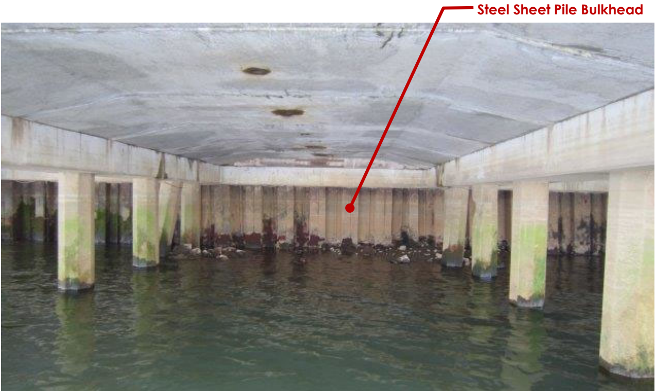
Photo ST16-014: Bulkhead and Pier Deck Soffit (Looking West)
