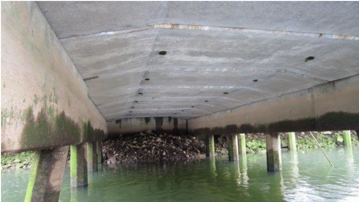
Photo ST05-24: Pier 5, Pier Deck Soffit
