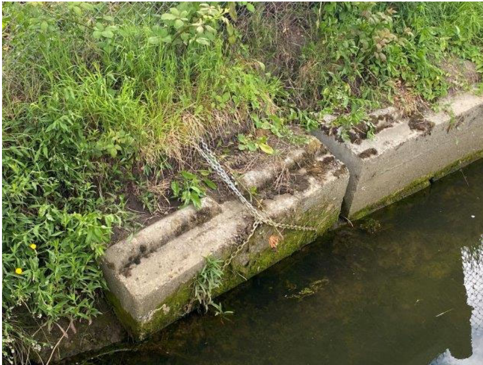
Photo ST20-05: Close Up of Chain Tie Back
