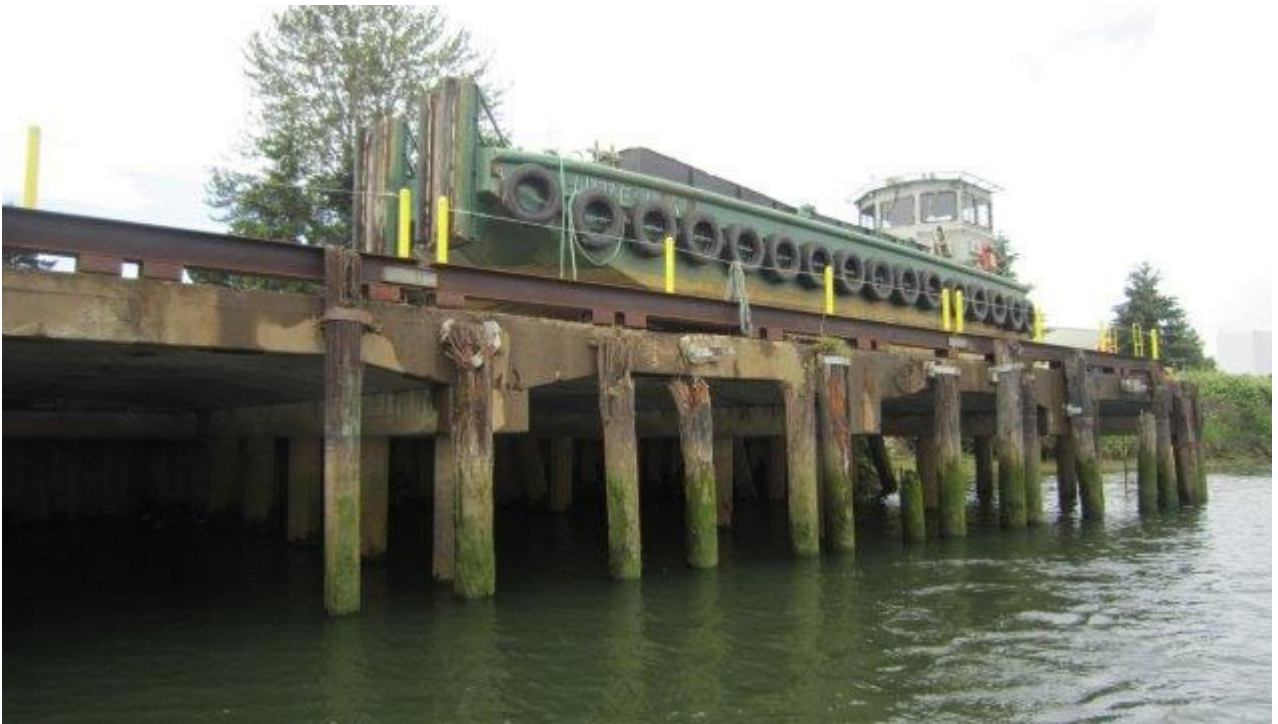
Photo ST16-02: Piers 2 to 4 (Looking Northwest)
