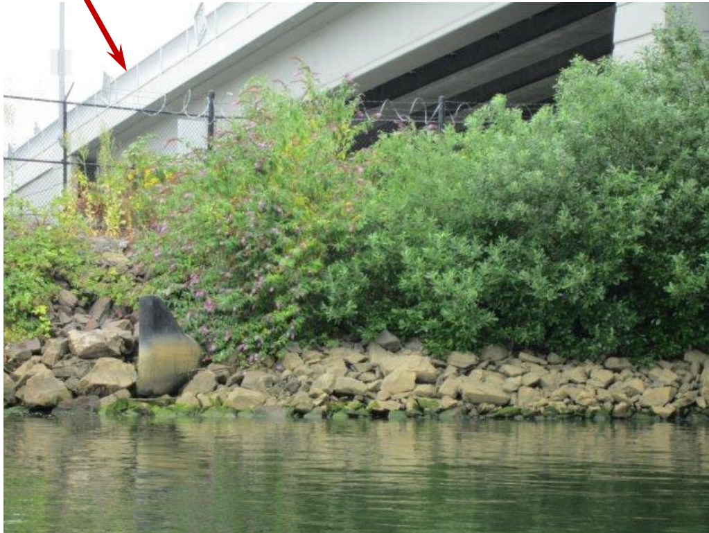
3031-02: Outfall (Looking Northeast)
