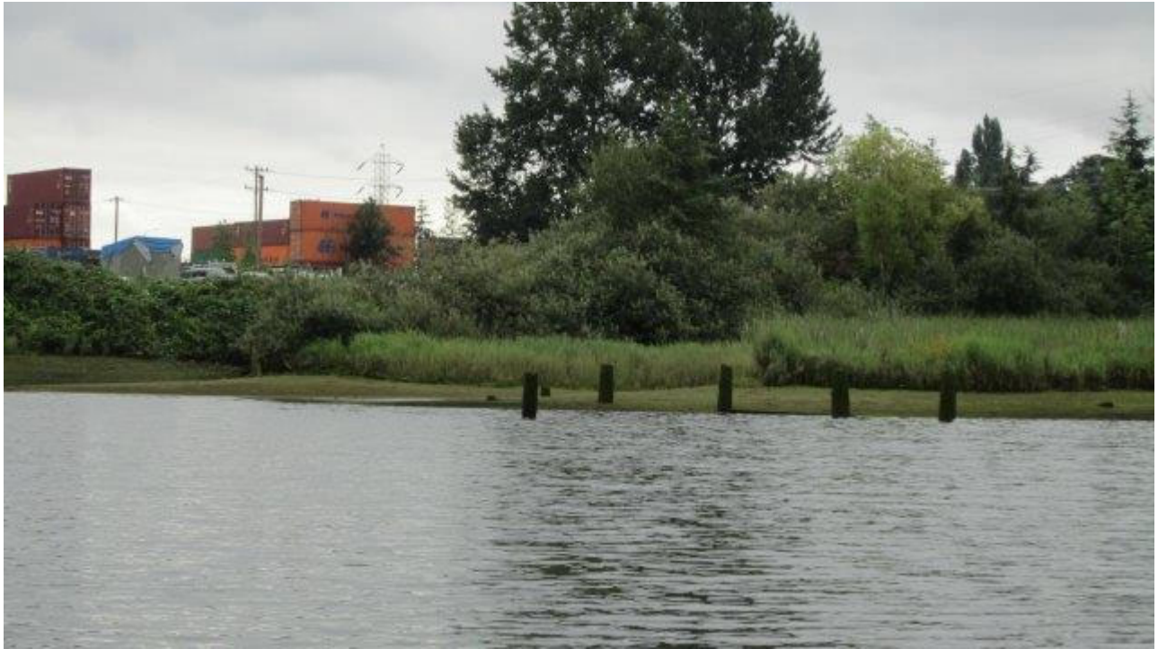
Photo ST10-01: Piles
