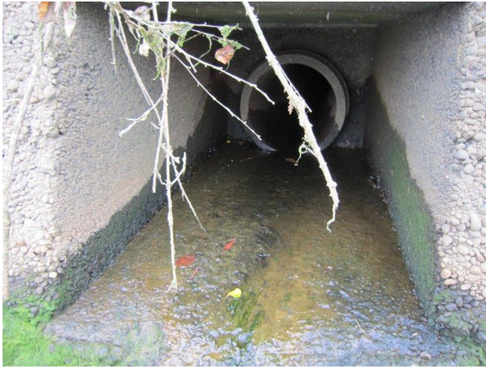
2073-03: Close Up of Outfall
