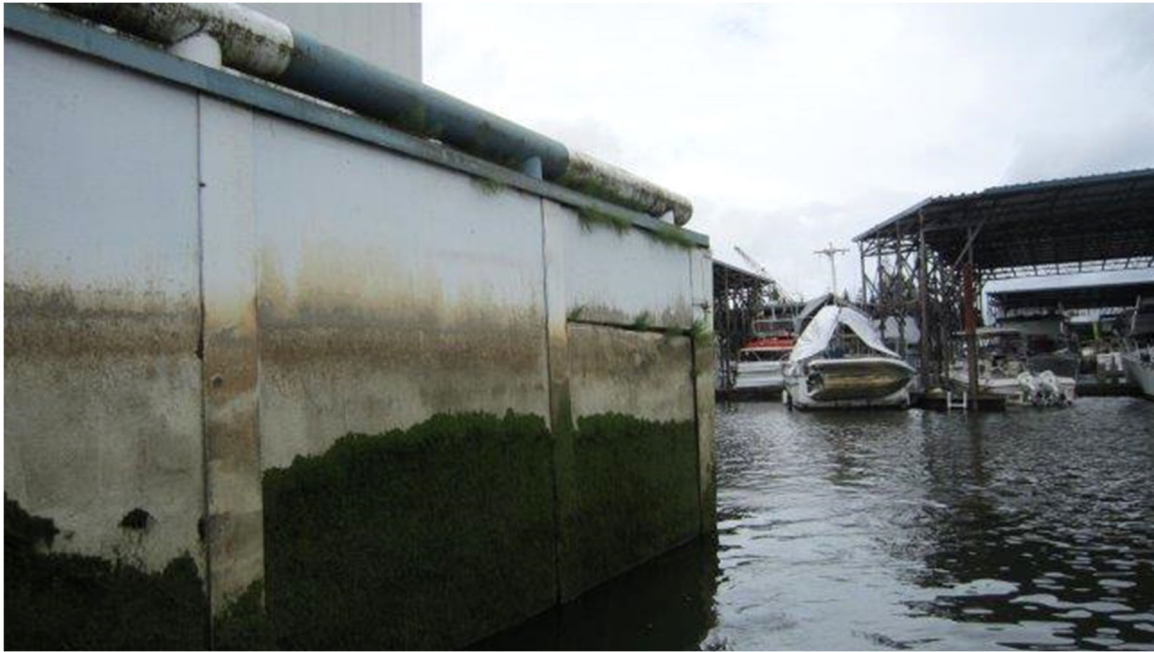
Photo ST12-13: North End Close Up of the H-Pile Bulkhead
