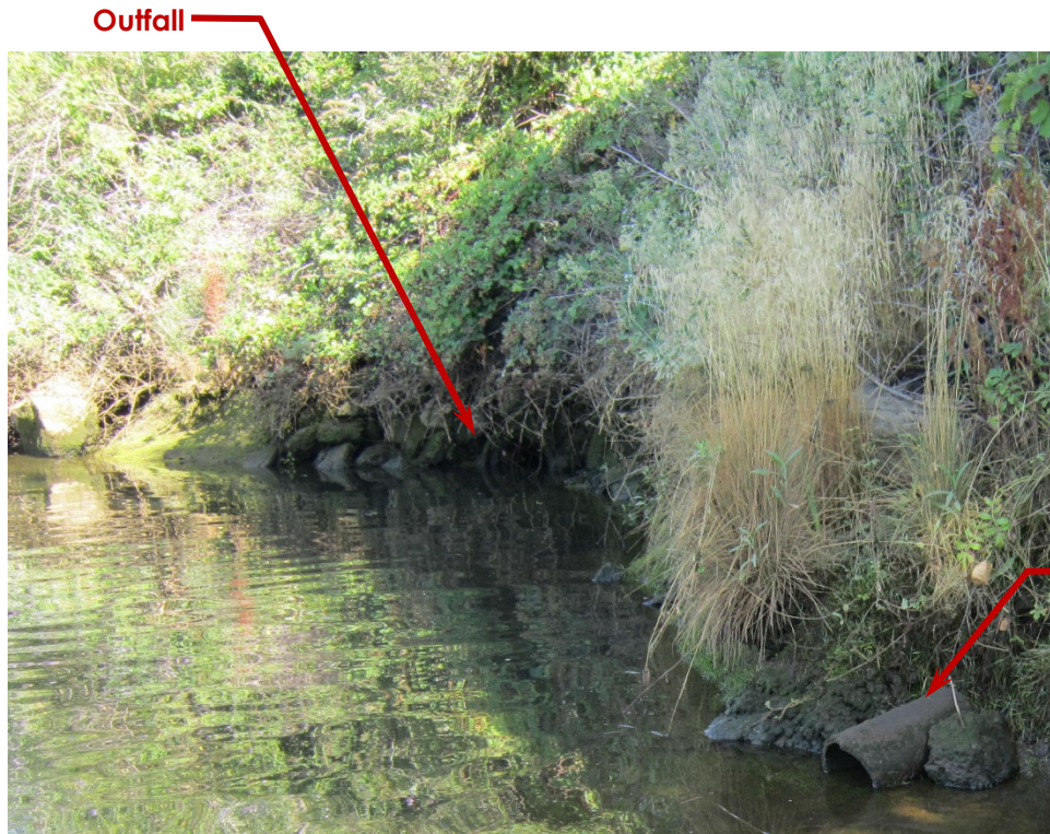
Photo 2093-02: Outfall (Looking Northeast)
