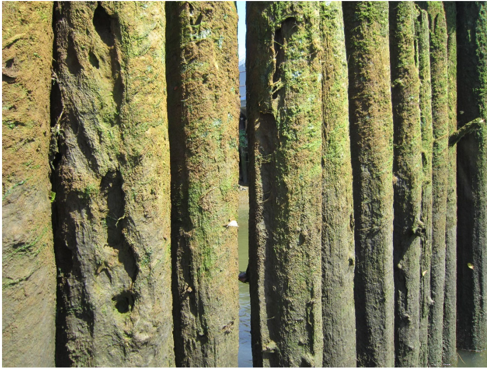
Photo ST07-09: Interior Groin Piles
