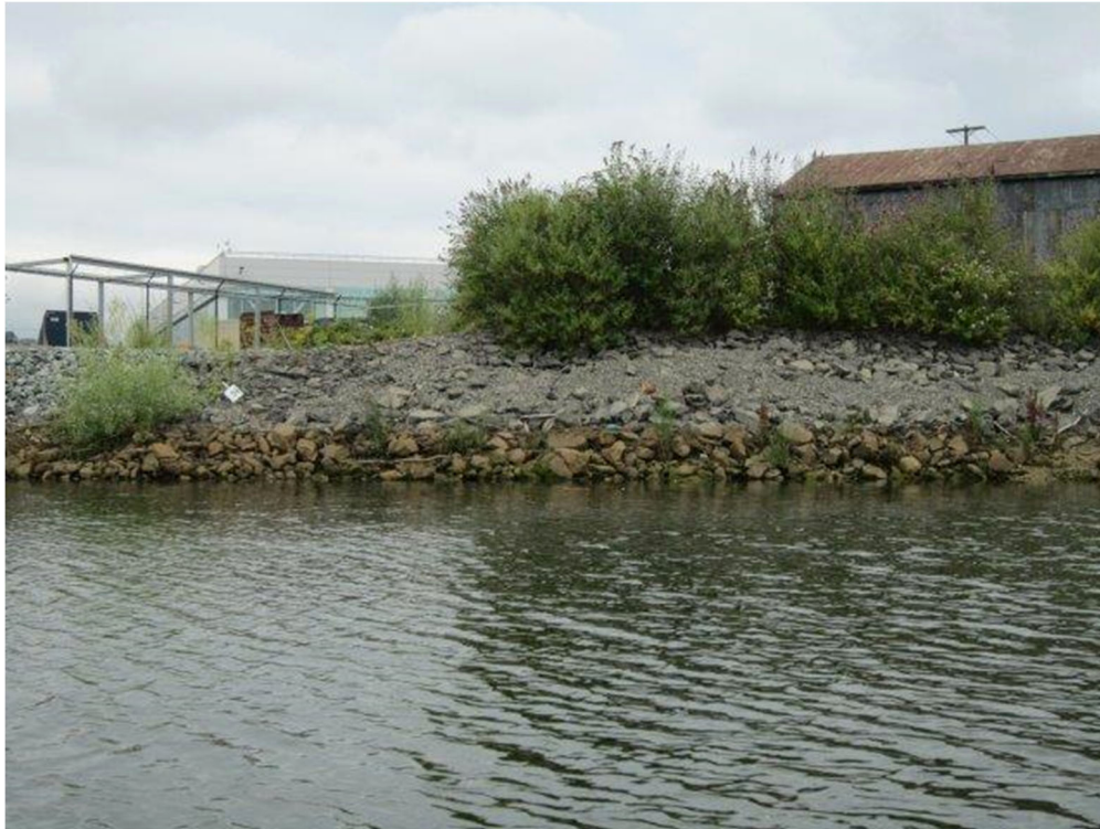
Photo ST03-03: Riprap Section
