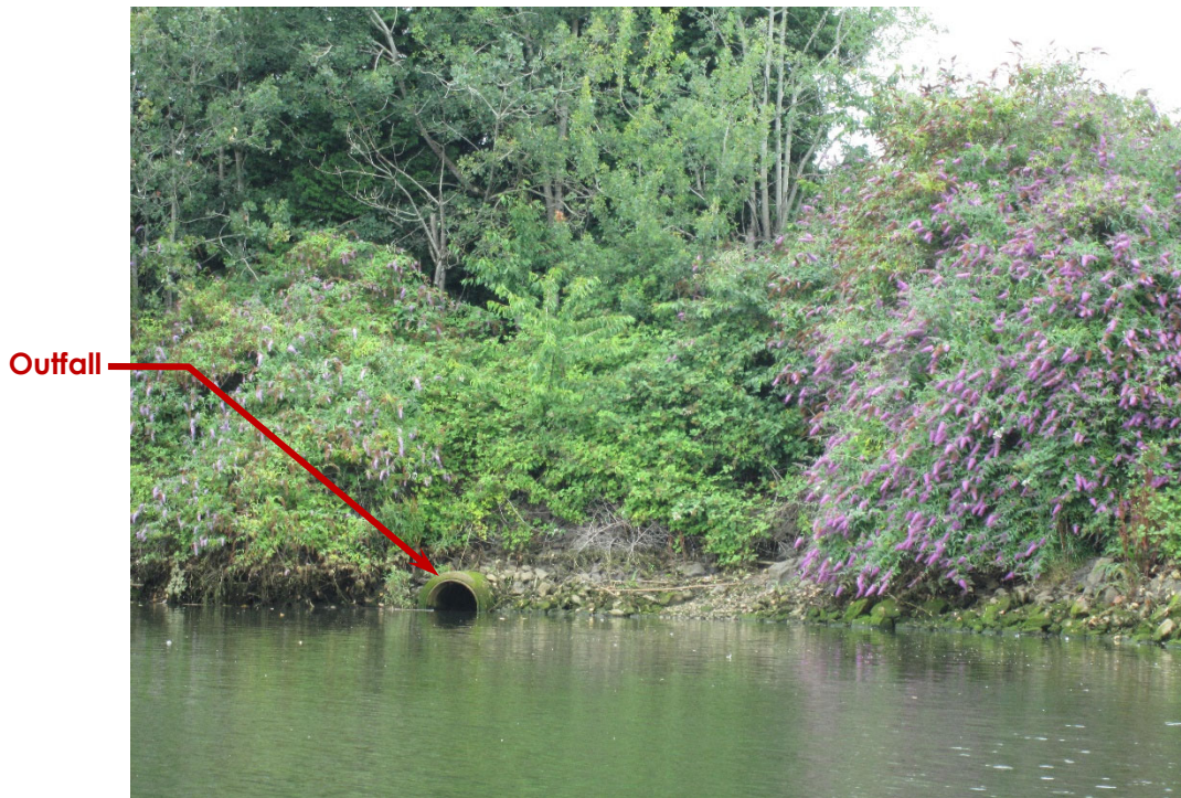
Photo BDC-1-02: Outfall South of Dolphin (Looking East)
