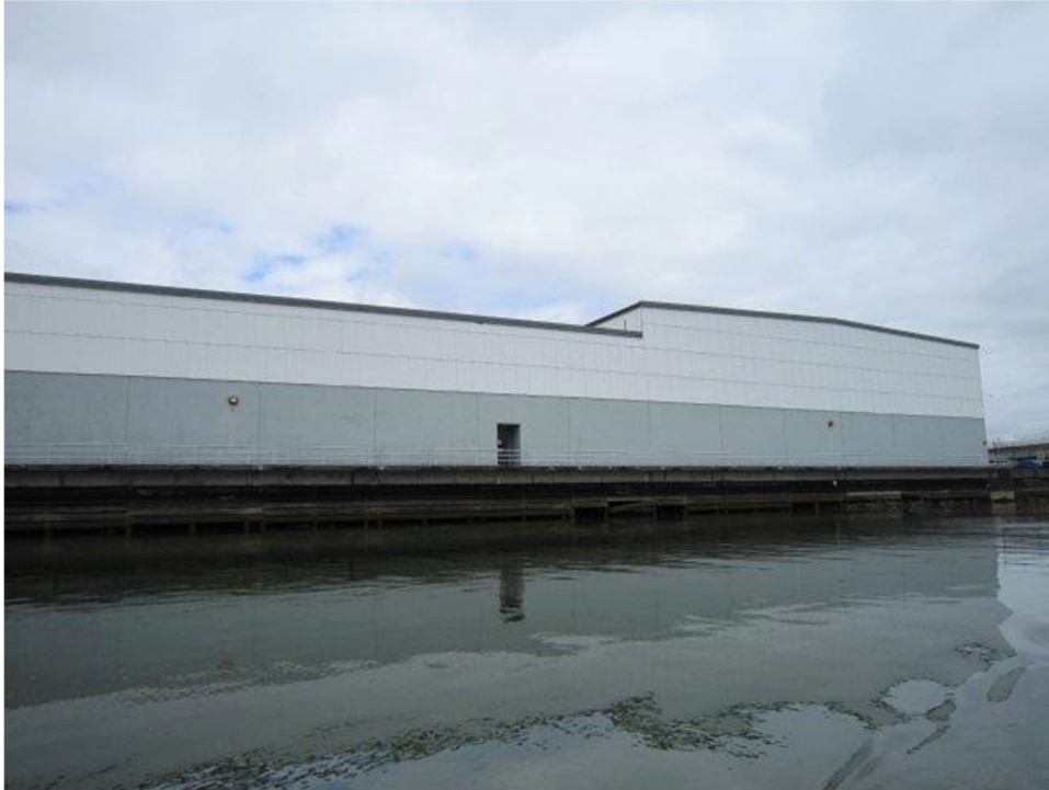
Photo ST38-03: Mid to South End of Building
