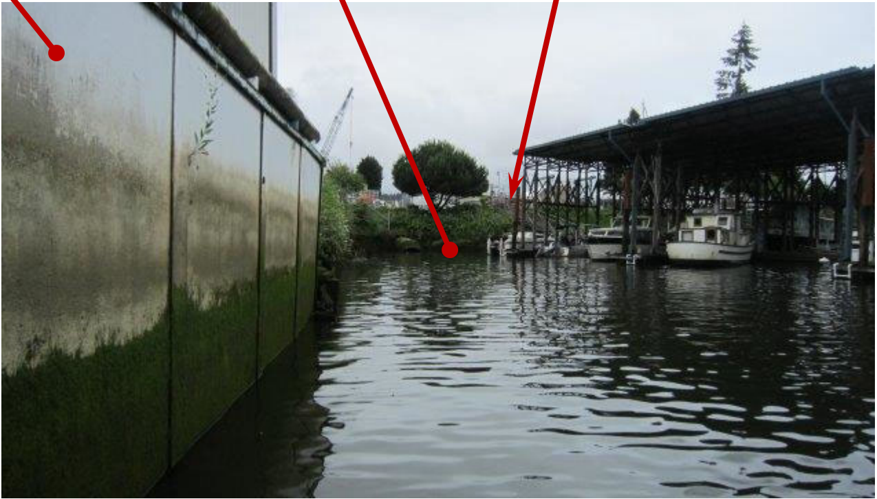
Photo ST15-01: South-most Float (Looking West)
