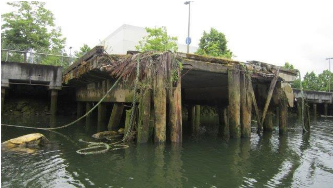
Photo ST05-09: Pier 2
