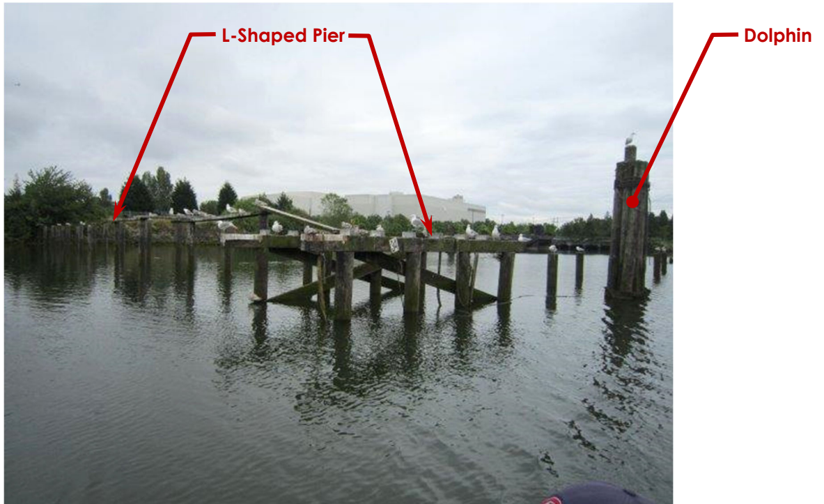
Photo ST04-01: L-Shaped Pier and Dolphins (Looking South)
