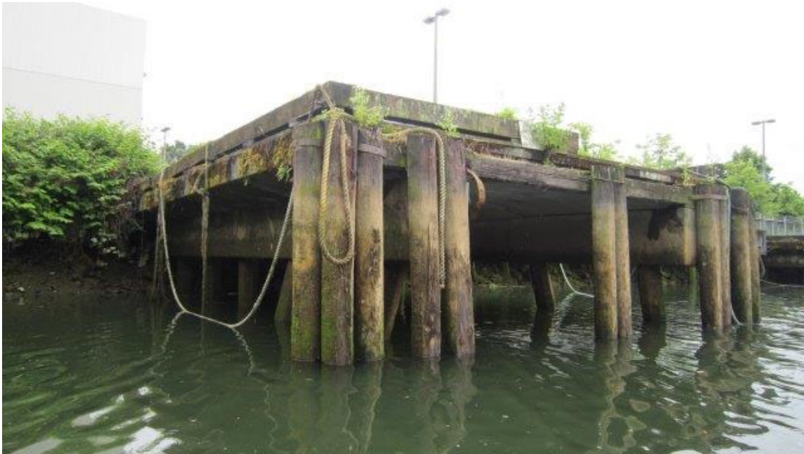
Photo ST05-01: Pier 1, East Most (Looking Southwest)
