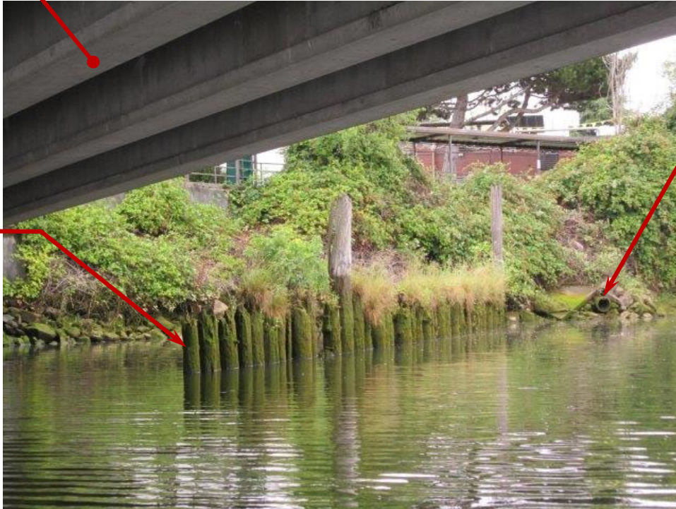
Photo 2092-01: Outfall (Looking East)
