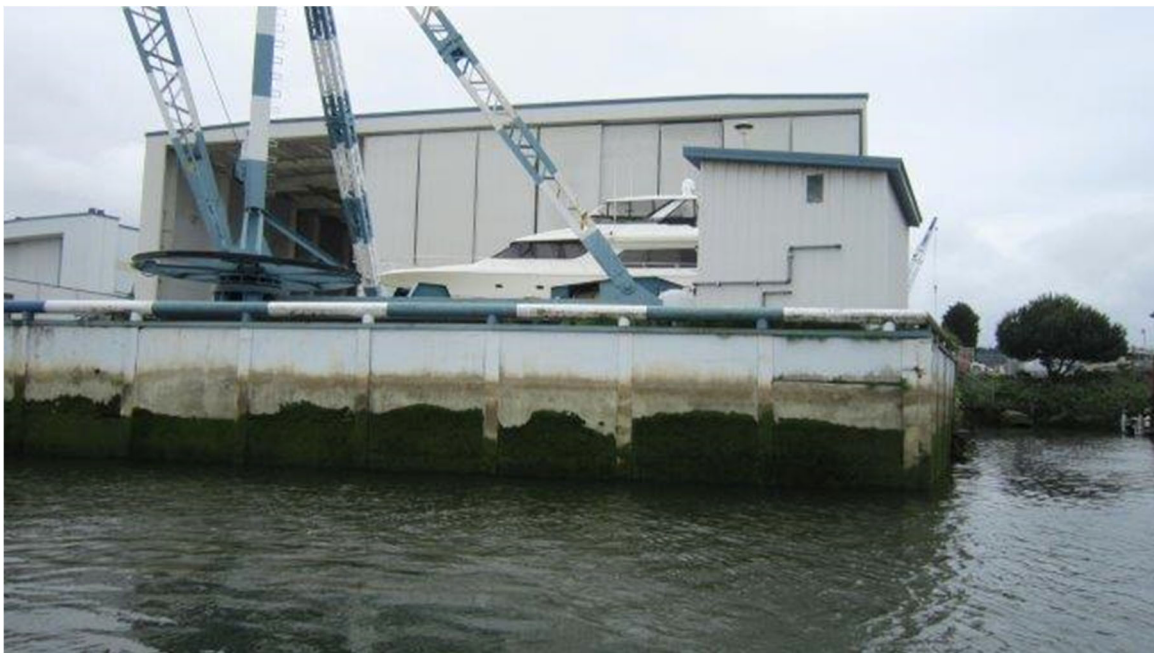
Photo ST12-12: North End Bulkhead and Return (Looking West)
