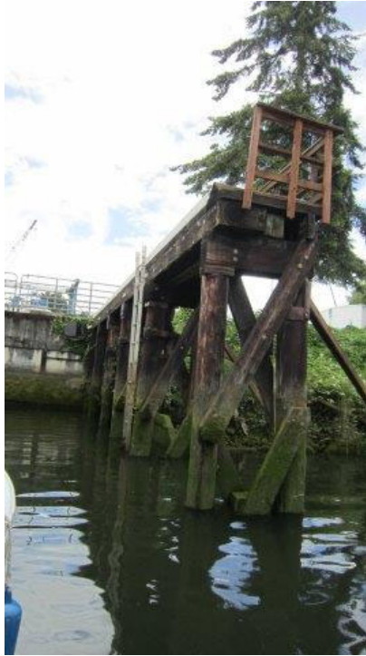
Photo ST14-03: North Bents
