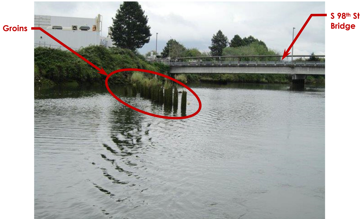
Photo ST07-11: Groins North of Bridge (Looking Southeast)
