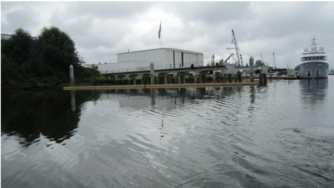
Photo ST12-016: Upstream Debris Deflector
