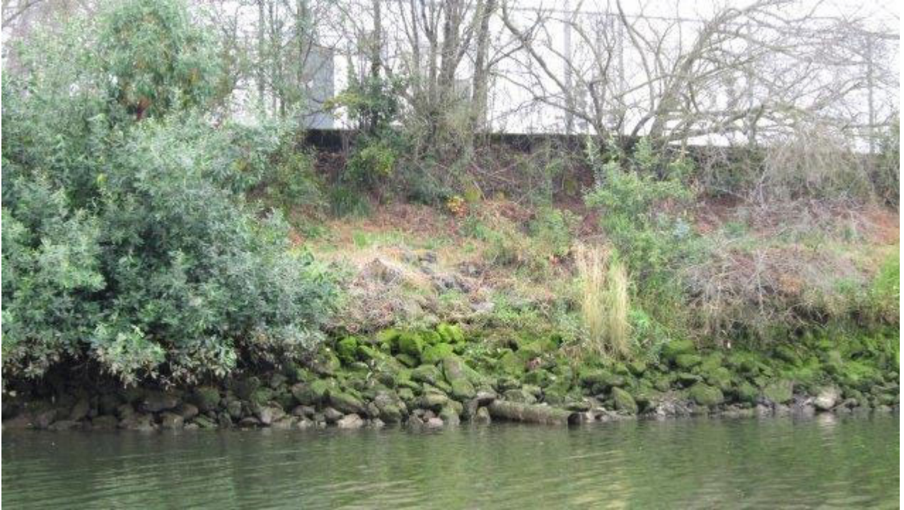
Photo 2098-01: Outfall (Looking West)
