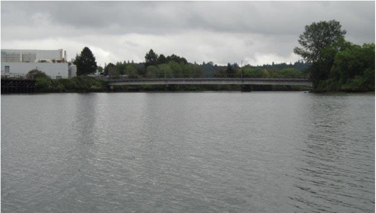
Photo ST08-01: Bridge (Looking South)
