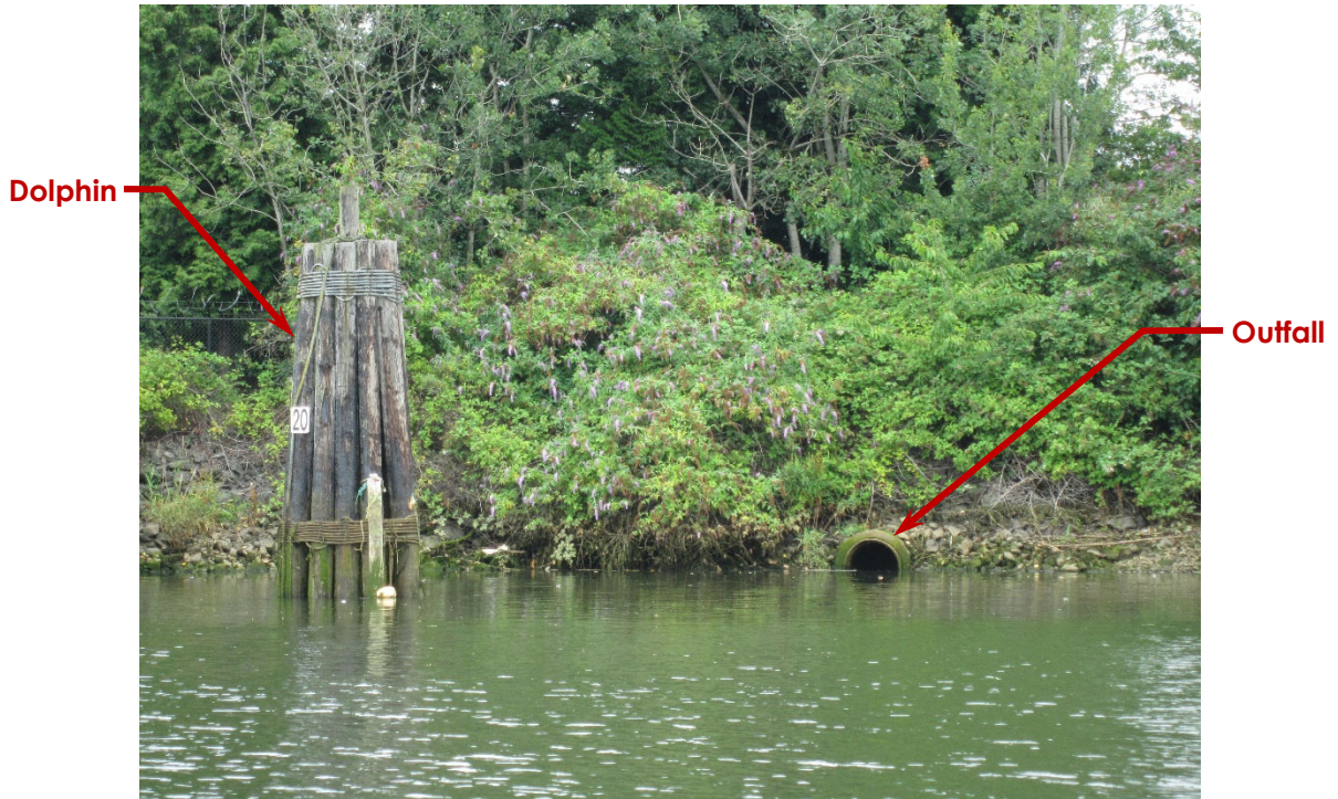
Photo BDC-1-01: Outfall South of Dolphin (Looking East)
