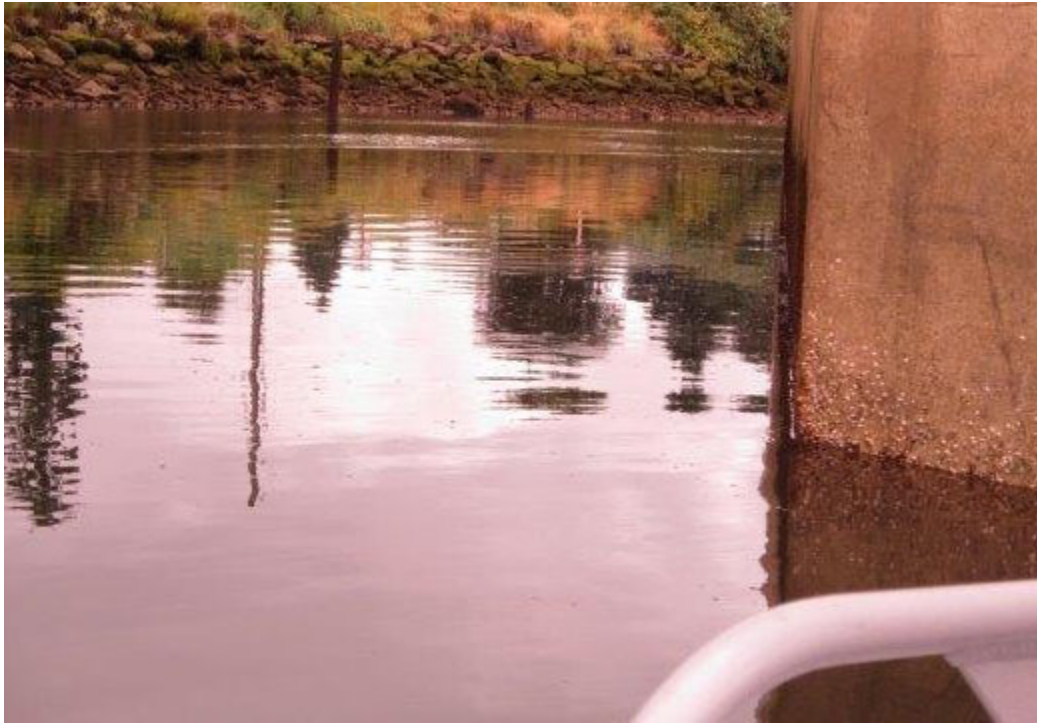
ST02-05: West Bascule Pier (south)
