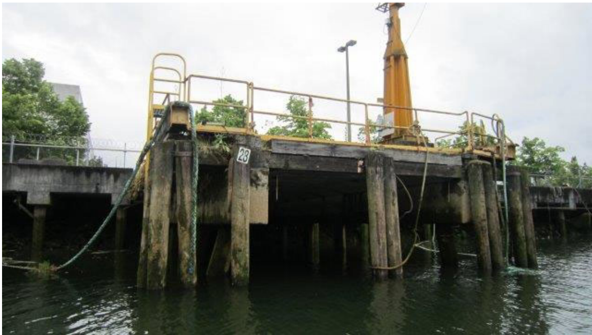
Photo ST05-19: Pier 4
