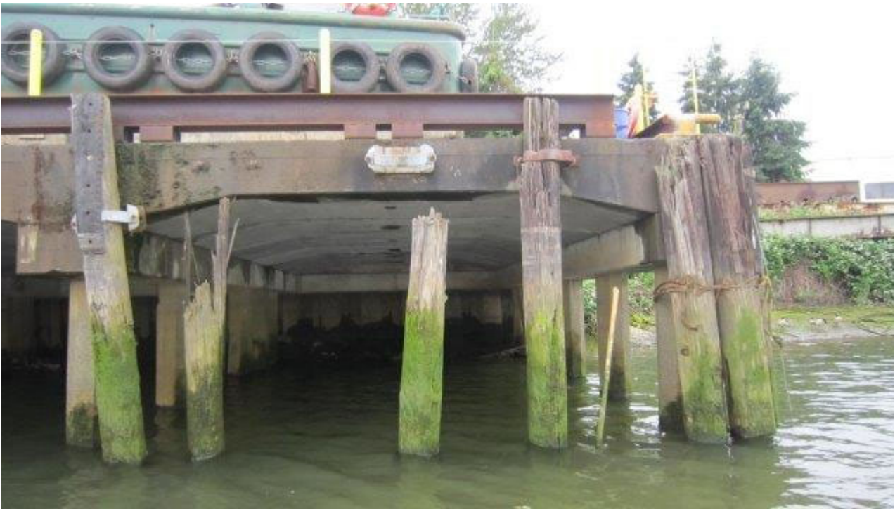
Photo ST16-016: Pier 4 Pier Deck (North Most, Looking West)
