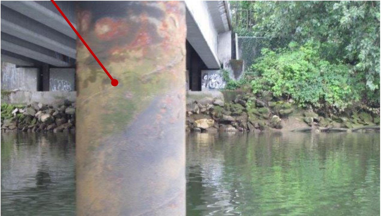
Photo ST08-05: West Bent (Looking West)
