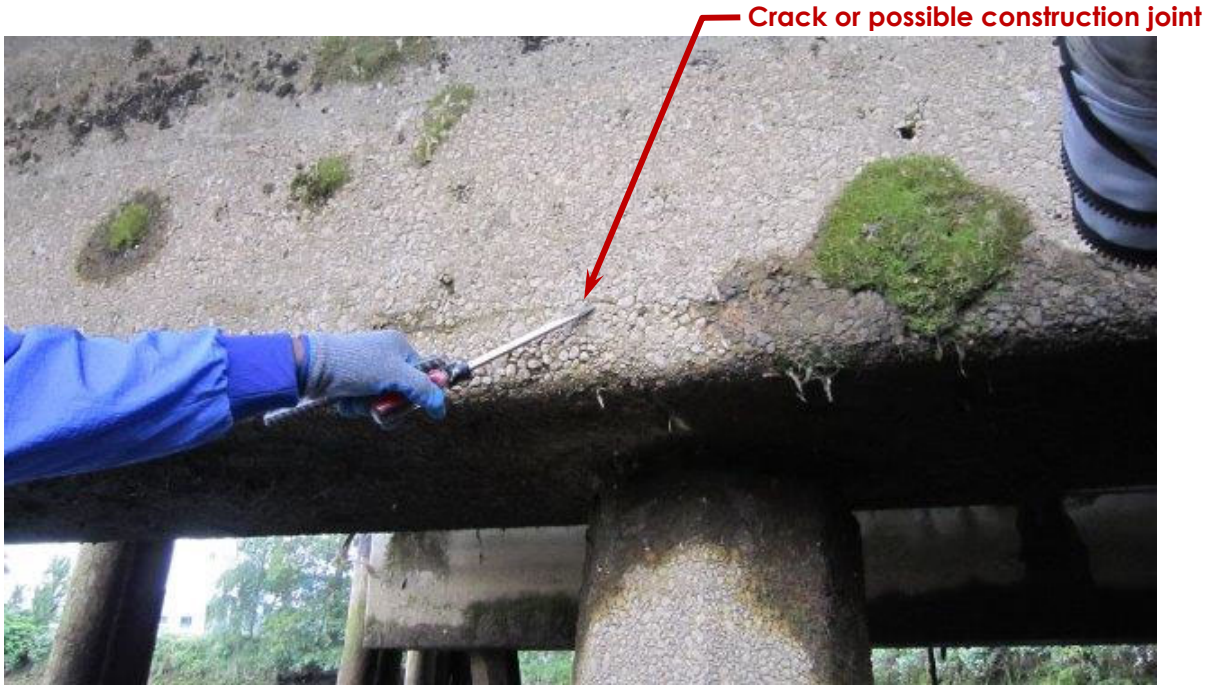
Photo ST05-05: Pier 1, West Side of West Pile Cap
