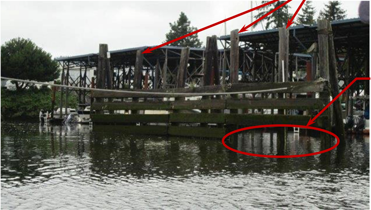
Photo ST13-01: Breakwater (Looking Northwest)
