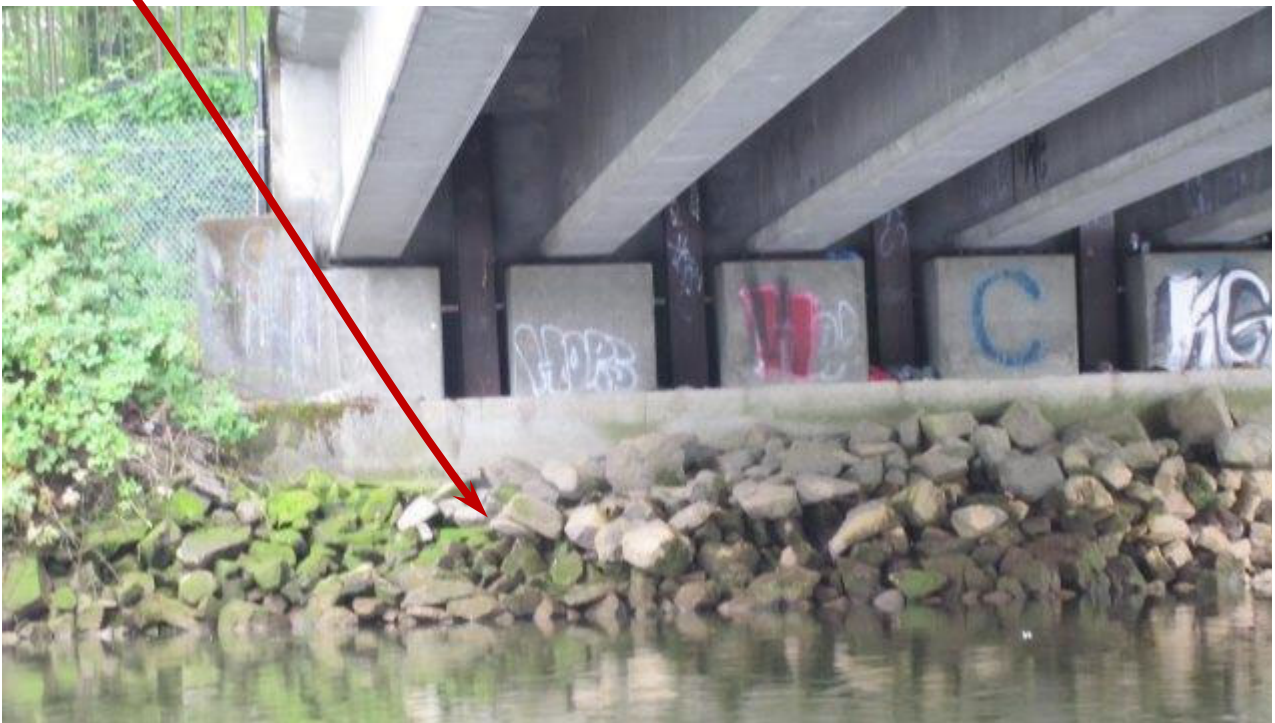
Photo ST08-02: East Abutment
