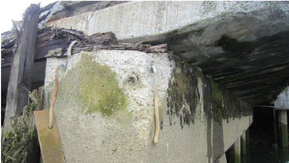
Photo ST05-11: Pier 2, West Cap Beam
