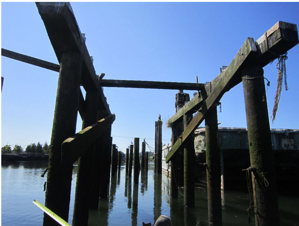
Photo ST04-04: Pile Bent Looking South
