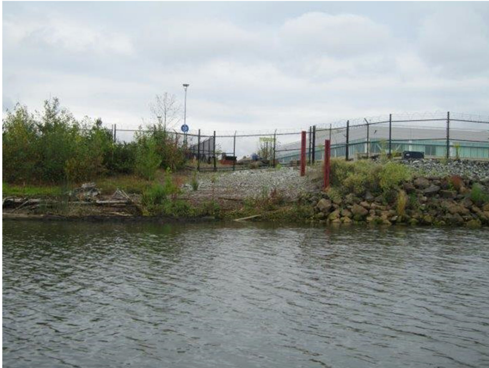
Photo ST03-01: Riprap Section
