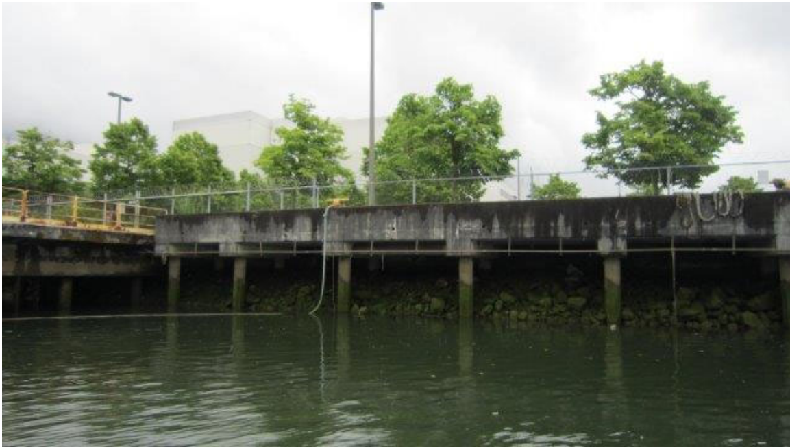
Photo ST05-21: Wharf Between Pier 4 and Pier 5
