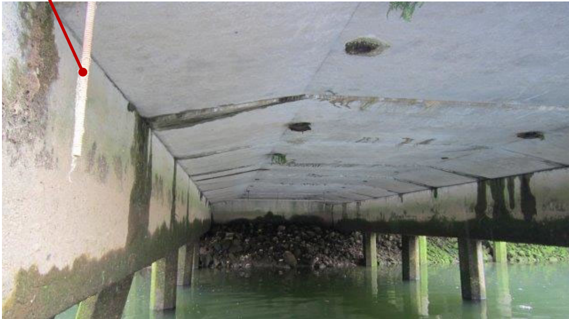
Photo ST05-20: Pier 4, Pier Deck Soffit
