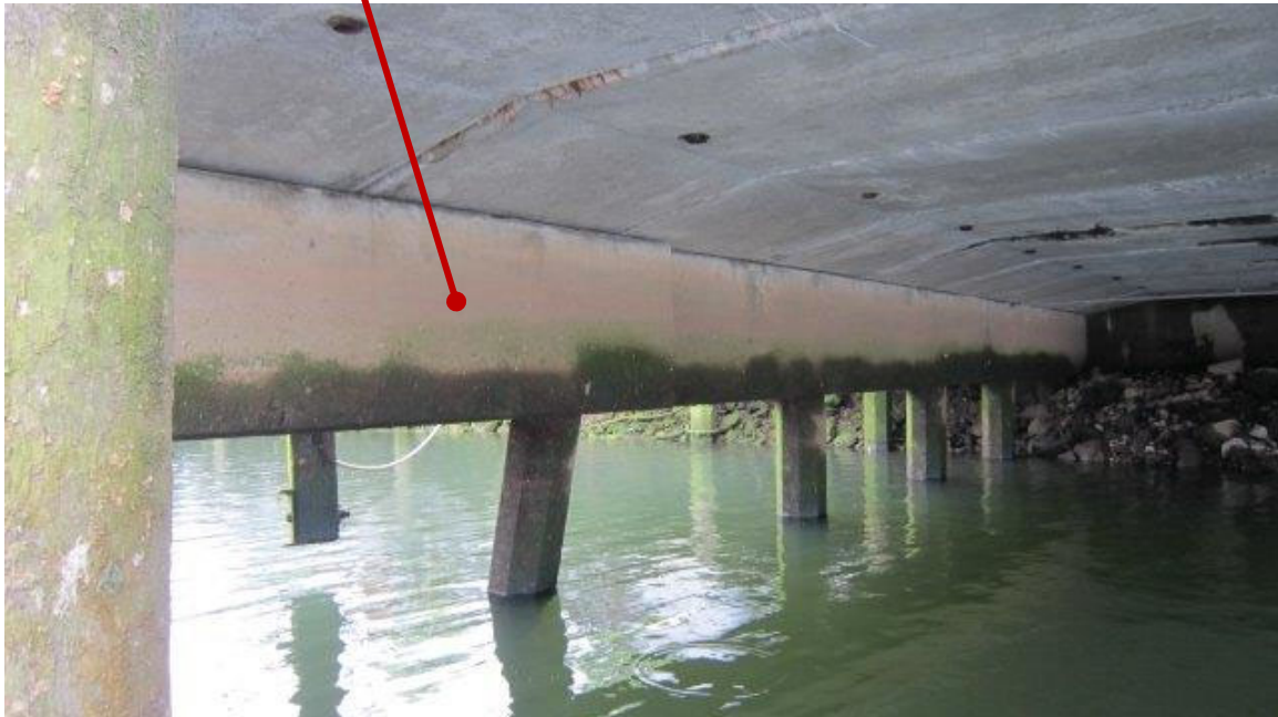
Photo ST05-28: Pier 6, East Pile Cap
