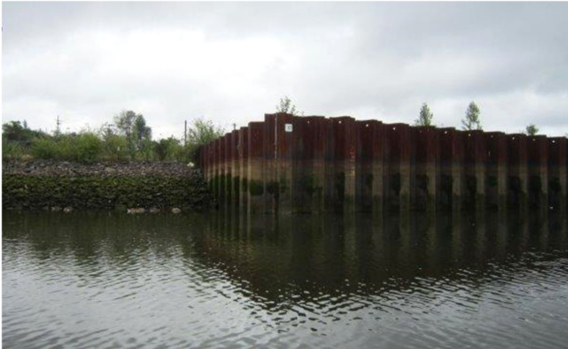
Photo ST19-01: South Return Wall (Looking Northwest)
