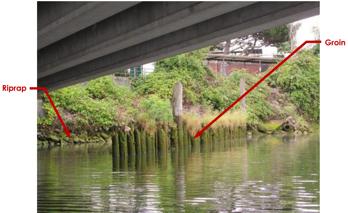
Photo ST07-13: Groins and Embankment South of Bridge
