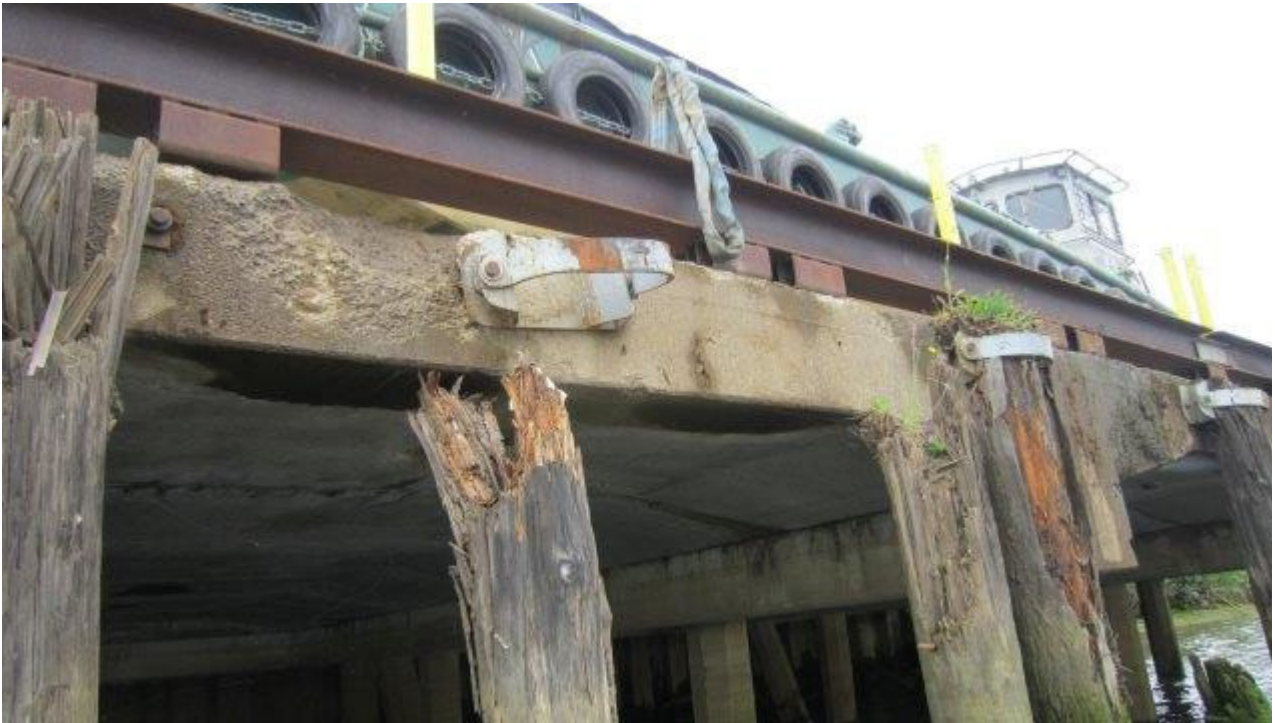
Photo ST16-12: Pier 3 Pier Deck
