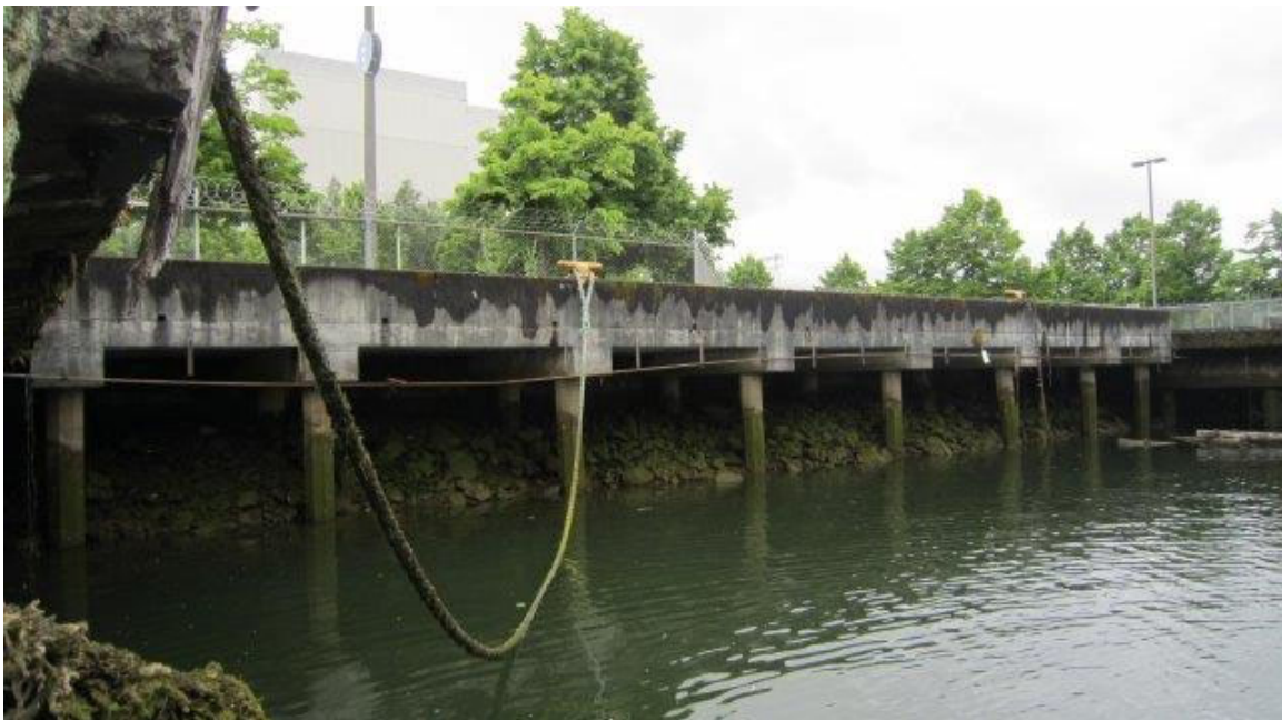
Photo ST05-14: Wharf Between Pier 2 and Pier 3
