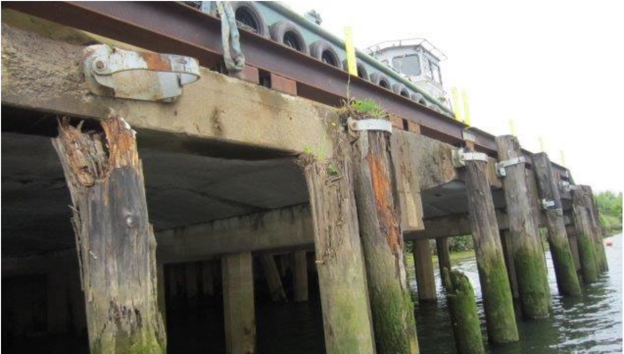
Photo ST16-13: Pier 4 Pier Deck
