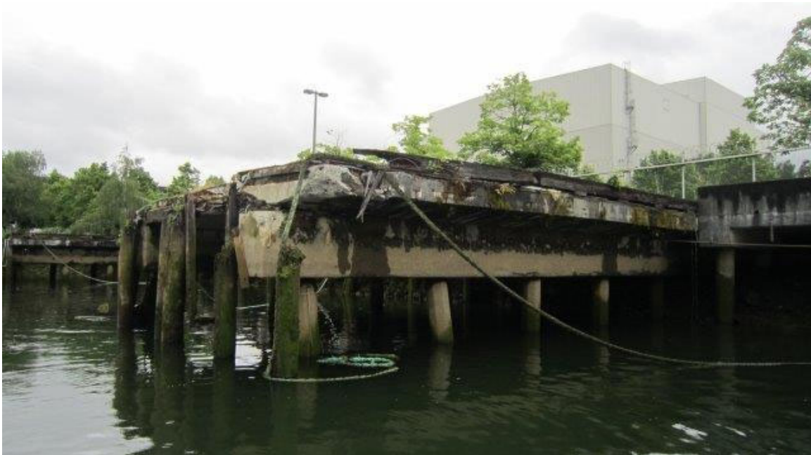
Photo ST05-10: Pier 2 (Looking Southeast)
