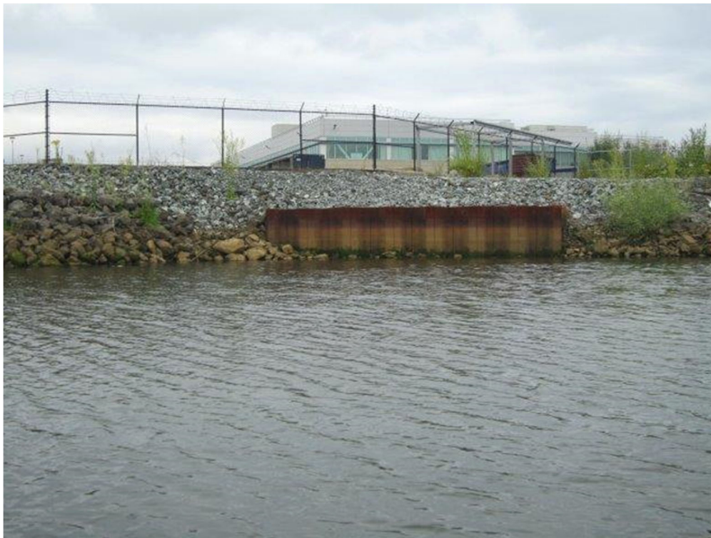
Photo ST03-02: Sheet Pile Bulkhead Section
