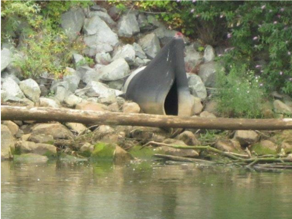
Boeing Plant 2 ————— Boeing 1-01: Outfall North of Building
