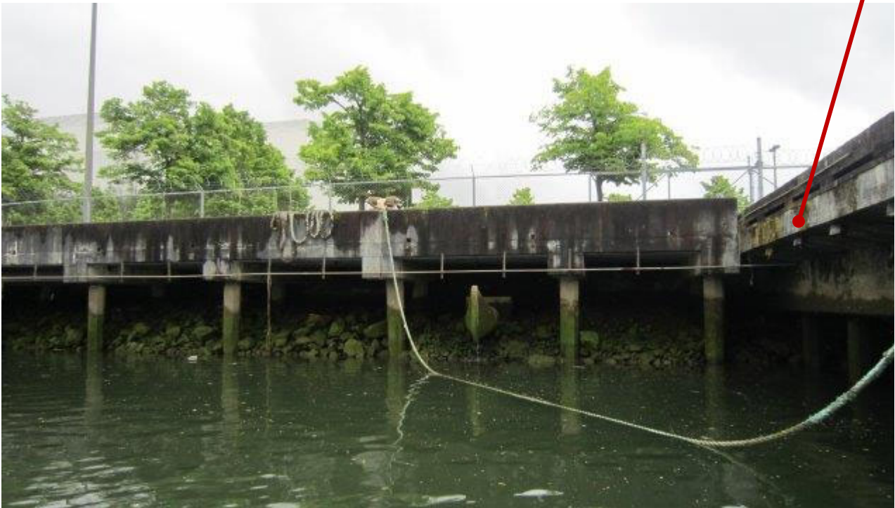
Photo 2082-01: Outfall Between Piers 4 and 5 (Looking South)
