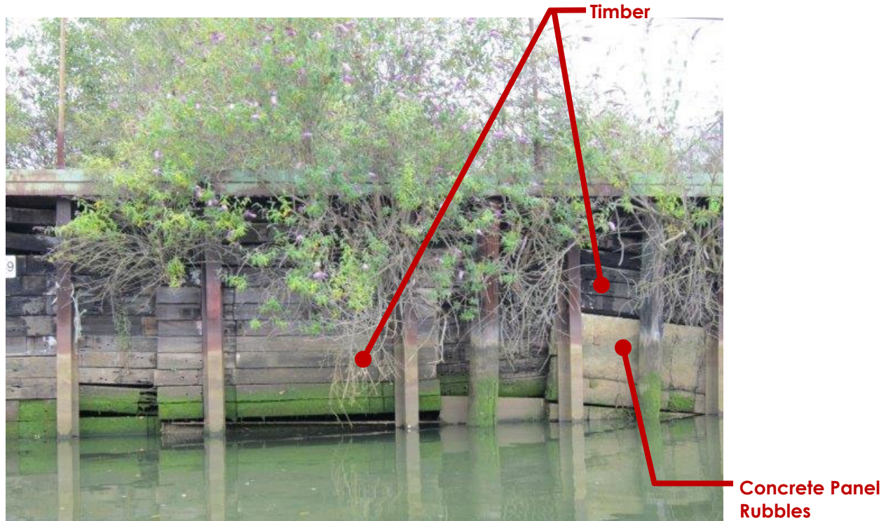
Photo ST03-15: H-Pile with Timber Lagging
