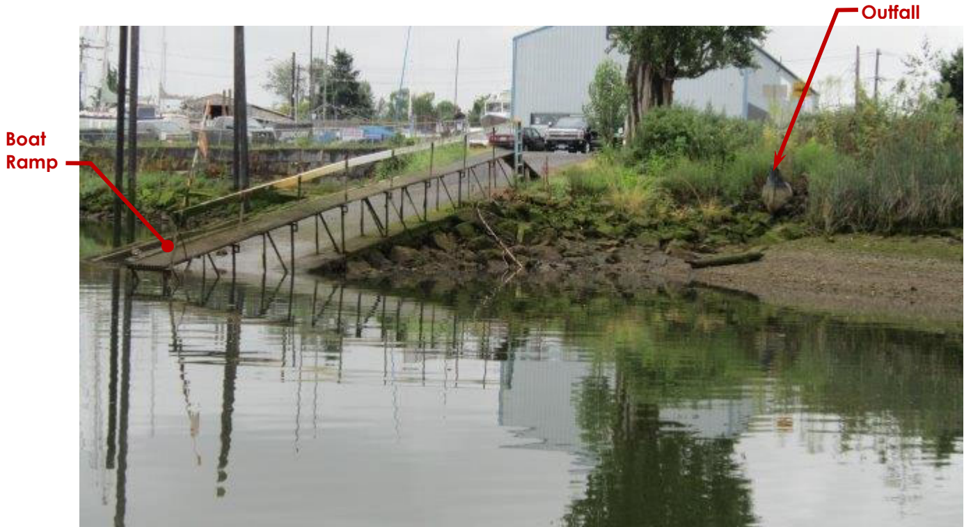
Photo 2215-03: Outfall (Looking Southwest)
