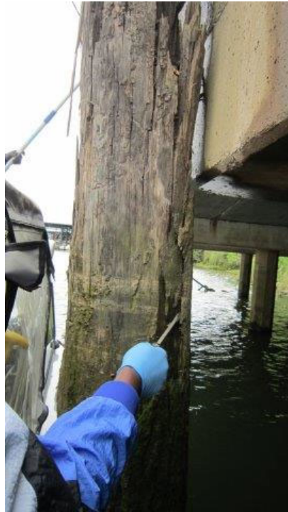
Photo ST16-05: Fender Pile
