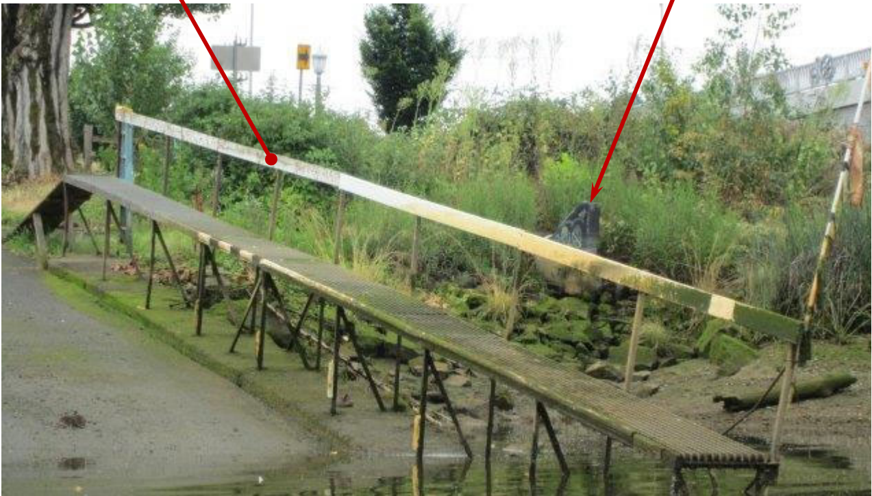
Photo 2215-02: Outfall (Looking Northwest)
