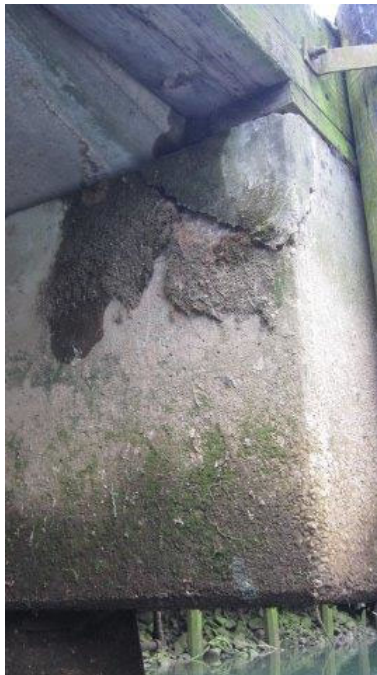
Photo ST05-04: Pier 1, East Side of West Pile Cap
