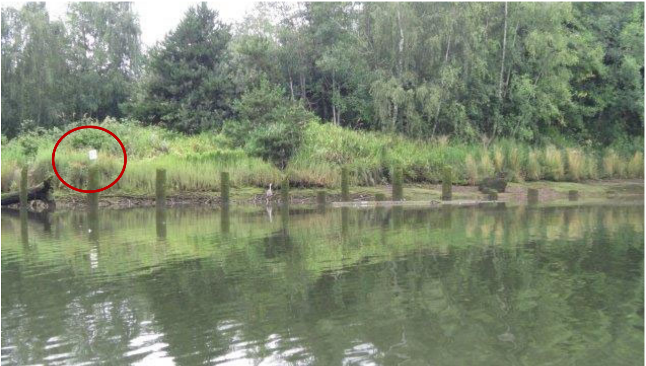
Photo ST11-02: North Pile Field
