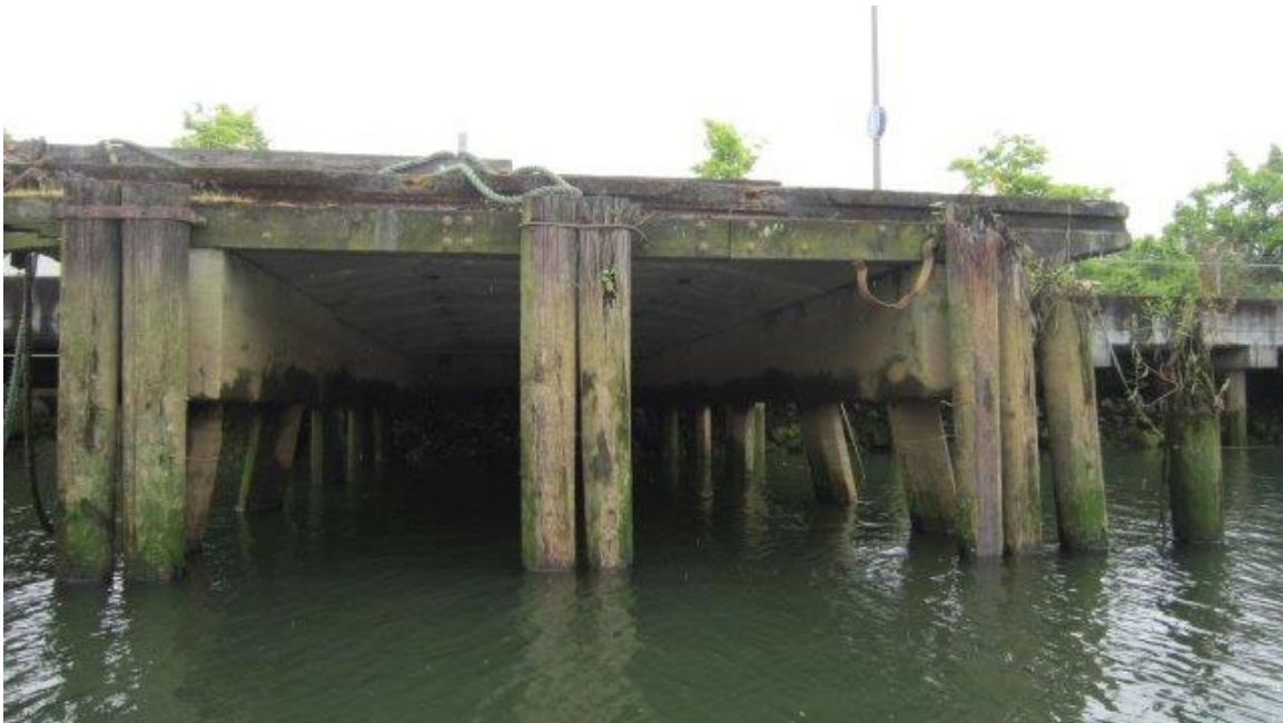
Photo ST05-22: Pier 5
