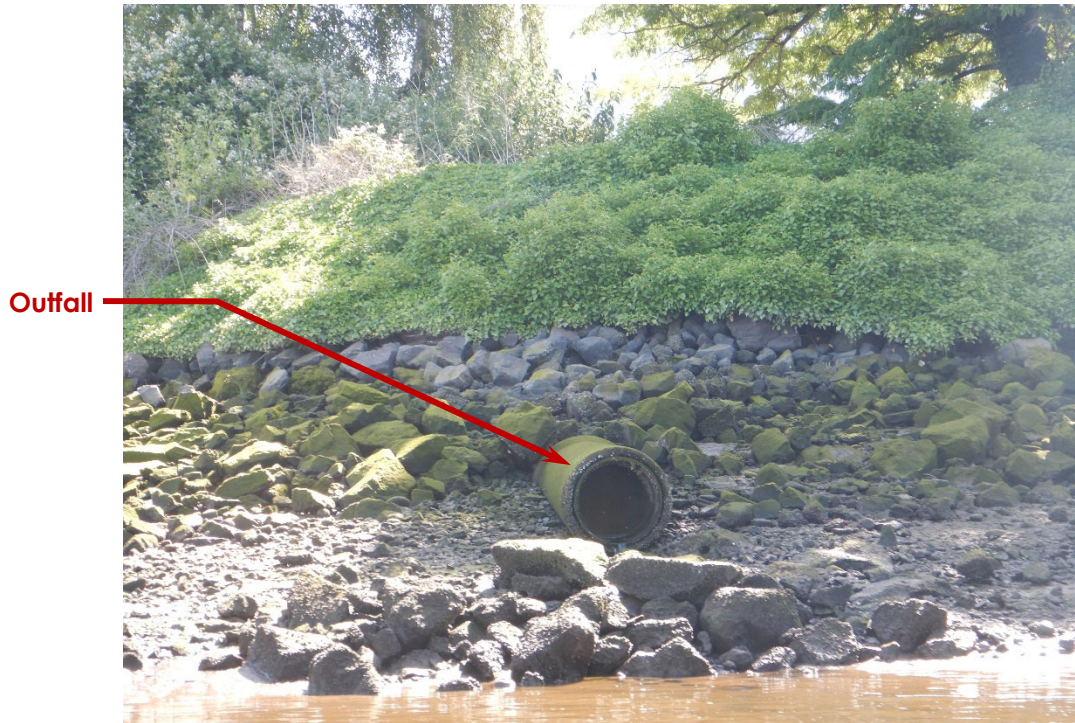
Photo 2087-01: Outfall (Looking East)
