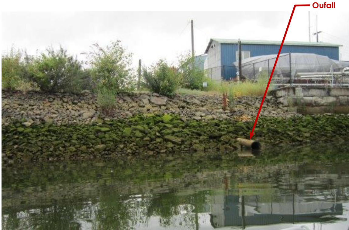
Photo 2214-01: Outfall (Looking West)
