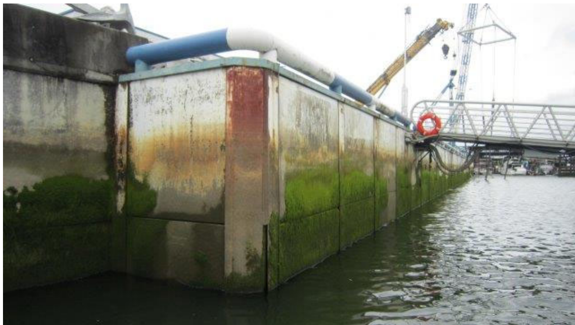
Photo ST12-10: H-Pile Bulkhead (Looking North)
