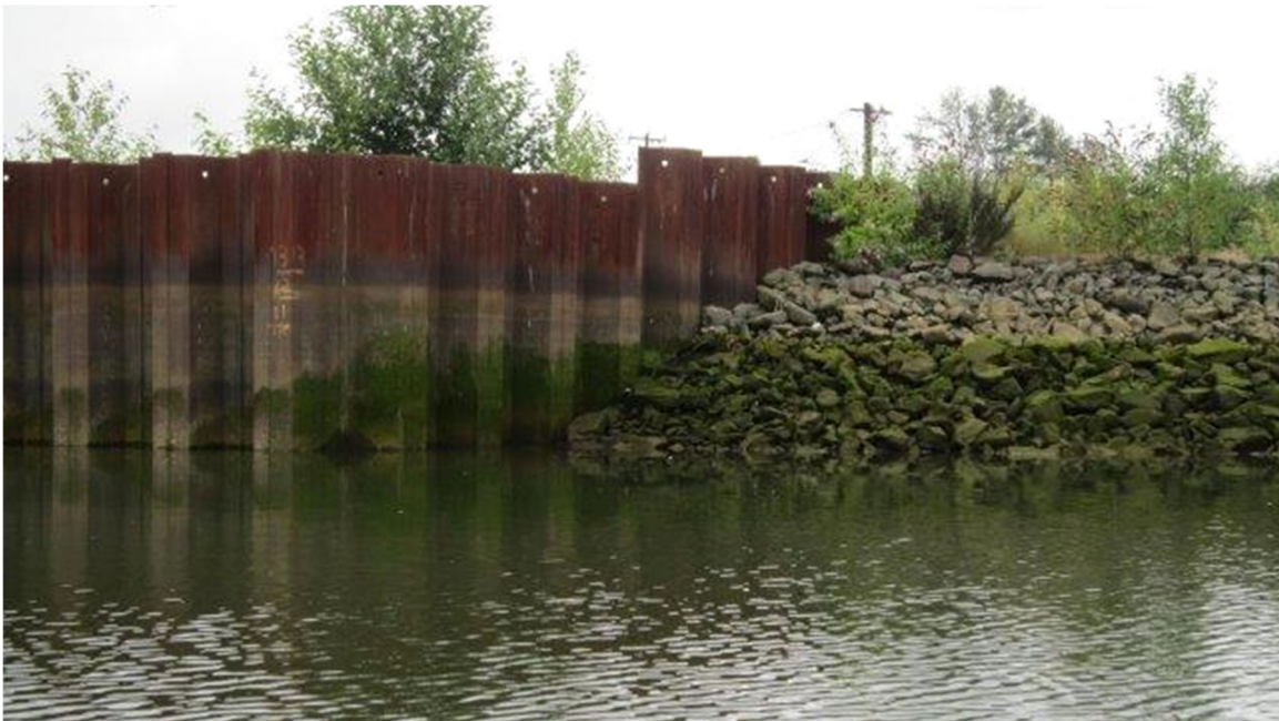
Photo ST19-04: North Return Wall (Looking West)
