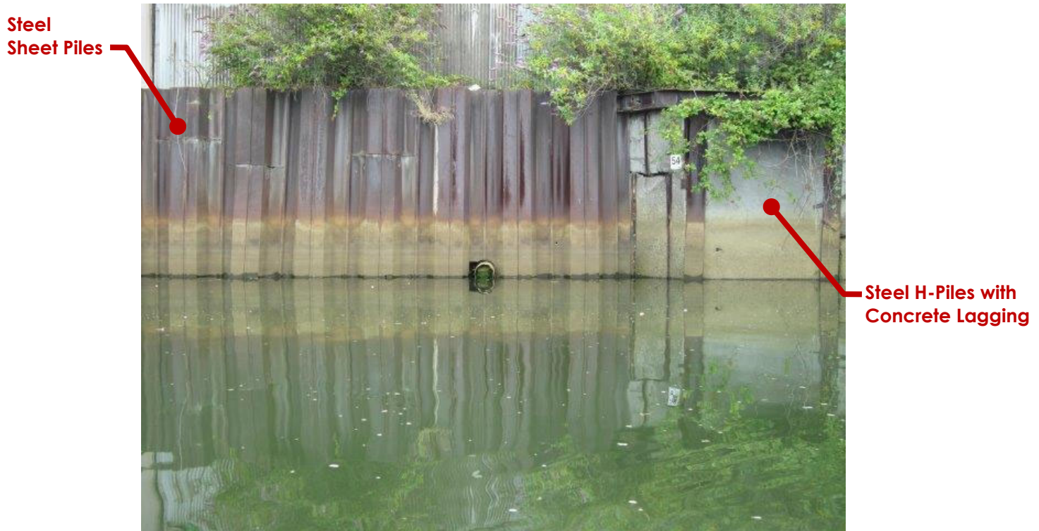
Photo ST03-06: Sheet Piles (south end)
