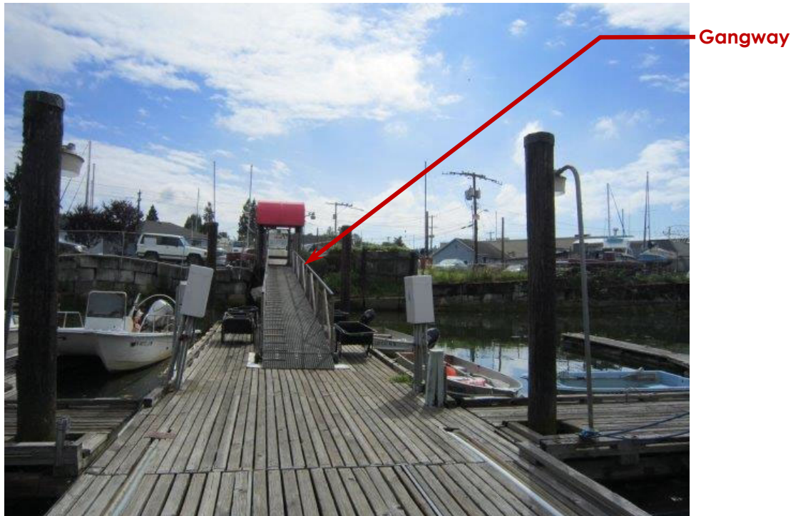
Photo ST20-09: Gangway and Walkway (Looking West)
