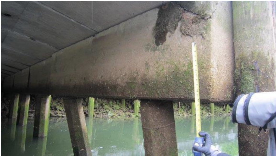
Photo ST05-03: Pier 1, East Side of West Pile Cap
