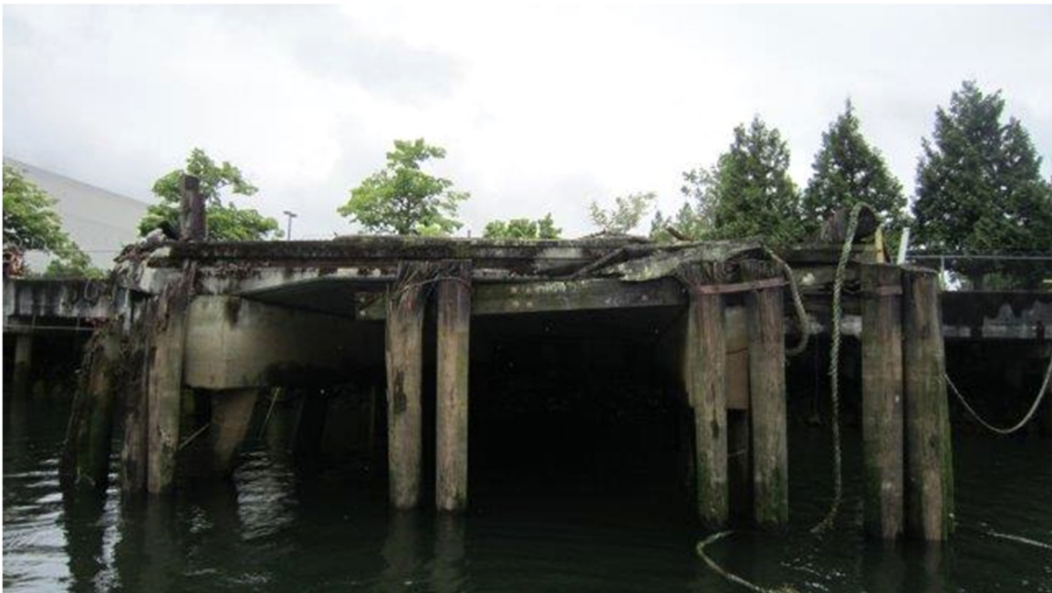
Photo ST05-26: Pier 6
