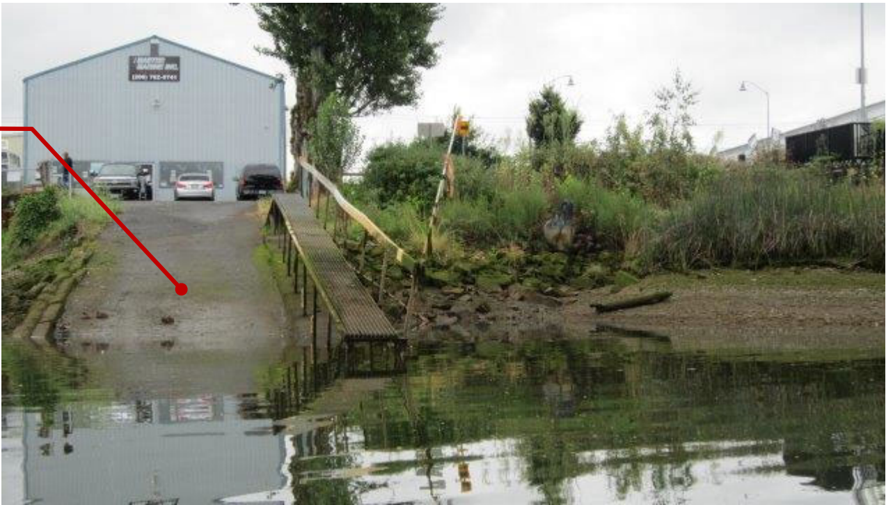
Photo ST20-08: Boat Ramp (Looking West)
