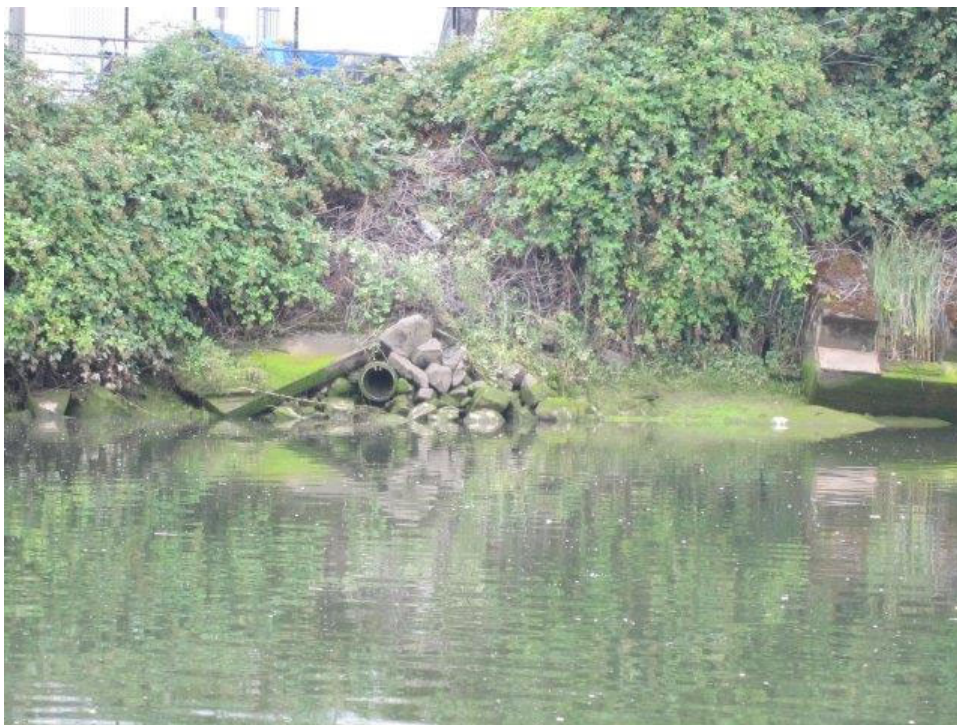
Photo 2092-02: Outfall (Looking East)
