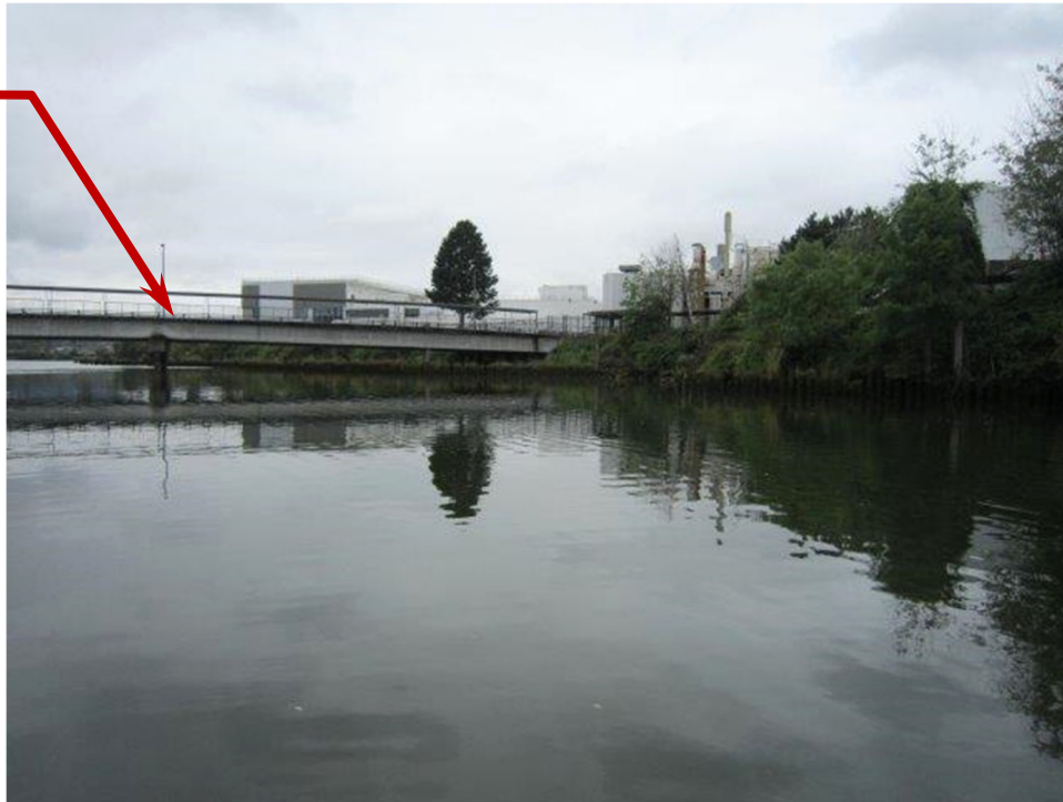
Photo ST07-15: Groins and Embankment South of Bridge (Looking Northeast)
