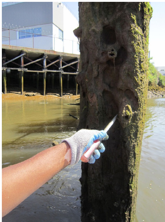
Photo ST07-10: End Pile
