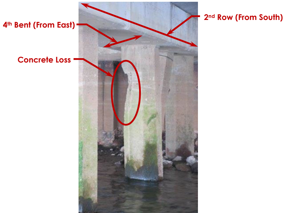
Photo ST16-08: Concrete Pile
