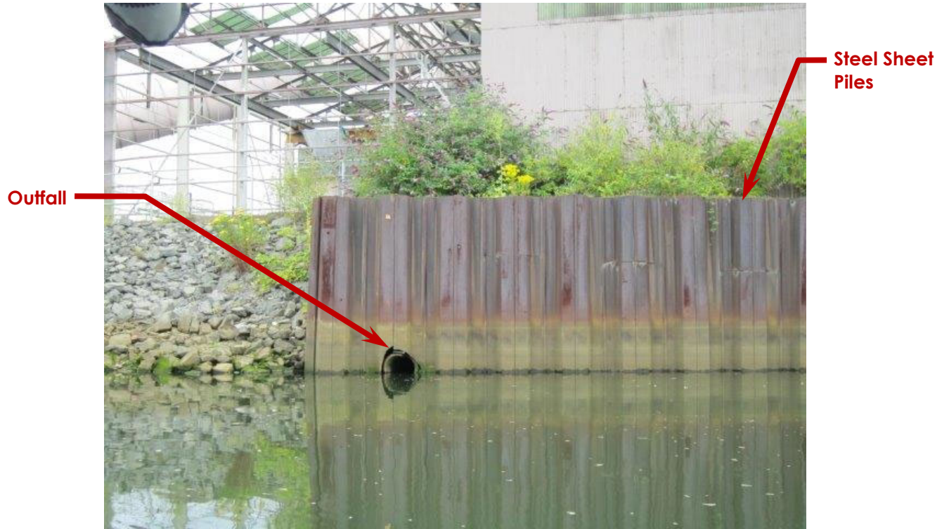
Photo ST03-05: Sheet Pile Bulkhead (north end)
