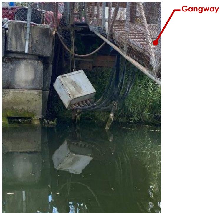
Photo ST20-10: Services (Looking West)
