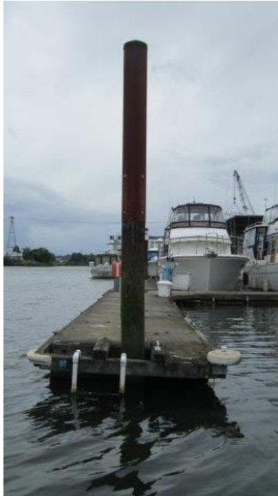
Photo ST15-07: Outboard Float (Looking South)
