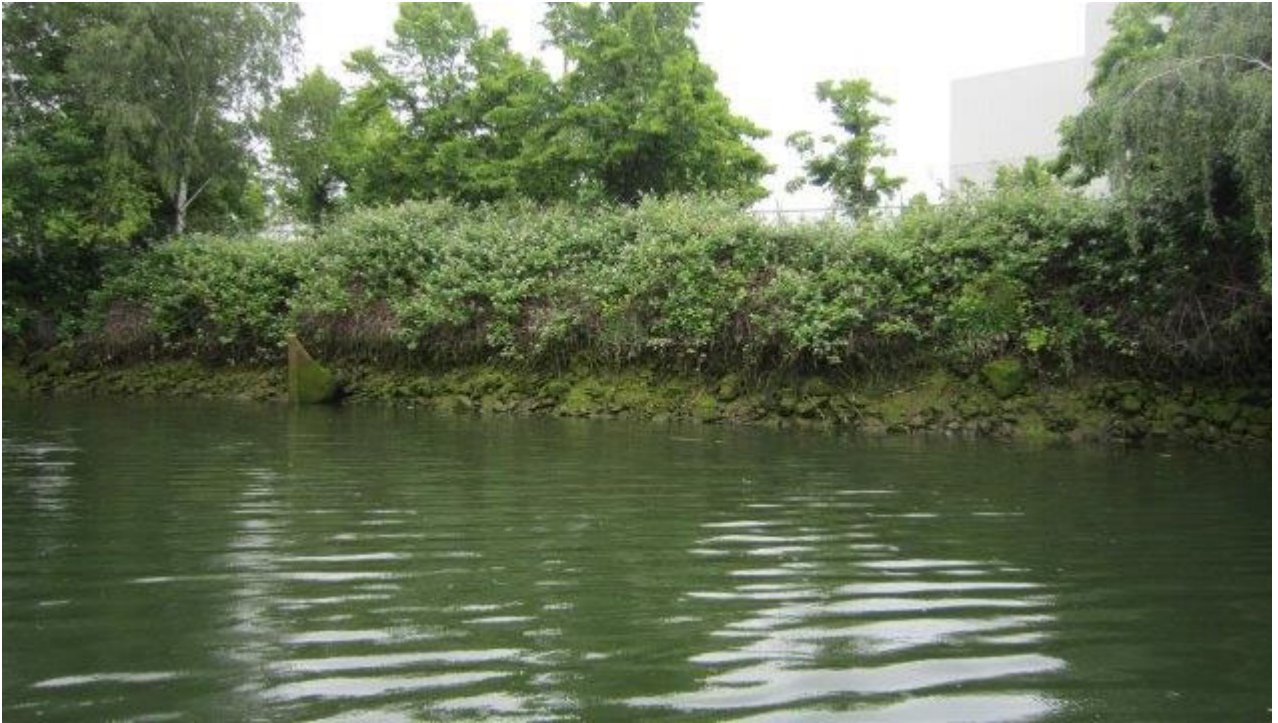
Photo 2081-01: Outfall (Looking North)
