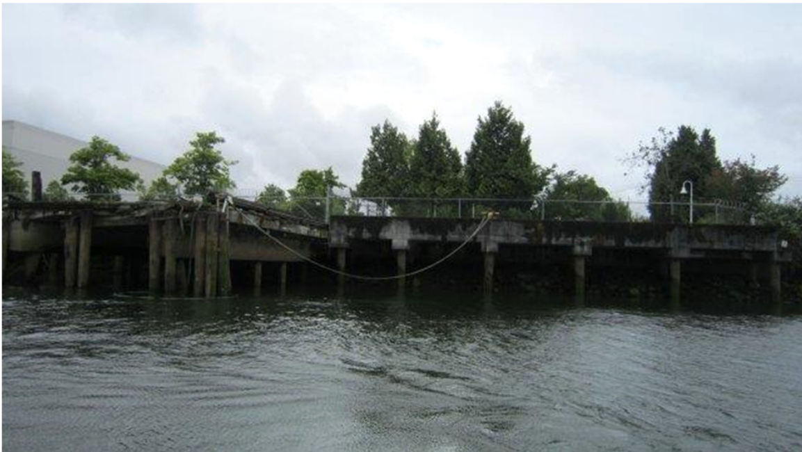
Photo ST05-30: Wharf West of Pier 6
