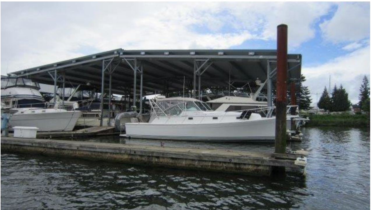
Photo ST15-06: Outboard Float (Looking West)
