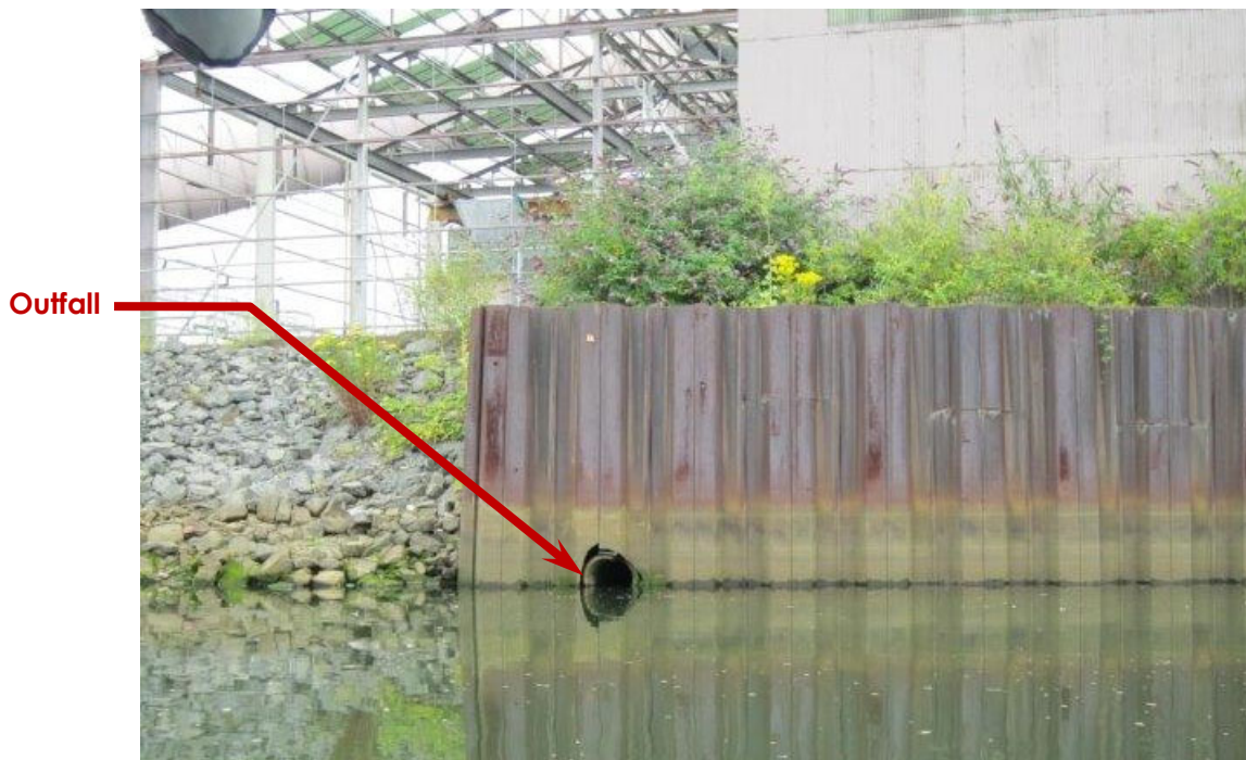
2072-02: Concrete Outfall at High Tide
