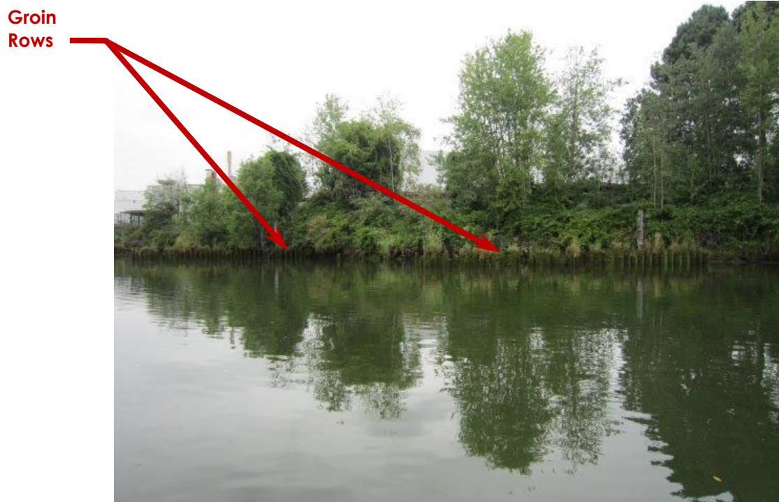
Photo ST07-14: Groins and Embankment South of Bridge
