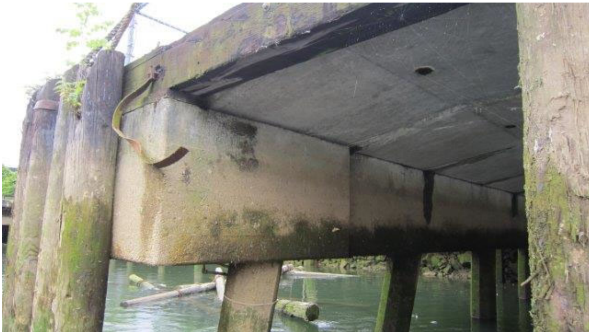
Photo ST05-16: Pier 3, East Pile Cap
