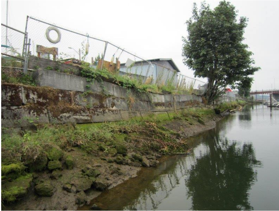
Photo ST20-03: Retaining Wall (Looking North)
