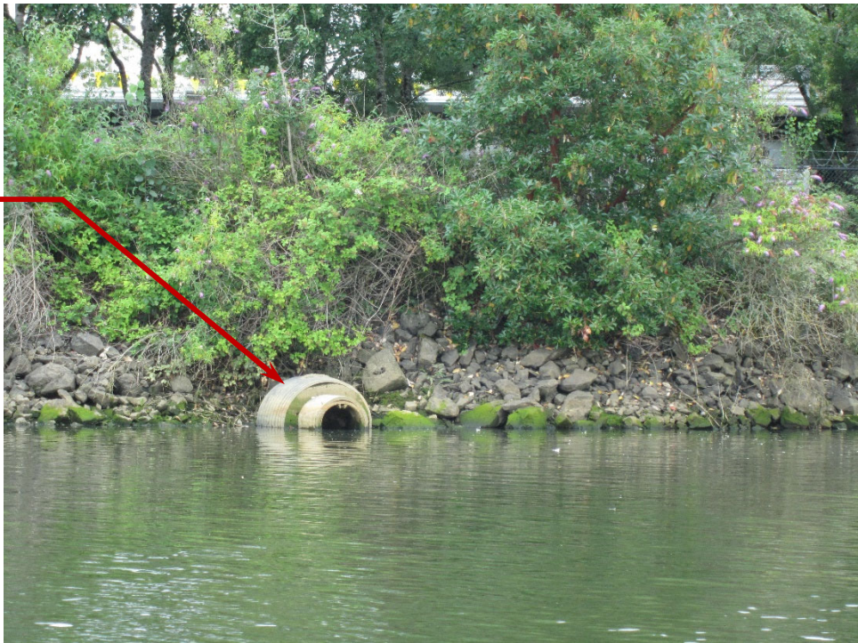
Photo 2089-02: Outfall (Looking East)
