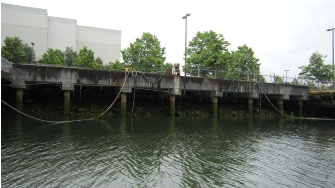
Photo ST05-18: Wharf Between Pier 3 and Pier 4
