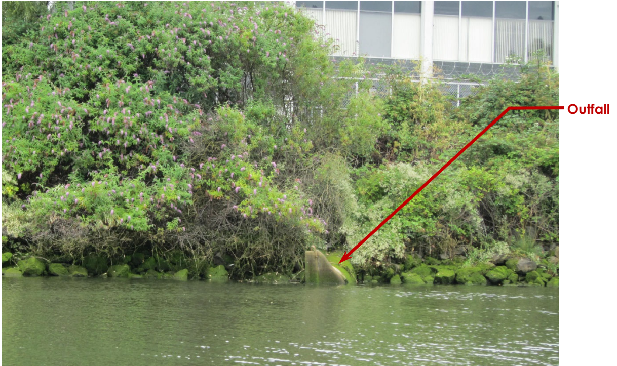
Photo 2090-01: Outfall (Looking East)
