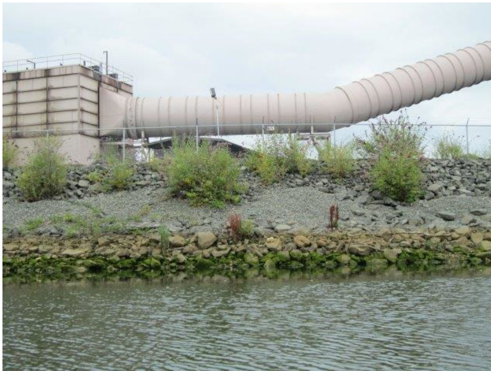
Photo ST03-04: Riprap Section
