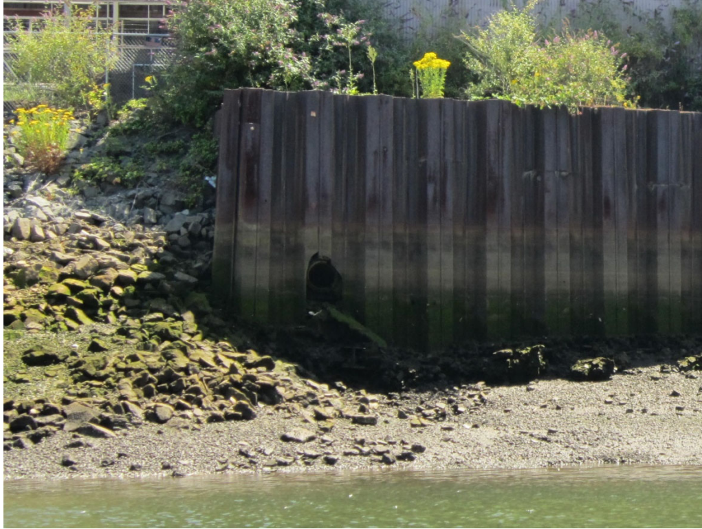
2072-03: Concrete Outfall at Low tide
