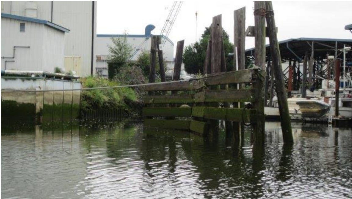
Photo ST12-15: Breakwater
