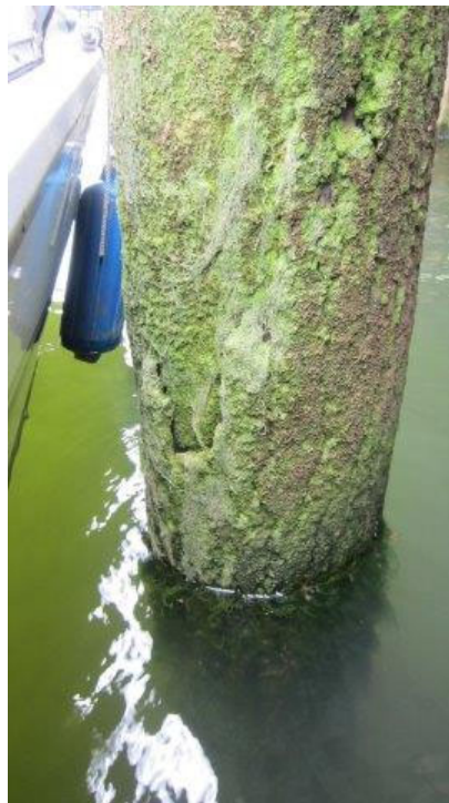
Photo ST16-04: Fender Pile
