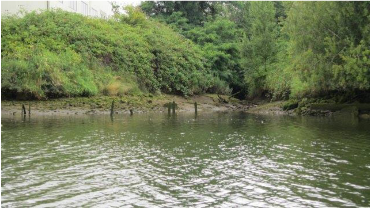
Photo ST17-01: Pile Field
