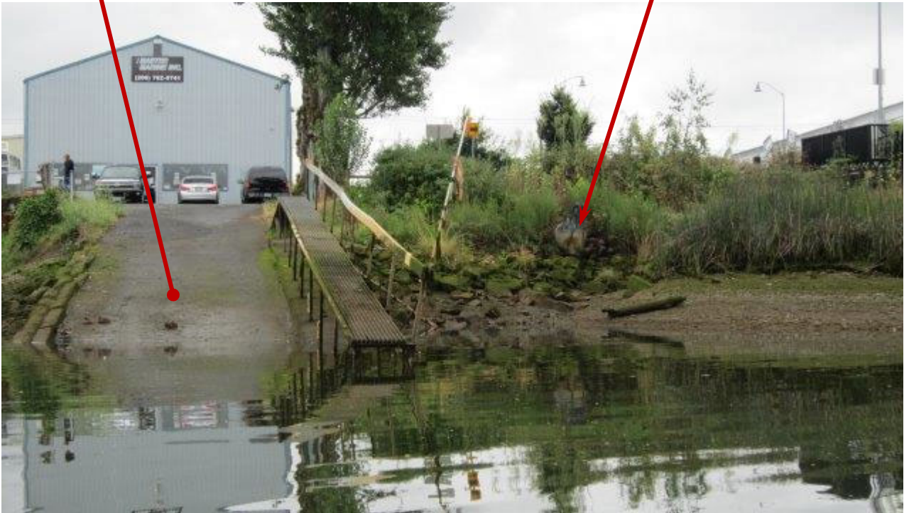
Photo 2215-01: Outfall (Looking West)
