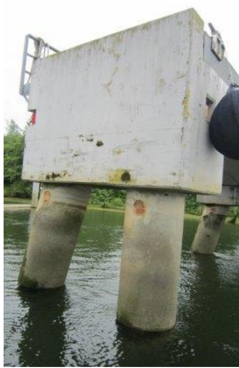
Photo ST12-03: East End Piles and Caps of South Finger Pier
