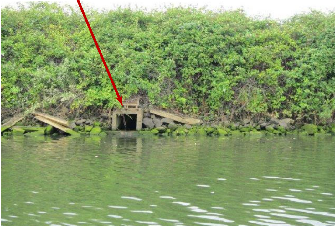
2073-01: Outfall Box at High Tide
