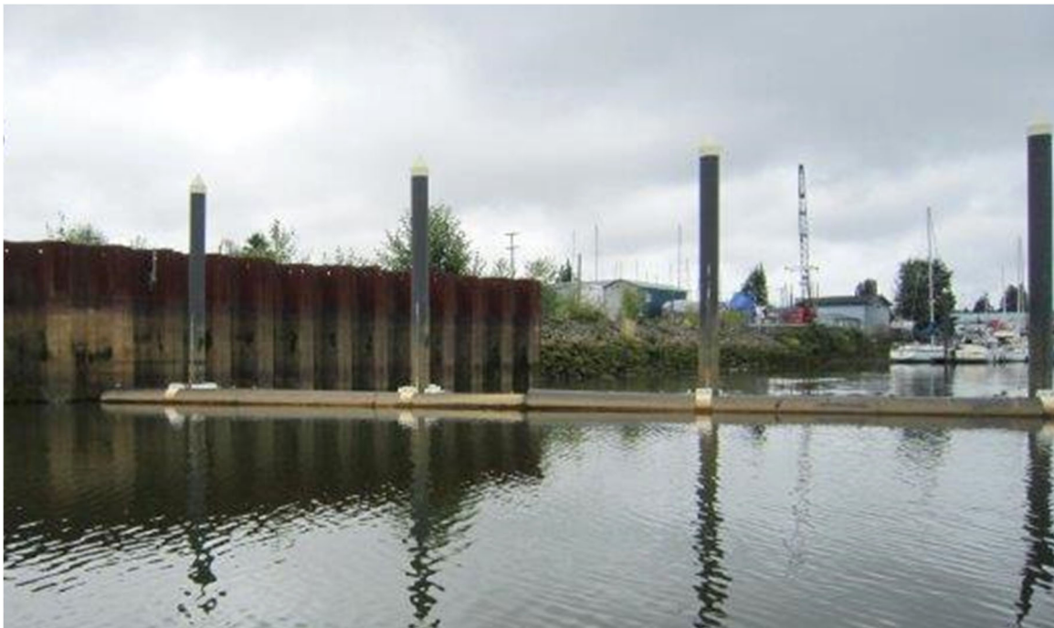
Photo ST19-02: Debris Deflector Float (Looking Northwest)
