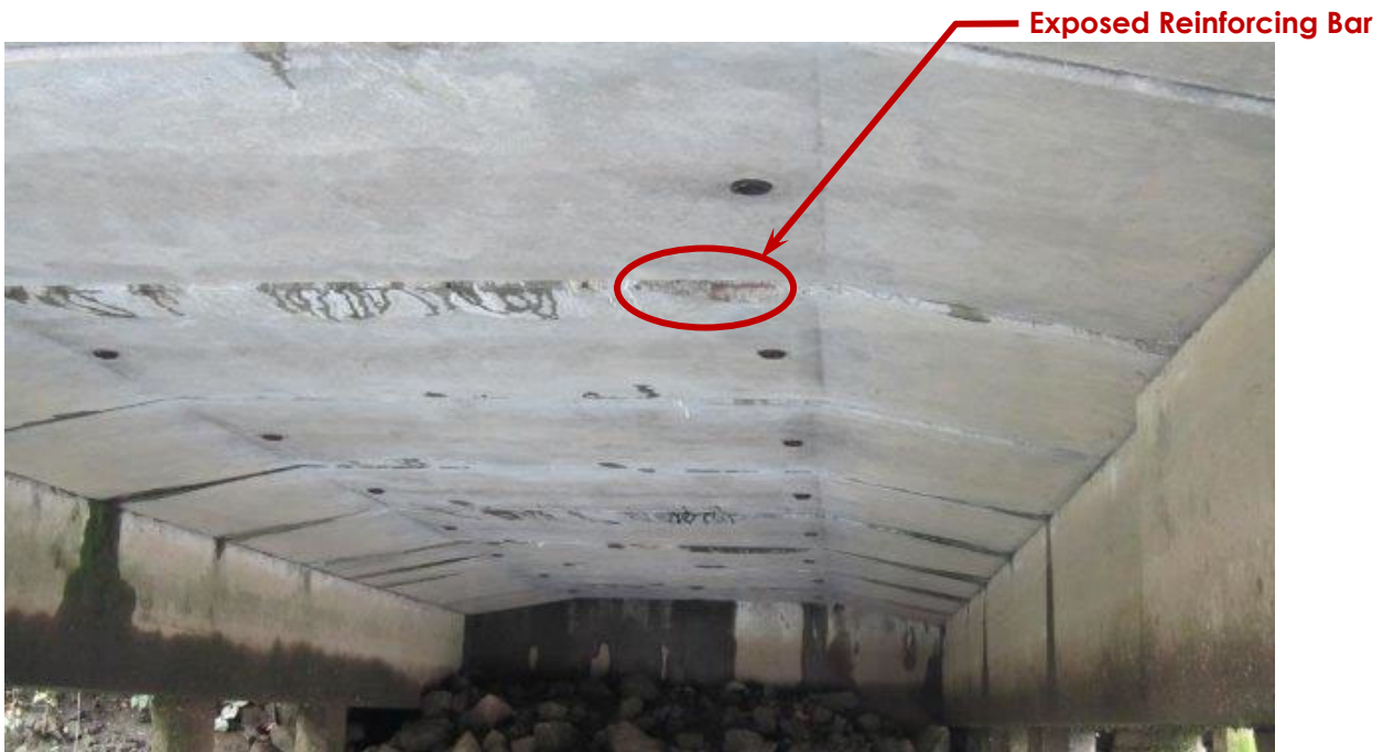
Photo ST05-06: Pier 1, Pier Deck Soffit
