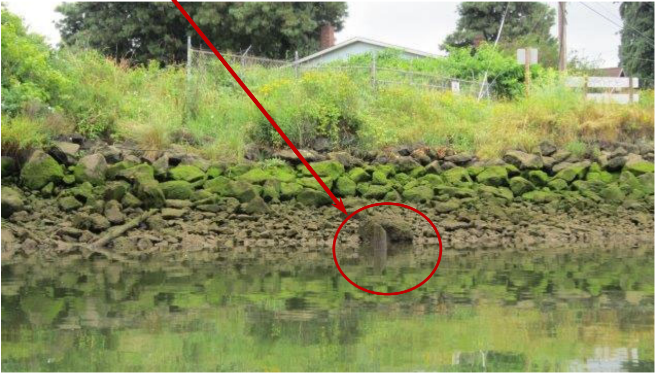
Photo ST21-01: Southmost Pile Field
