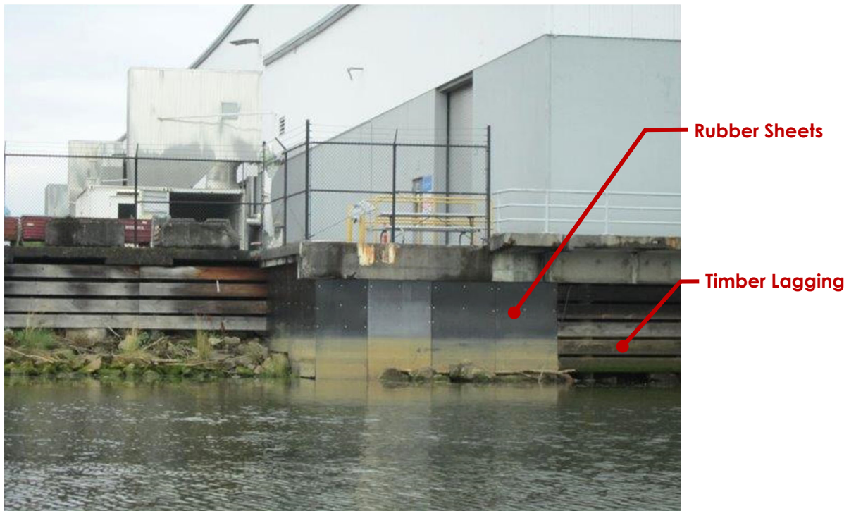
Photo ST38-02: North End of Building
