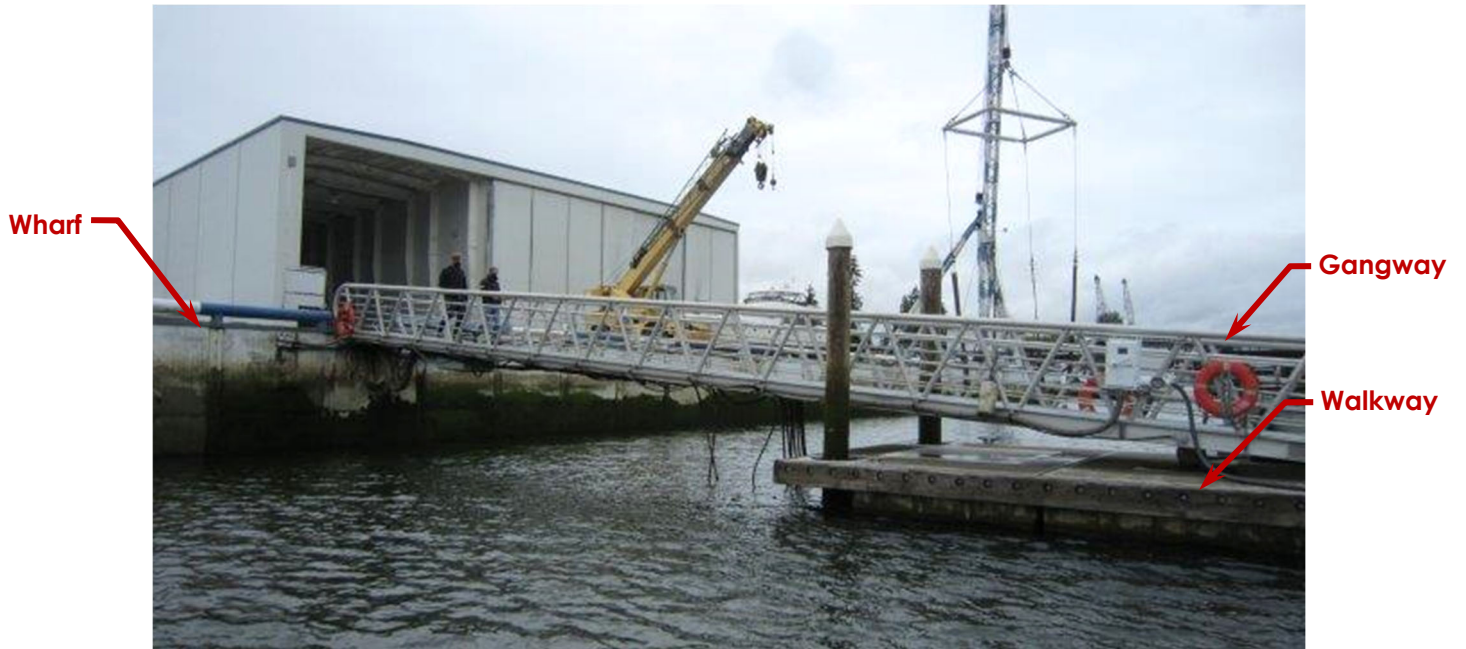
Photo ST12-06: Floating Dock Access Way (Looking North)
