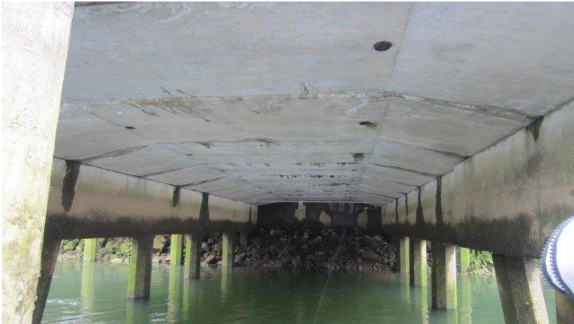
Photo ST05-17: Pier 3, Pier Deck Soffit
