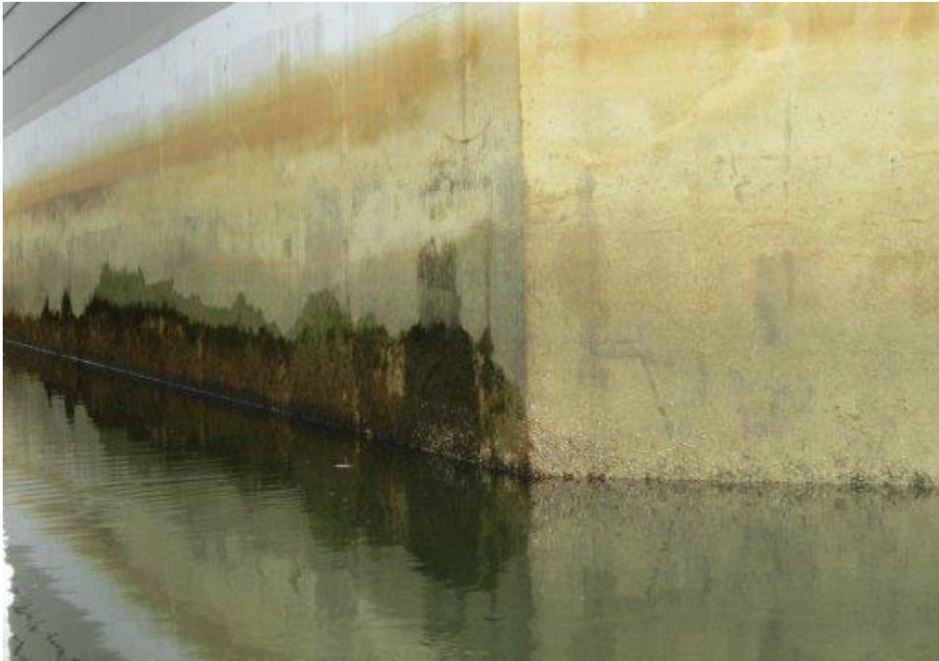
ST02-07: West Bascule Pier (southeast side)
