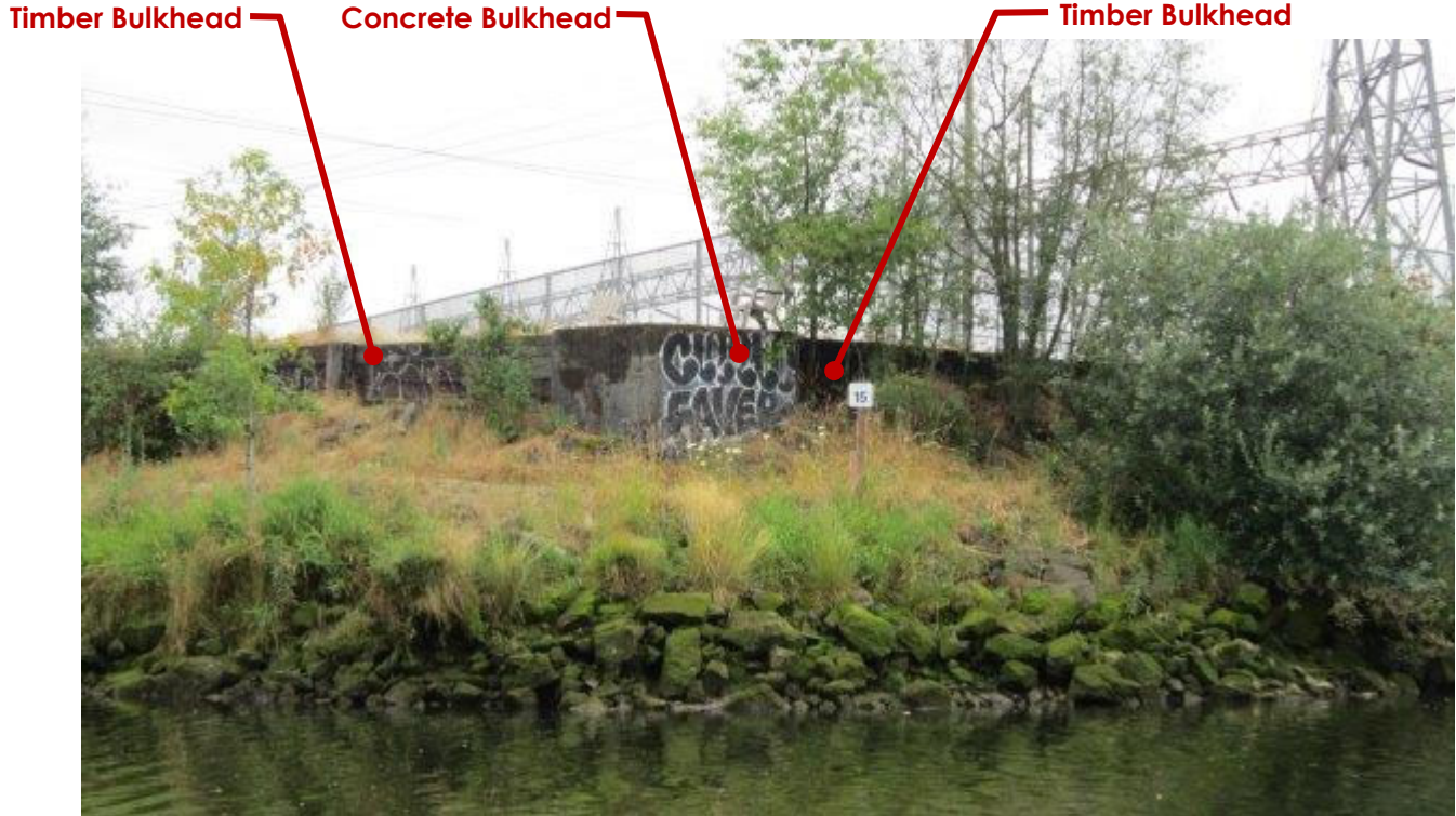
Photo ST06-01: West Shoreline Bulkhead South End
