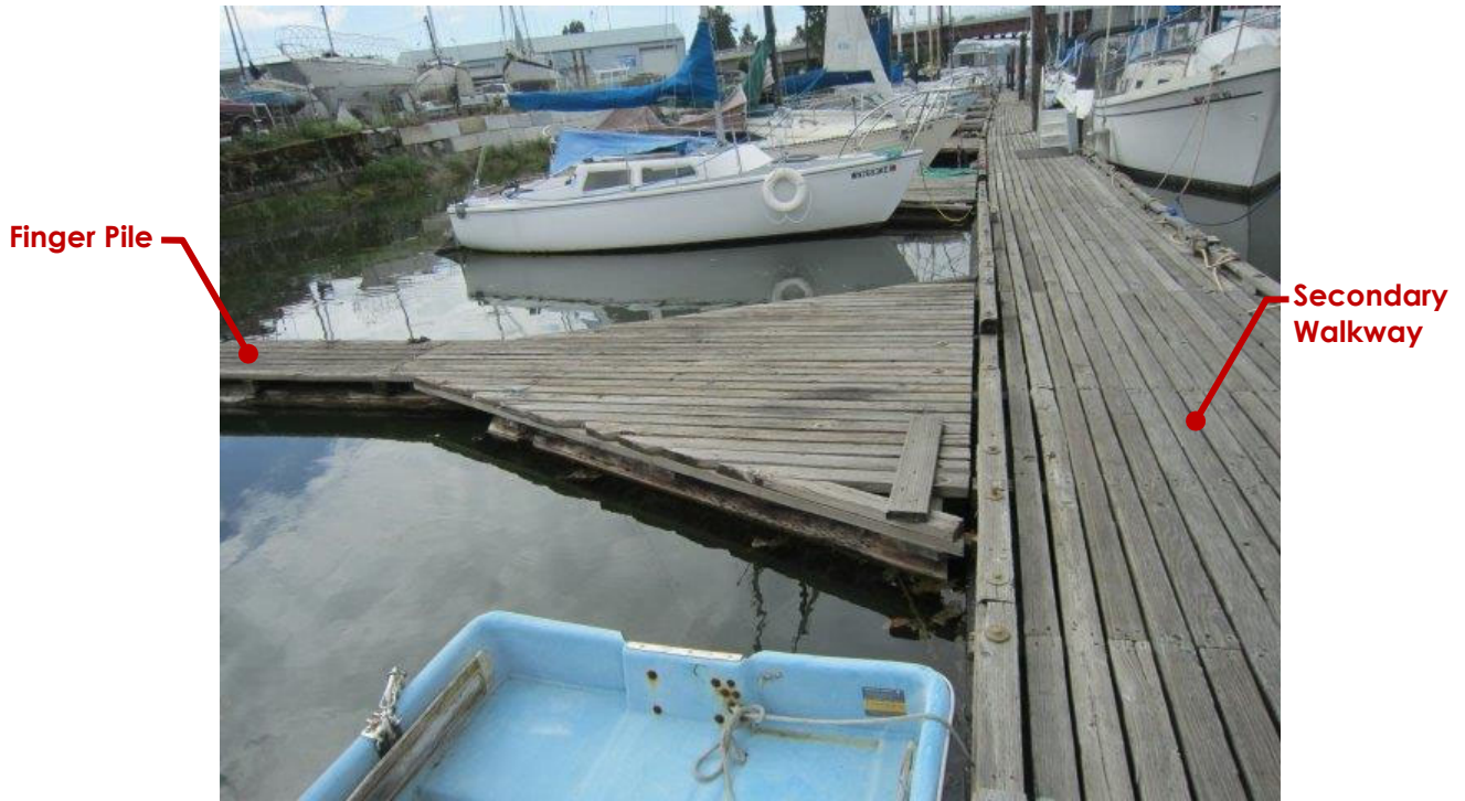
Photo ST20-13: West Secondary Walkway (Looking North)
