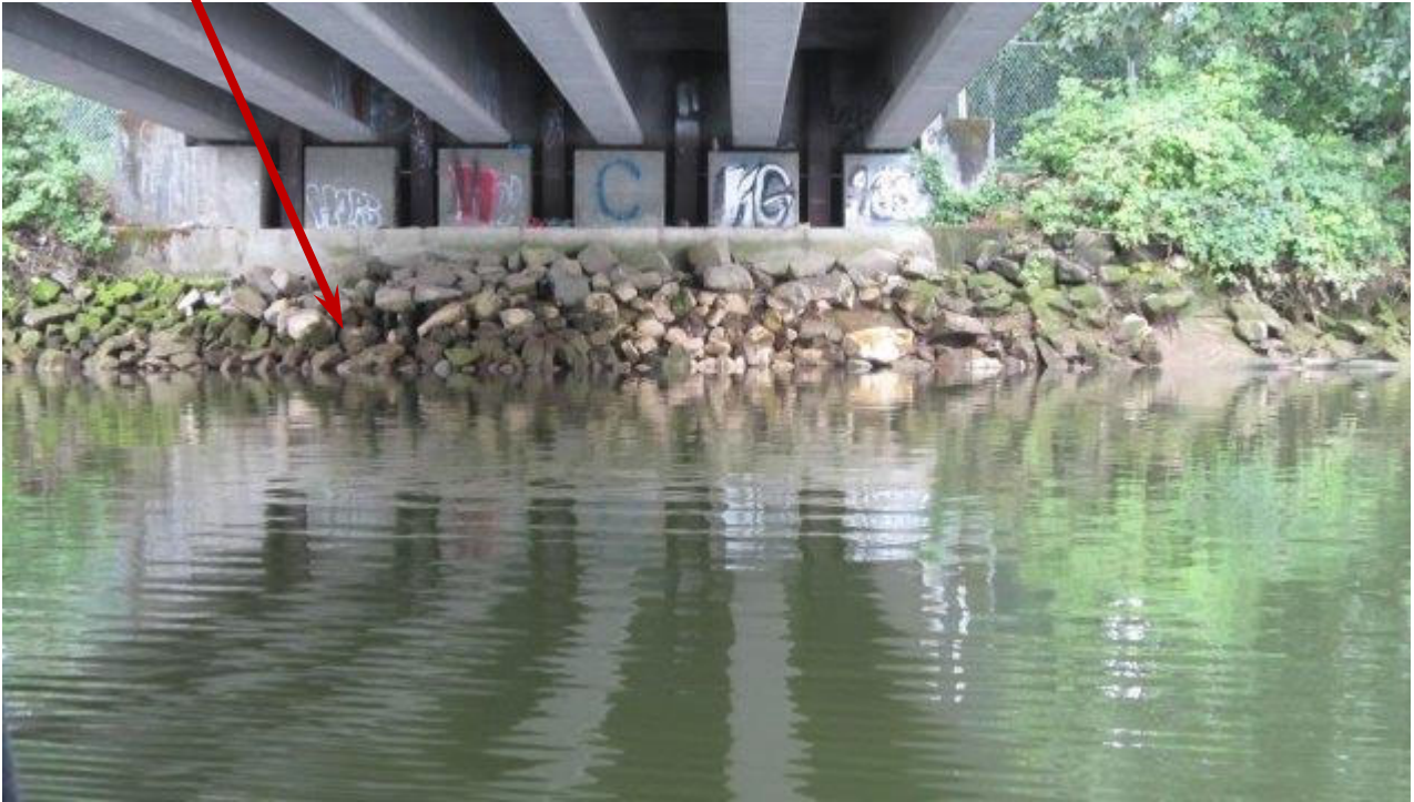
Photo ST08-03: West Abutment
