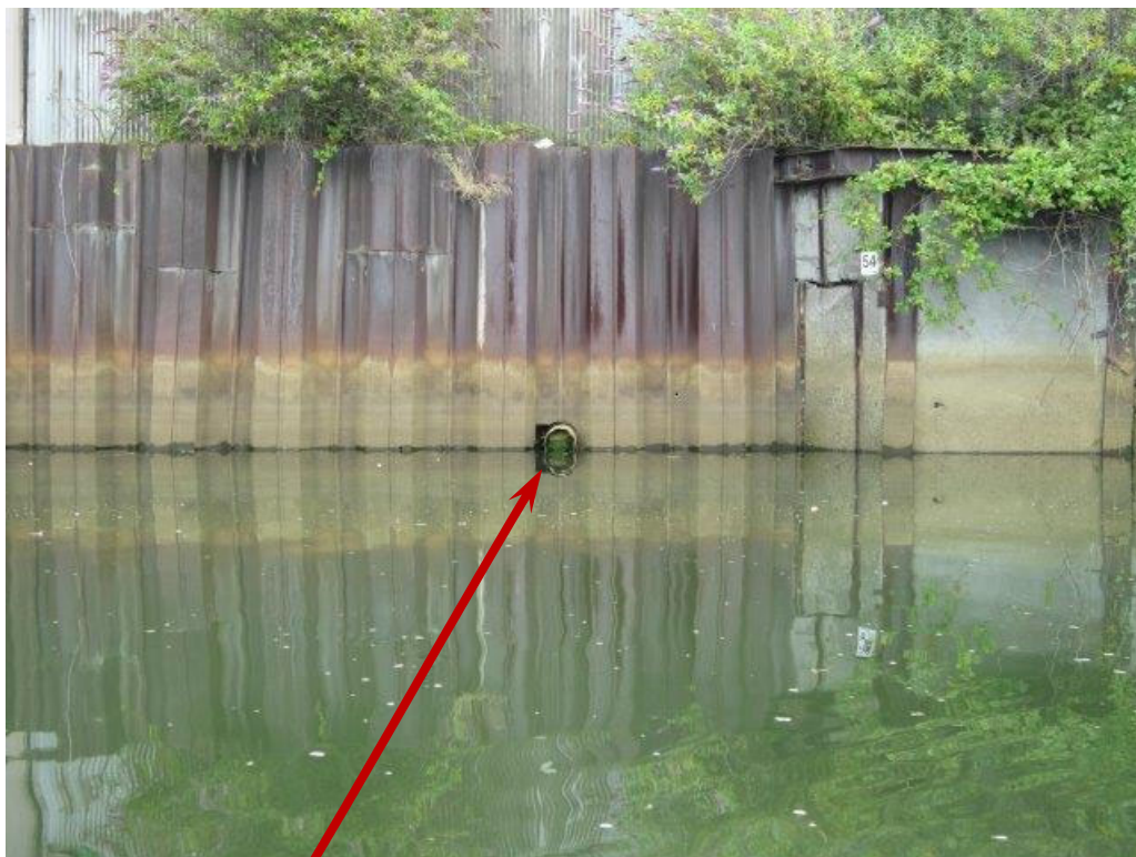
Outfall 2063-02: Outfall at High Tide
