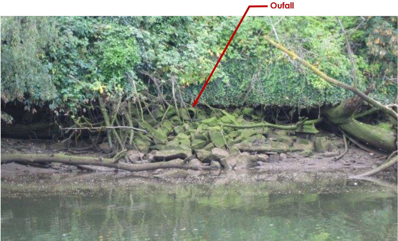
Photo SP3-01: Outfall (Looking West)
