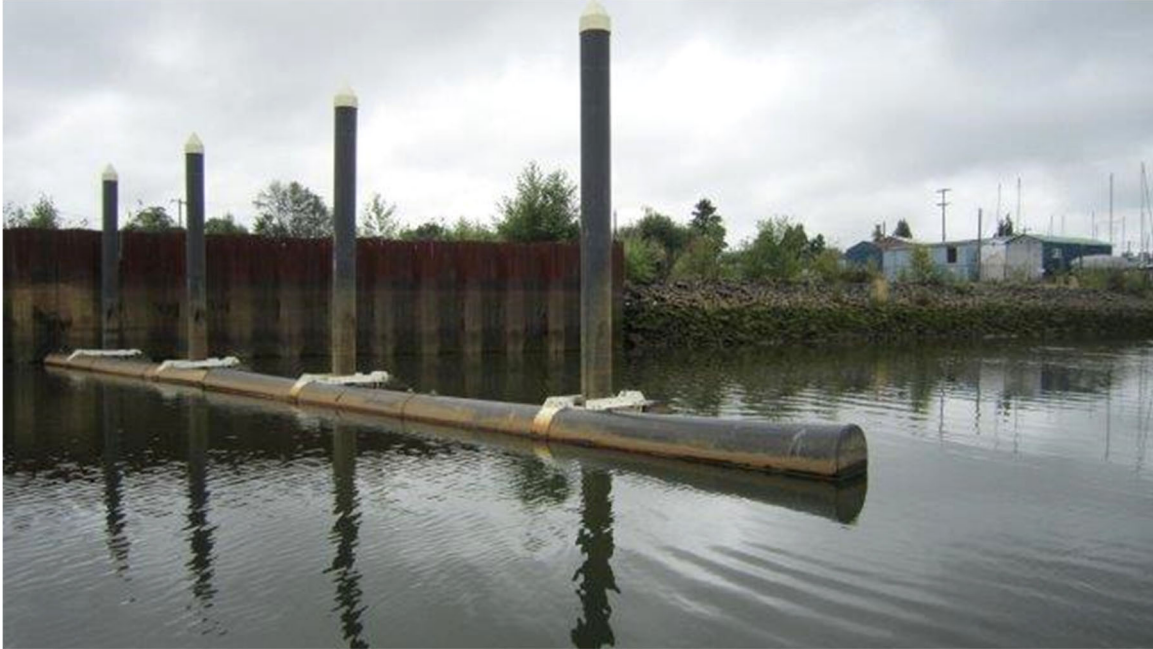
Photo ST19-03: Debris Deflector Float (Looking Northwest)
