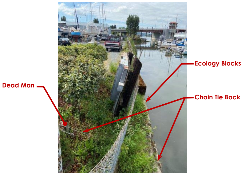
Photo ST20-04: Retaining Wall Bulkhead (Looking North)
