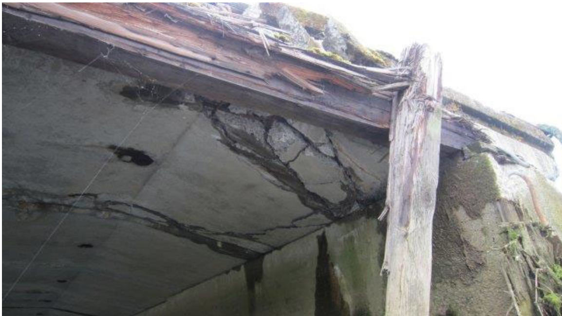
Photo ST05-12: Pier 2, Top West Corner of 1 st Deck Panel
