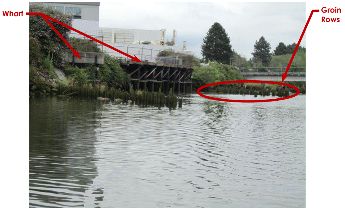
Photo ST07-02: Wharfs (Looking East)
