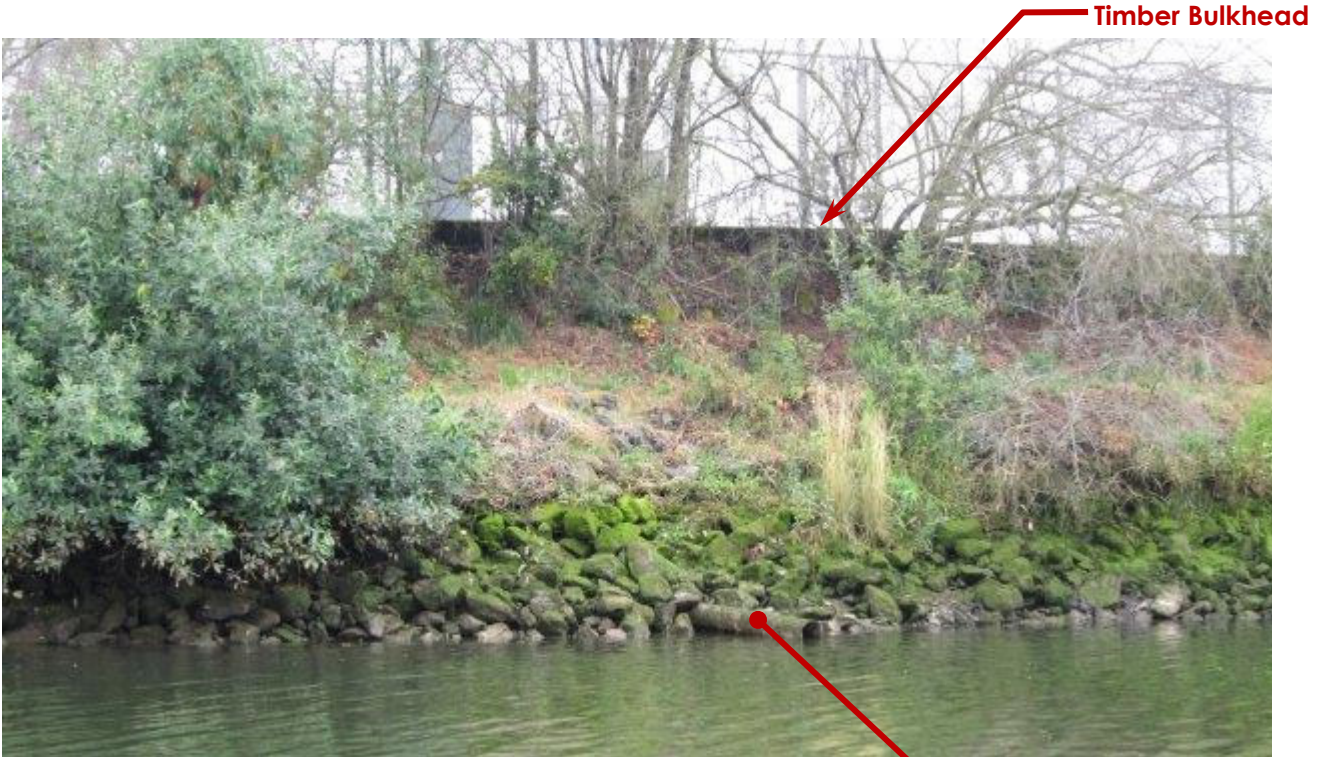
Photo ST06-02: West Shoreline Bulkhead
