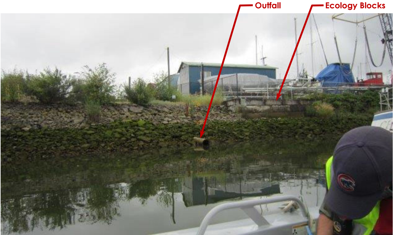
Photo ST20-01: Retaining Wall Bulkhead (Looking Northwest)
