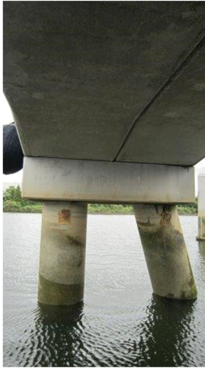
Photo ST12-05: Pile Cap and Pier Decks (Looking West)
