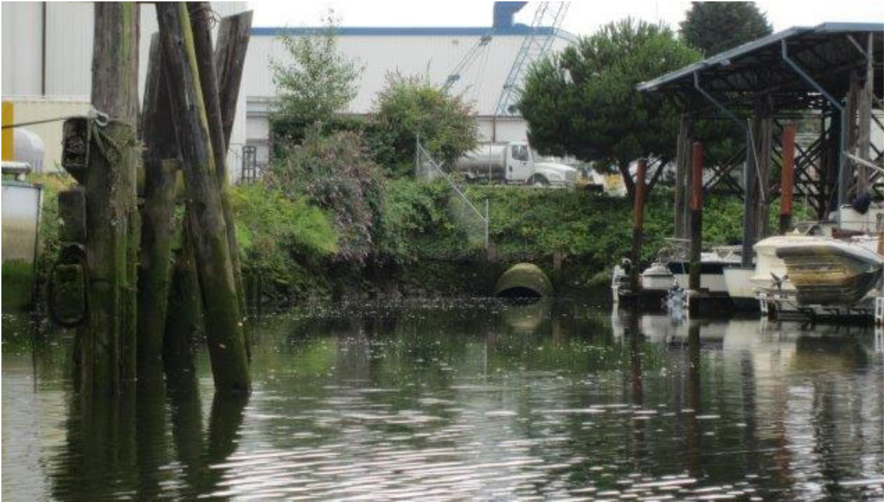
Photo 2100B-01: Outfall at High Tide Level
