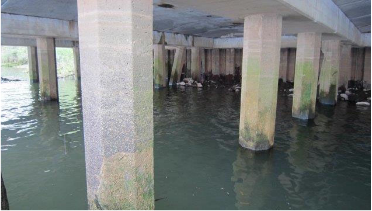
Photo ST16-07: Concrete Piles (Looking Southwest)
