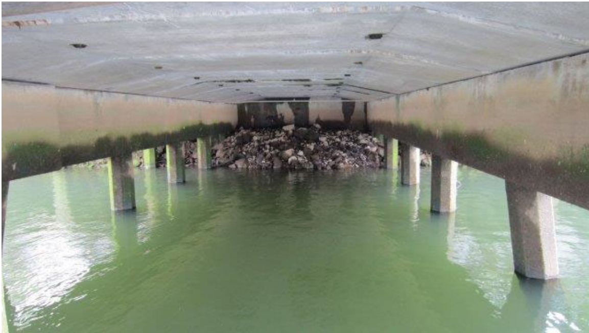
Photo ST05-29: Pier 6, Pier Deck Soffit
