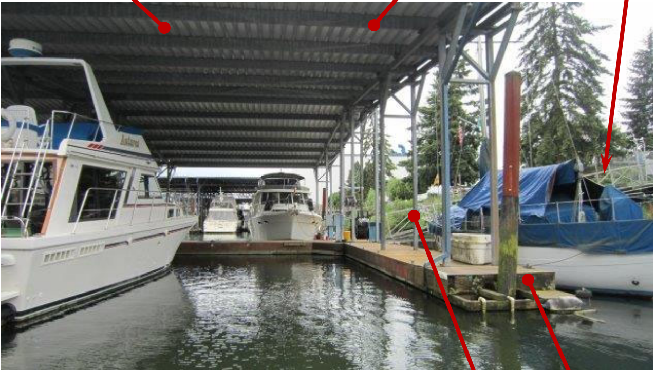
Photo ST15-02: Floats (Looking South)
