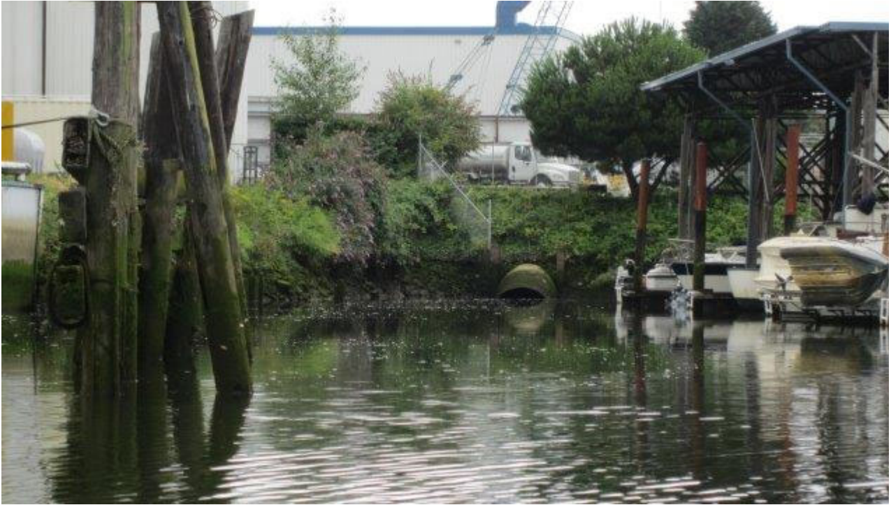
Photo ST13-03: View of Battered Piles (Looking West)
