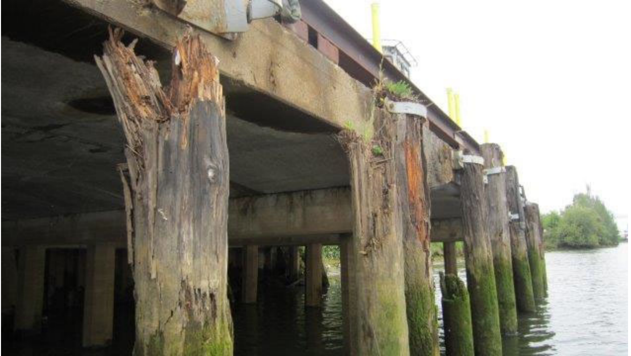
Photo ST16-03: Piers 3 and 4
