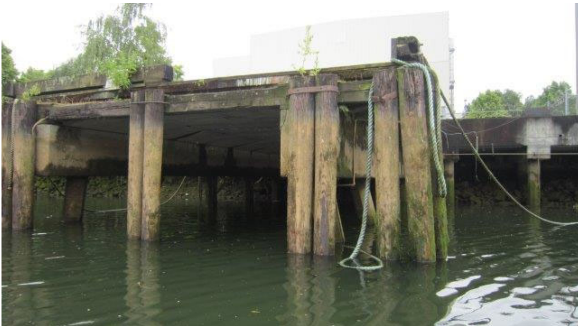
Photo ST05-02: Pier 1 (Looking South)
