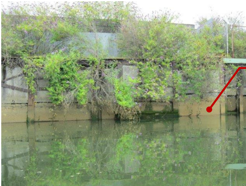
Photo ST03-08: H-Piles with Concrete Panels
