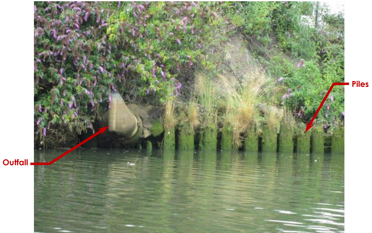
2077-01: Outfall at High Tide
