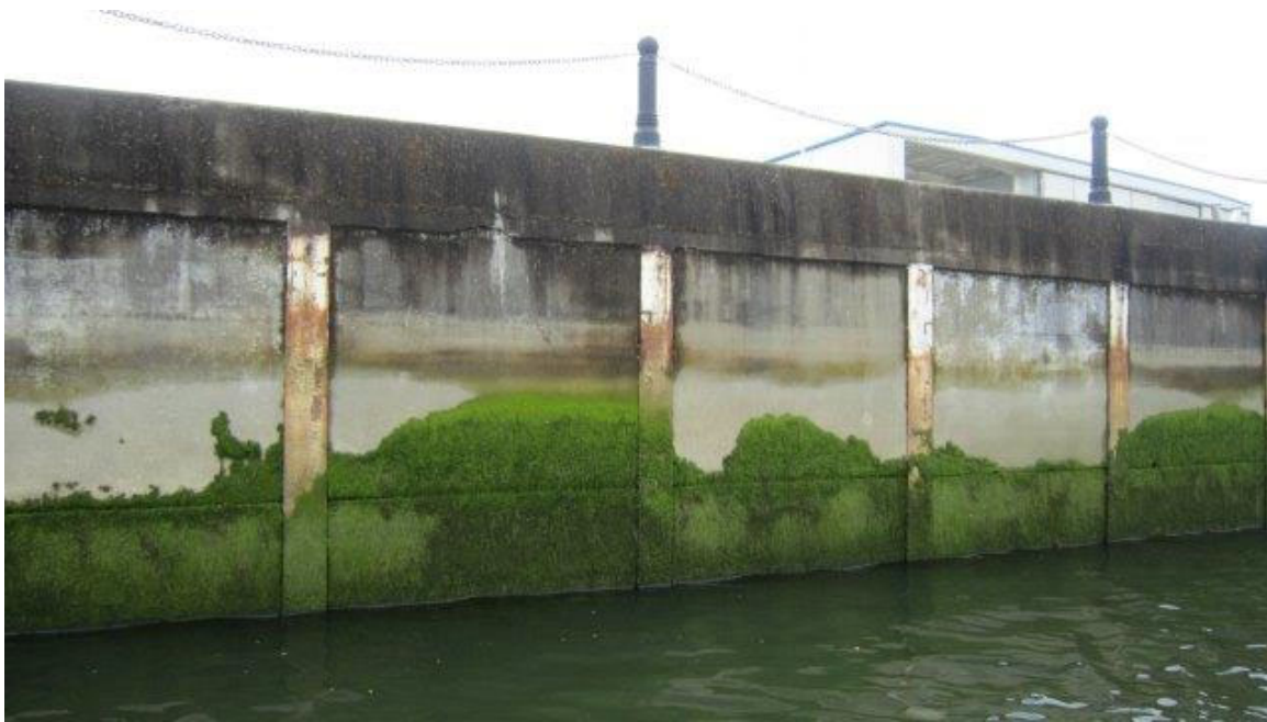
Photo ST12-11: Close Up of H-Pile Bulkhead
