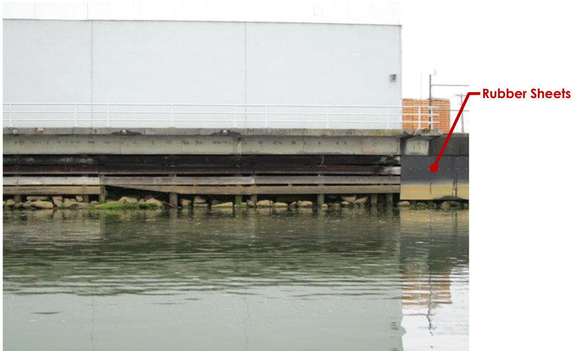
Photo ST38-05: South End of Building
