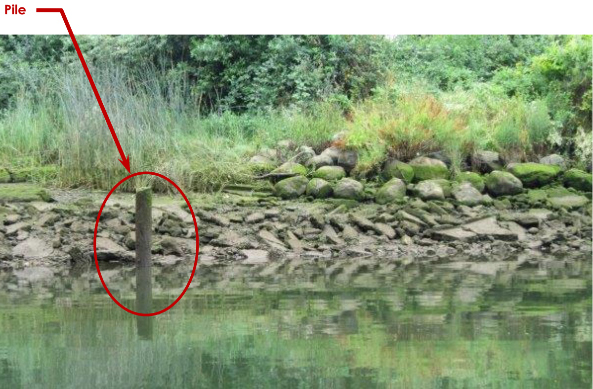
Photo ST21-02: Central Pile
