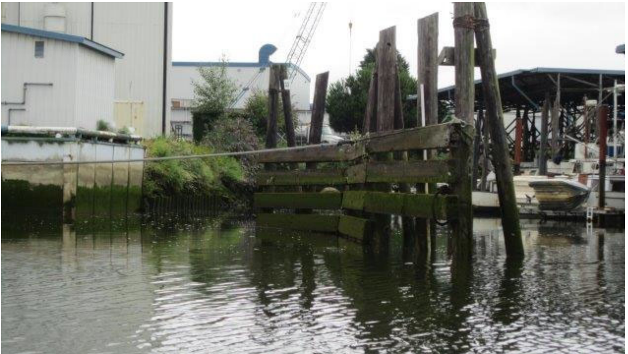
Photo ST13-02: Breakwater (Looking West)
