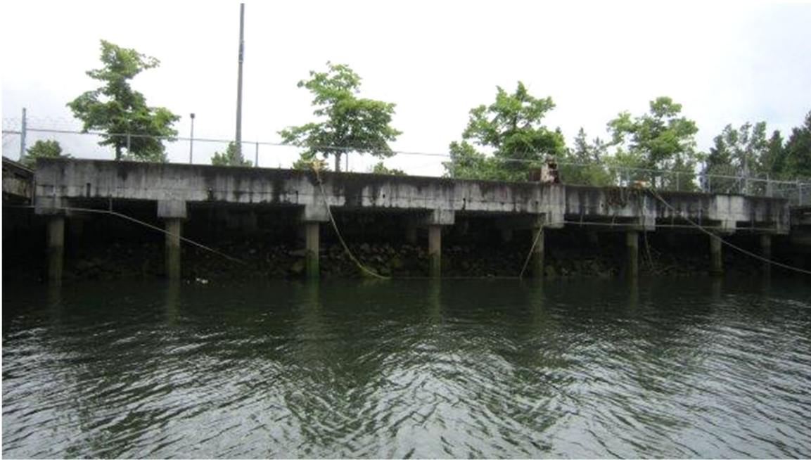
Photo ST05-25: Wharf Between Pier 5 and Pier 6
