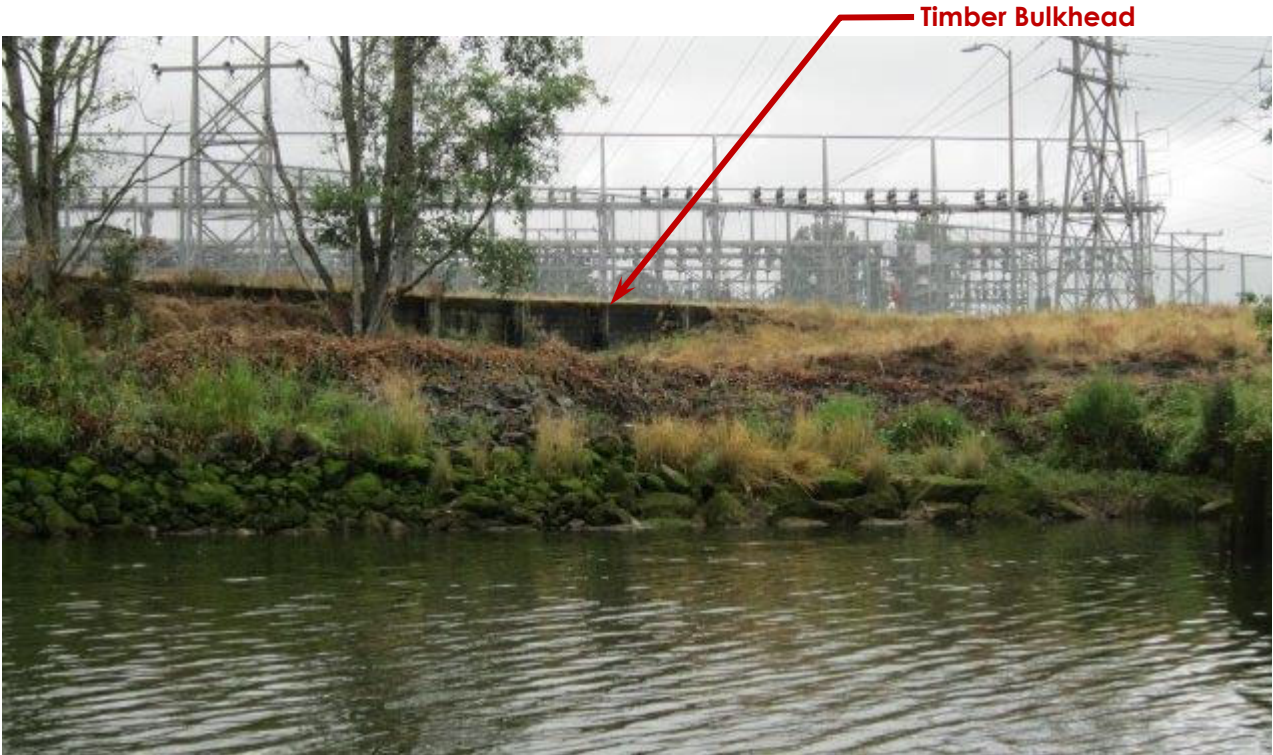
Photo ST06-03: West Shoreline Bulkhead
