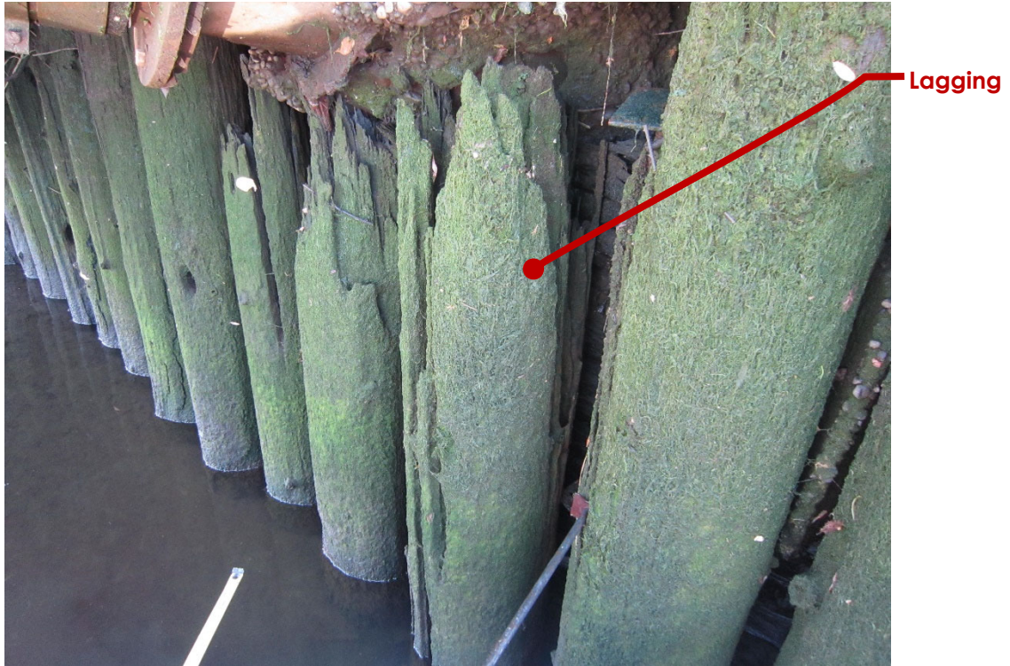
Photo ST03-25: Bulkhead Lagging Beneath Outfall
