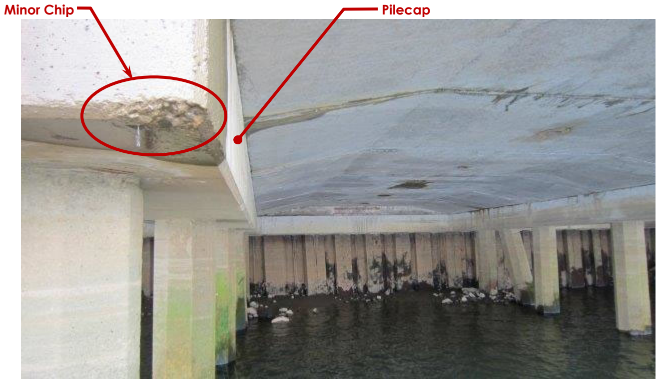
Photo ST16-15: Pier Deck Soffit
