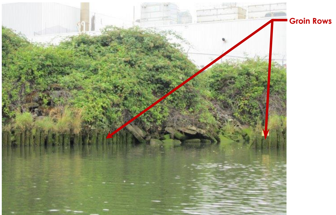
Photo ST07-12: Groins and Embankments North of Bridge
