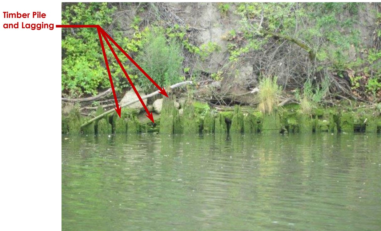
2077-02: Shoreline Timber Pile Bulkhead
