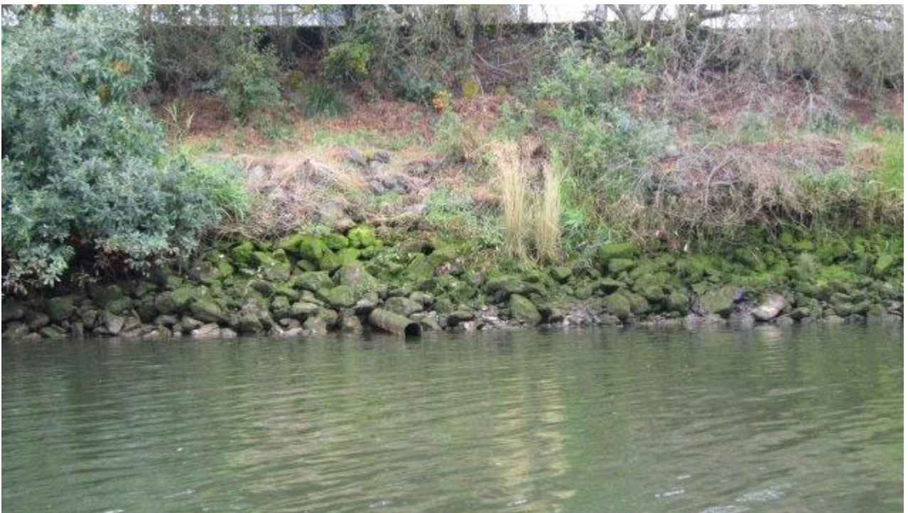
Photo 2098-02: Outfall (Looking West)
