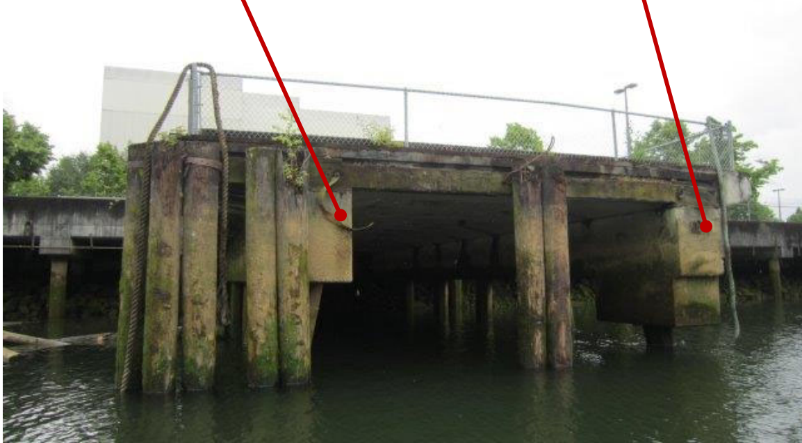
Photo ST05-15: Pier 3
