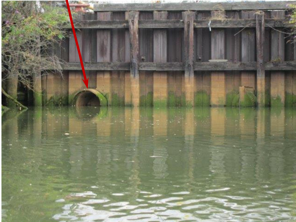
2062-02: Outfall at High Tide
