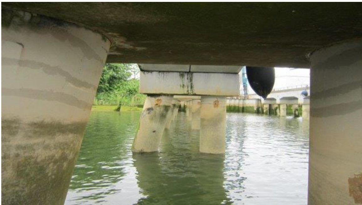
Photo ST12-04: South Pier Pile Rows (Looking West)
