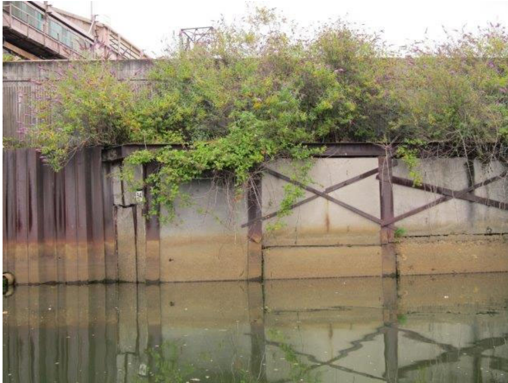
Photo ST03-07: H-Piles with Concrete Lagging (south end)
