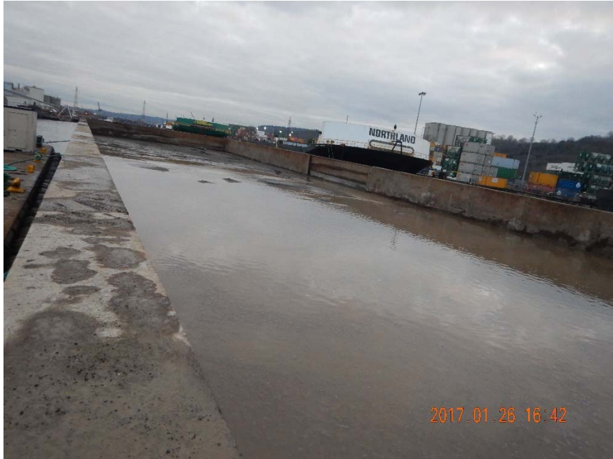
Photo 2-A: KP-3 barge after the last of the Sand ENR material has been placed.
