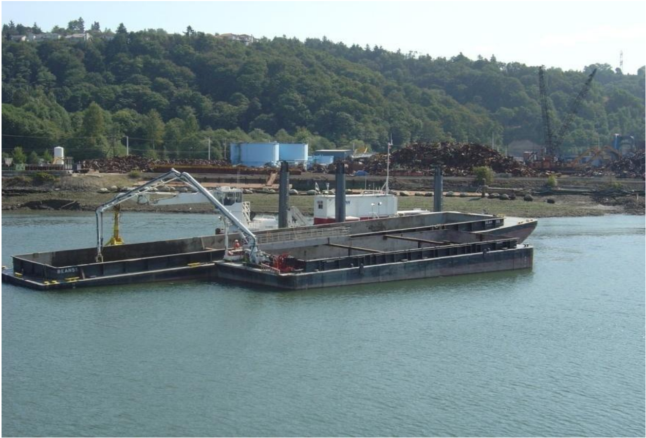
Figure 7-10 Sloping Drain Barge (Hylebos Waterway, Tacoma, WA)
