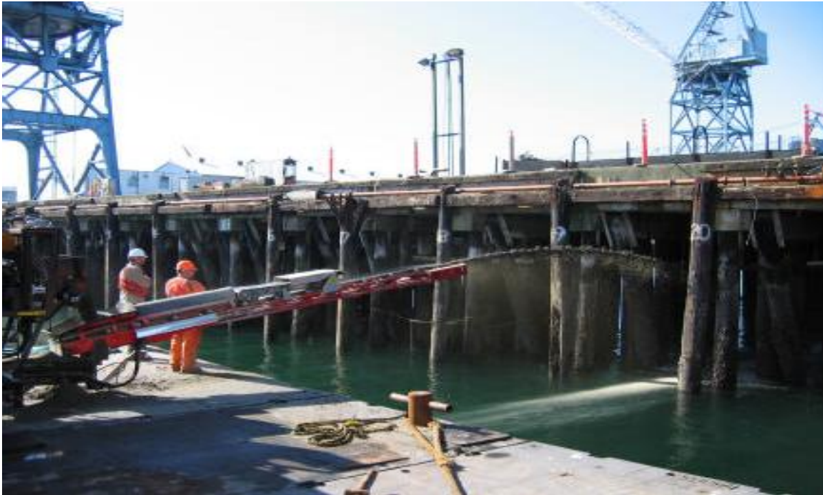
Figure 7-6 Placement of Under-pier Capping Sand between Bents by Sand Throwing Barge
