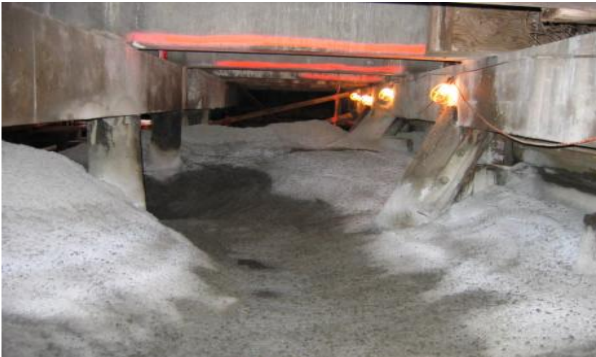
Figure 7-7 Finished Shotcrete Surface on Debris Mound
