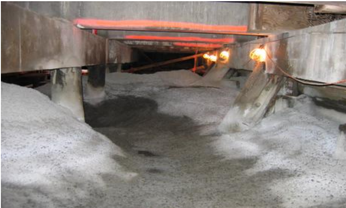
Figure 7-7 Finished Shotcrete Surface on Debris Mound
