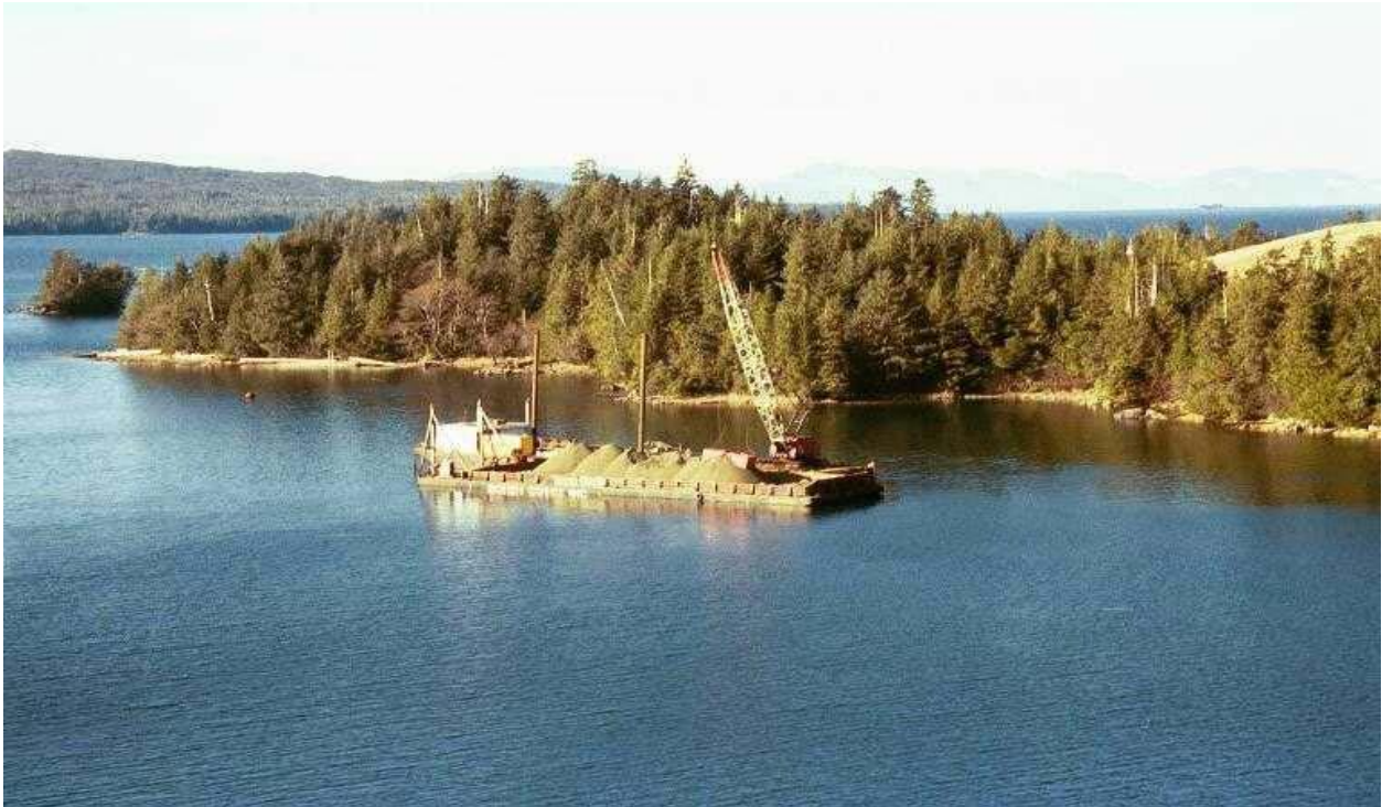
Figure 7-3 Mechanical Placement of Cap at Ward Cove, Alaska
