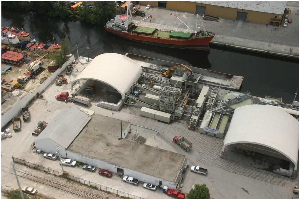
Soil Washing, Miami River Soil/Sediment Separation Plant. Source: Boskalis-Dolman 2006
