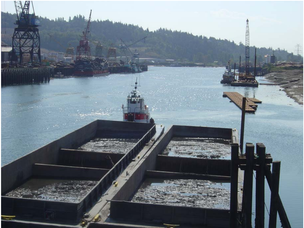
FIGURE 9-2 PASSIVE DEWATERING OF DREDGED SEDIMENTS IN BARGES ON THE HYLEBOS WATERWAY
