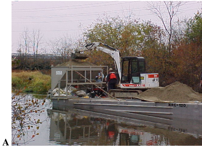
FIGURE 7-8 DRY CAP PLACEMENT AT THE PINE STREET CANAL DEMONSTRATION PROJECT, VERMONT
