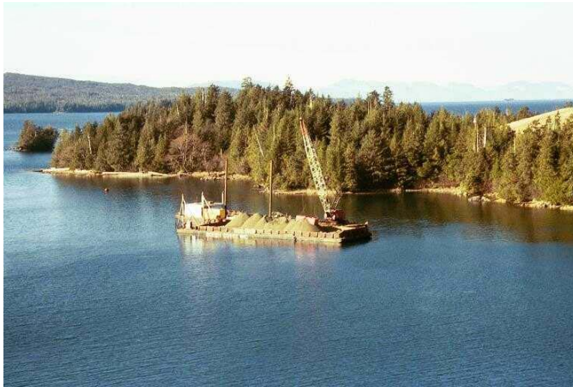
FIGURE 7-9 MECHANICAL PLACEMENT AT WARD COVE, ALASKA
