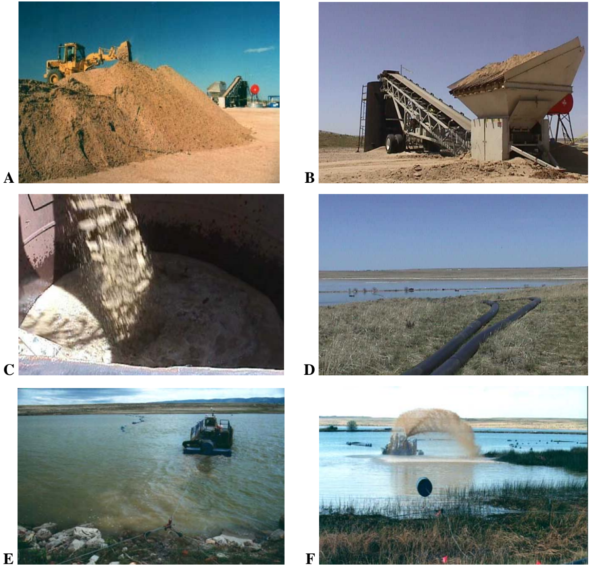
FIGURE 7-6 HYDRAULIC PLACEMENT AT SODA LAKE, WYOMING
