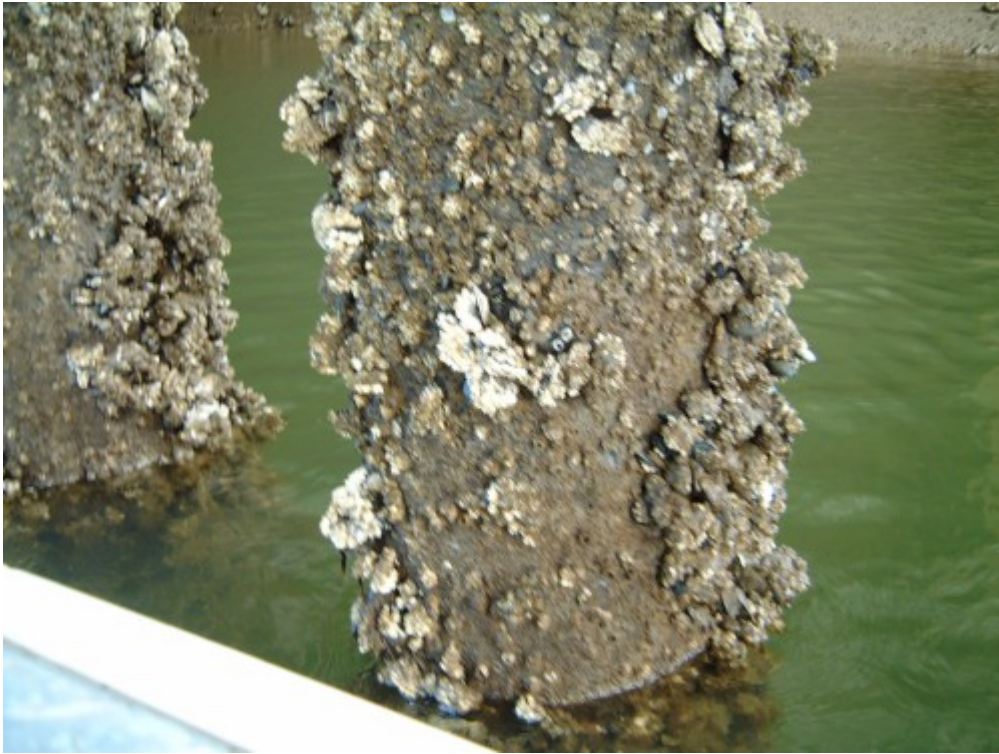
Photo 3. Mussels on pilings of the 16 th Avenue Bridge (RM 3.3). Photo taken during initial reconnaissance survey, July 16, 2003.
