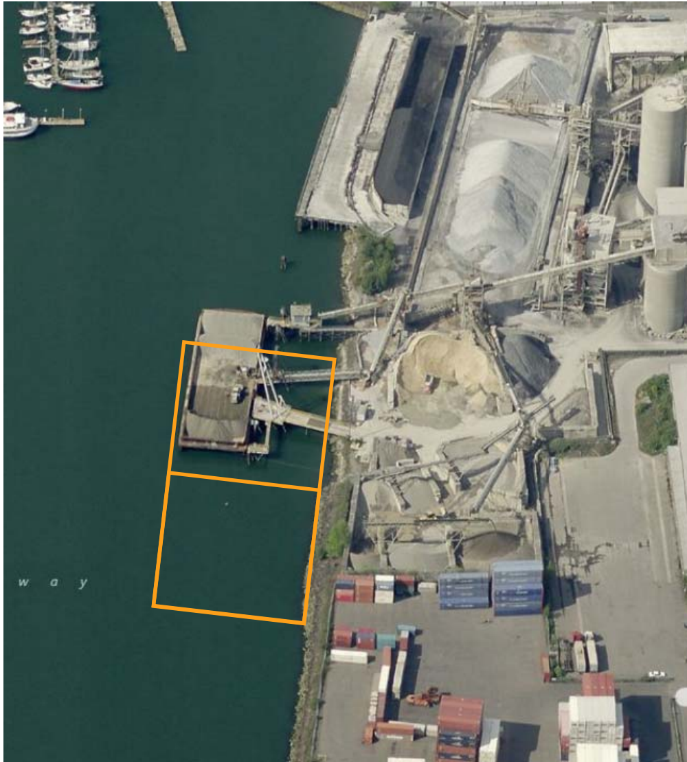
Area 2 - Scour Mitigation
