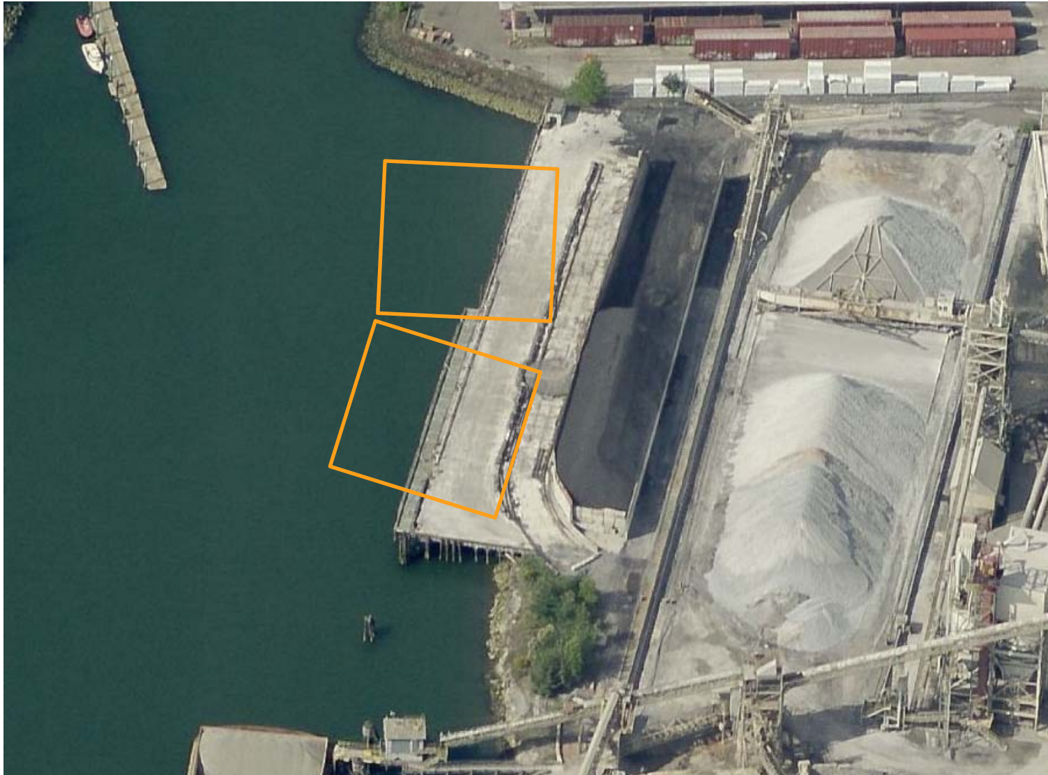
Area 1 –Scour Mitigation
