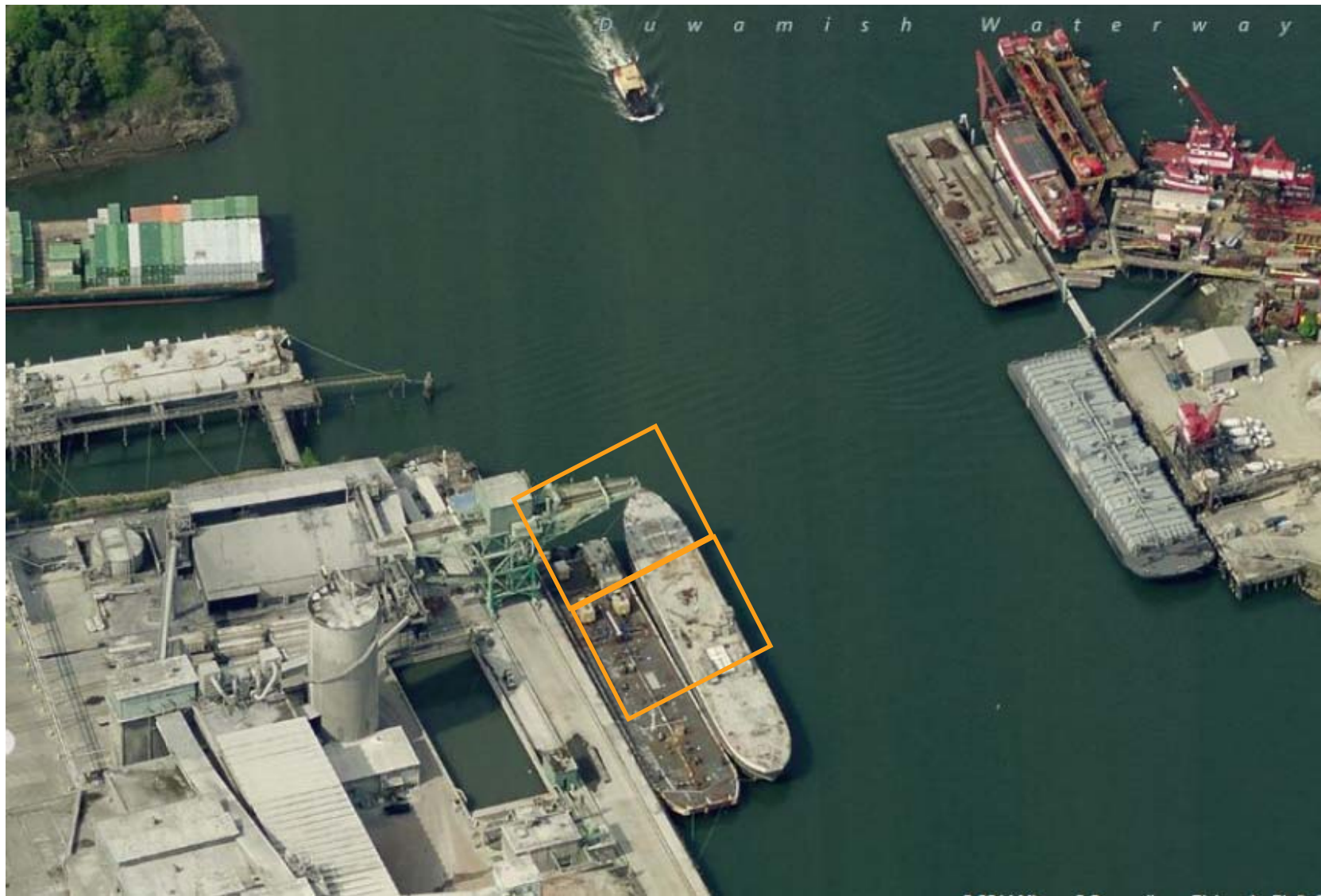
Area 7 –Scour Mitigation
